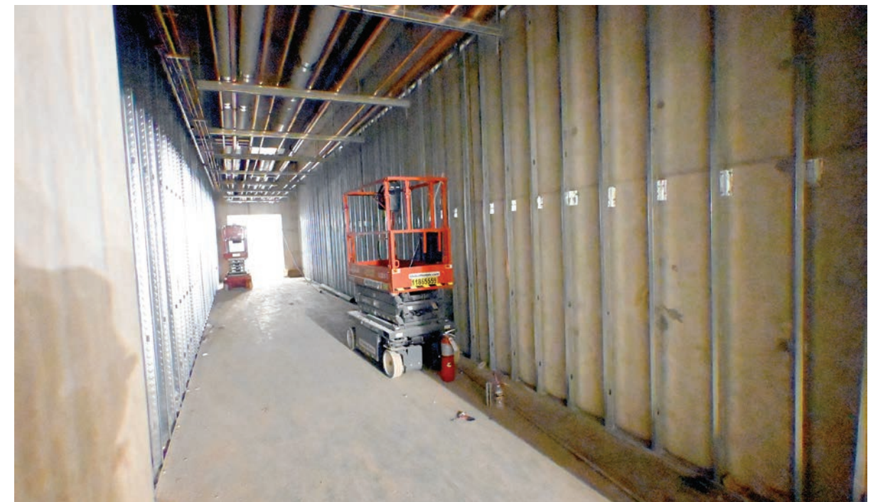
Overhead mechanical piping has been installed in the basement.
