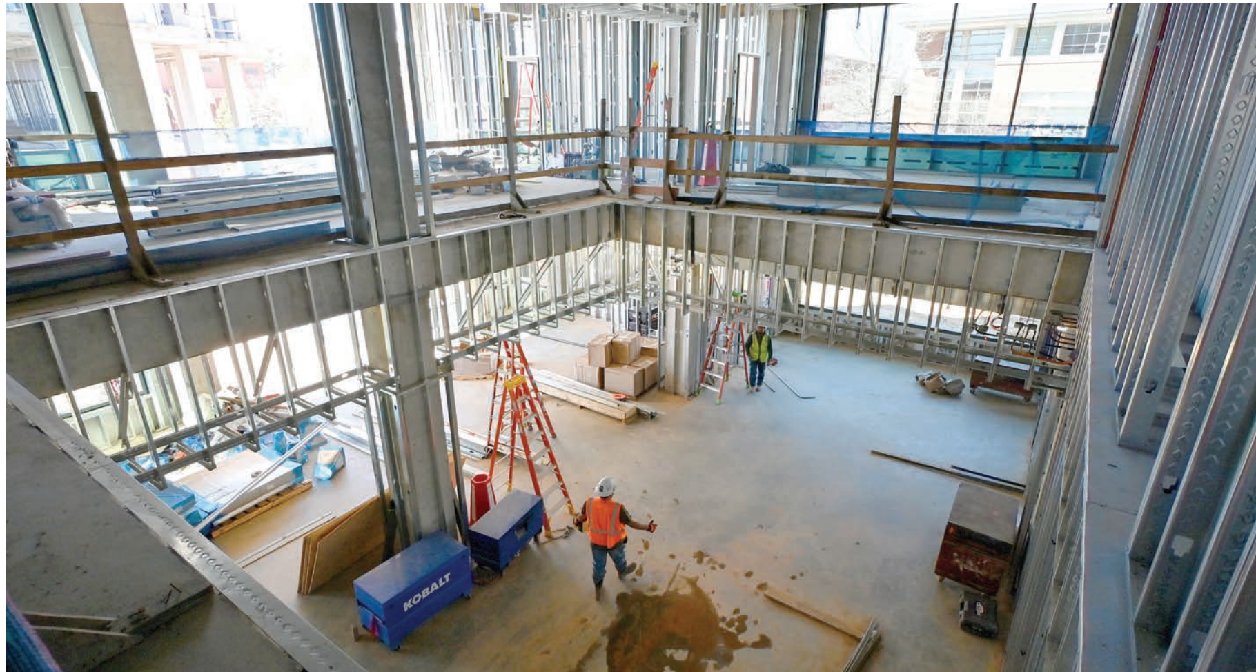
Metal framing is being installed around the lobby area.
