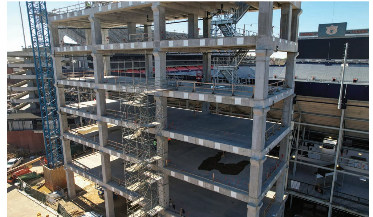
The steel stairway has been installed. Mechanical, electrical and plumbing lines are being added.
