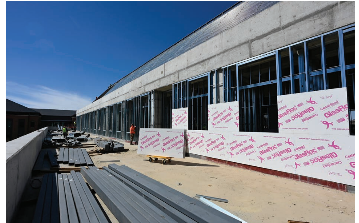
The mechanical penthouse is being enclosed, as viewed from the rooftop terrace.
