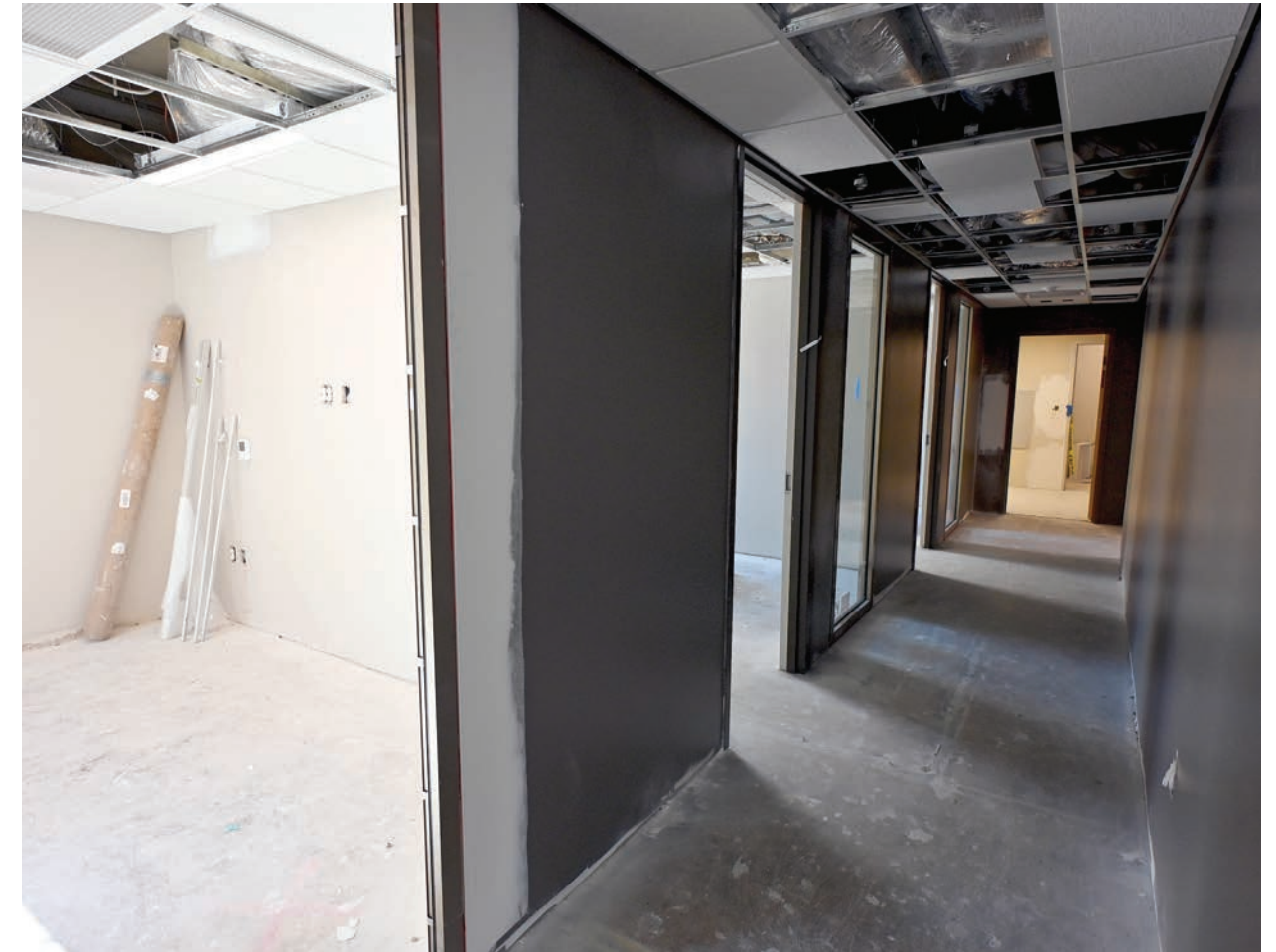
Offices have been painted and are awaiting installation of windows and doors.
