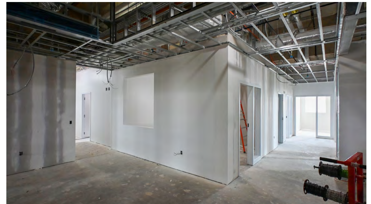
Ceiling grid installation continues on the third floor.
