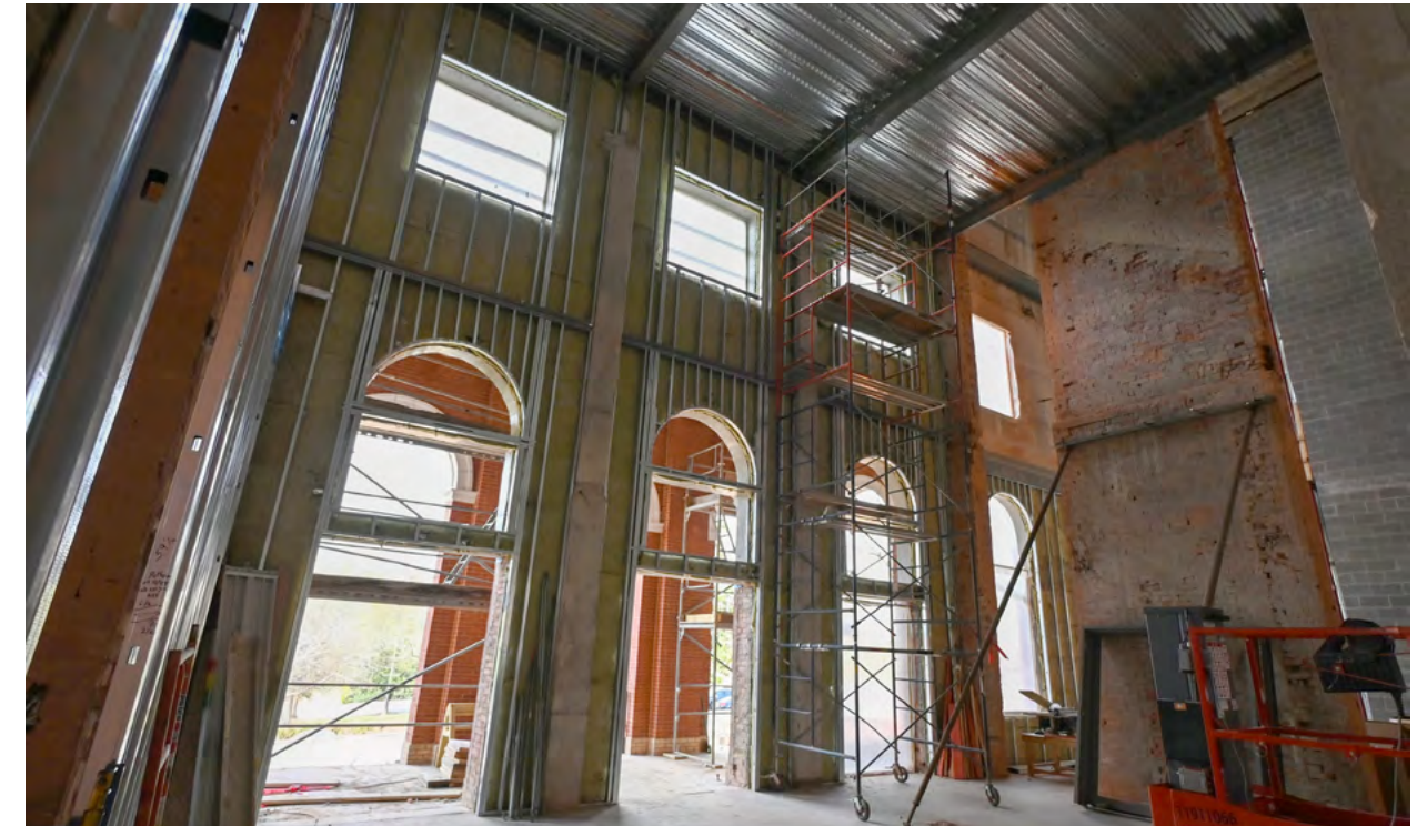
The new first-floor entry atrium.
