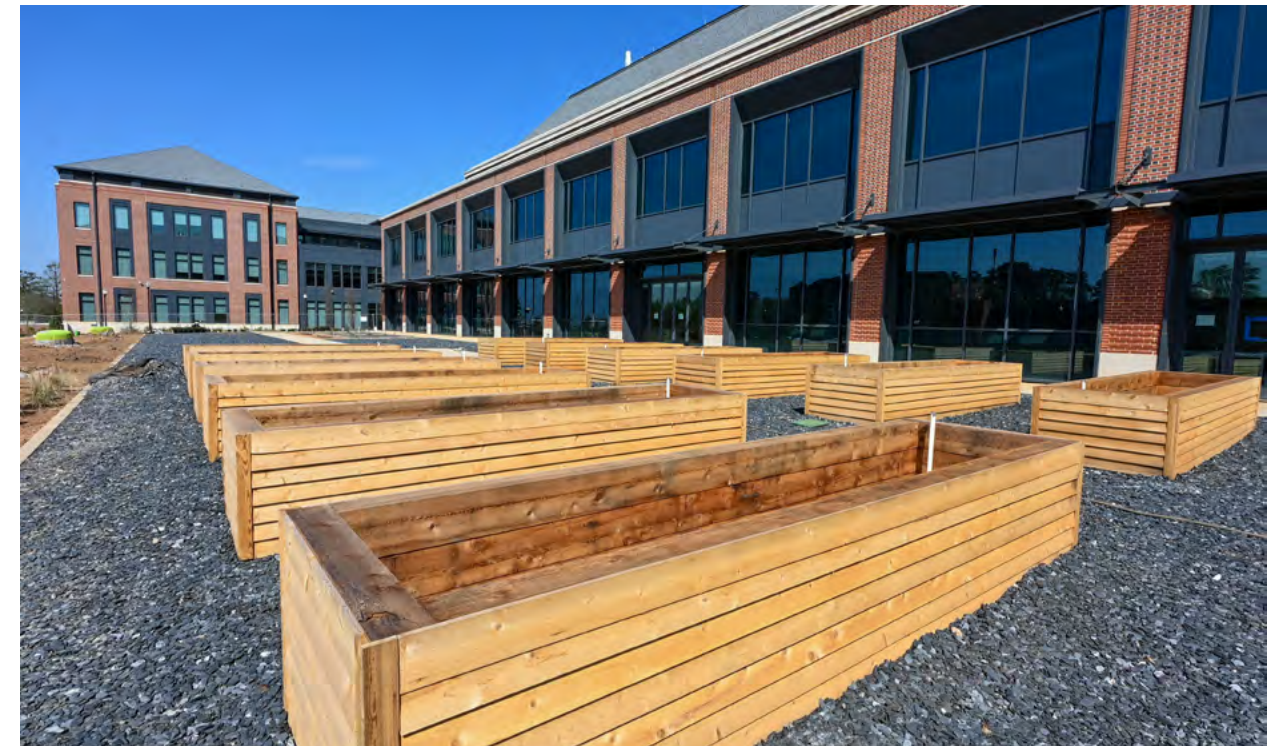
Construction of the raised bed planters is complete in the teaching garden.
