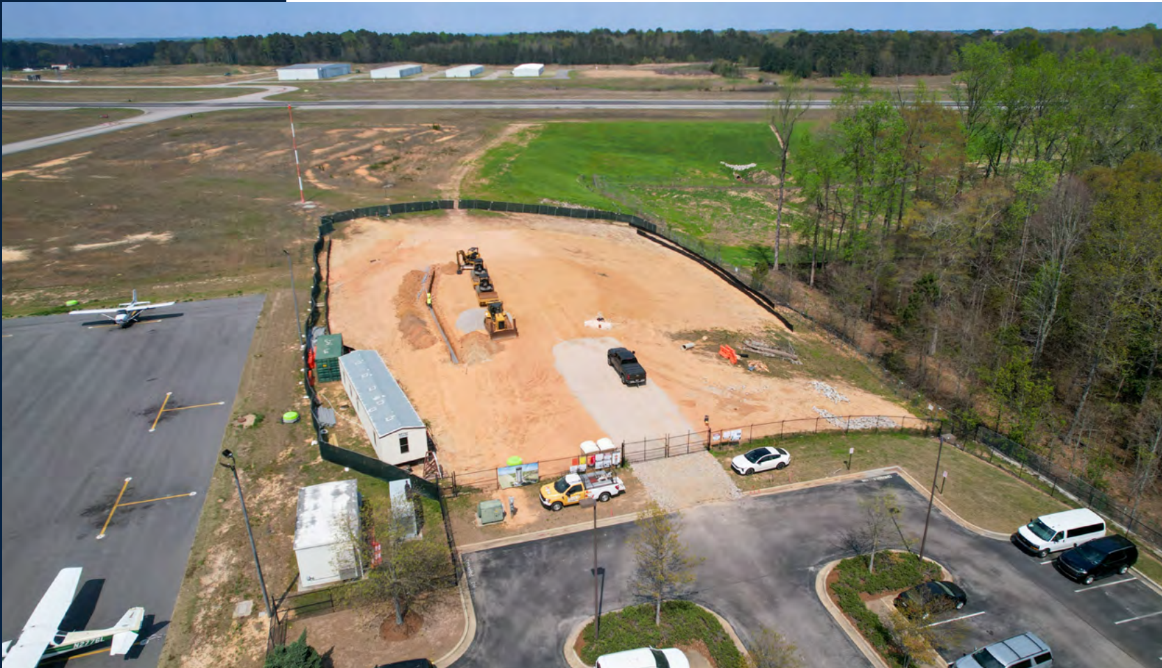
Utility and foundation work is underway at the future air traffic control tower site.
