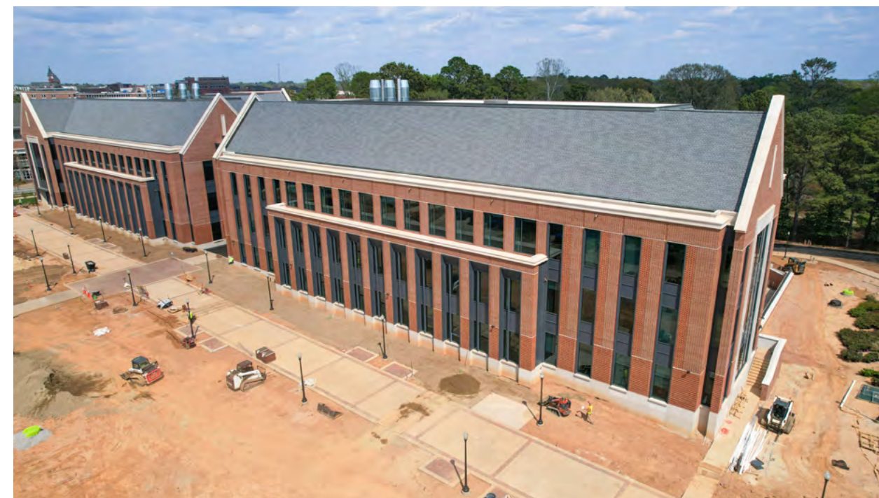
Lighting and landscape installation is taking place beside Building C.
