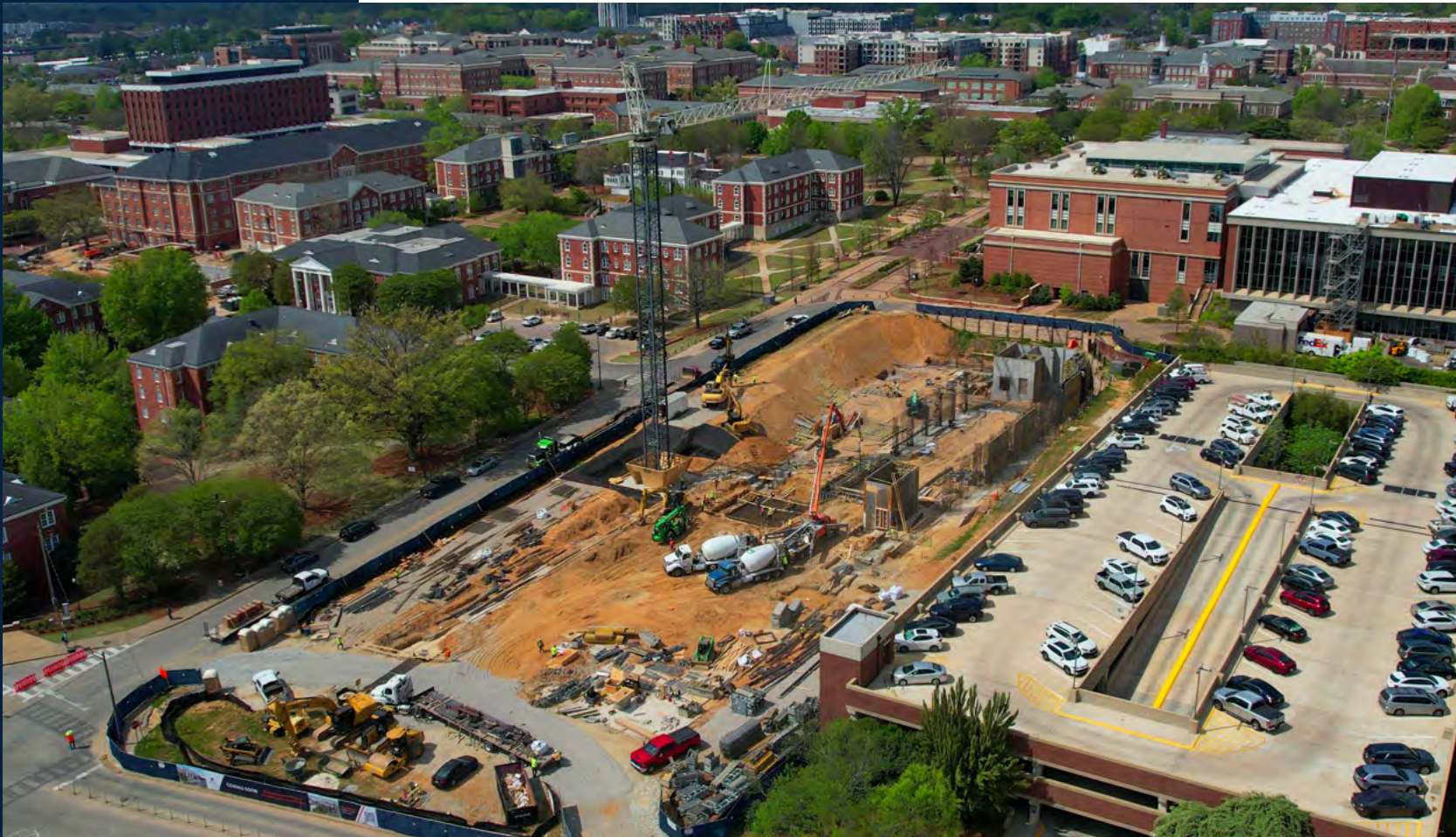
Reinforcement and framework is being erected for the elevator and stair tower.
