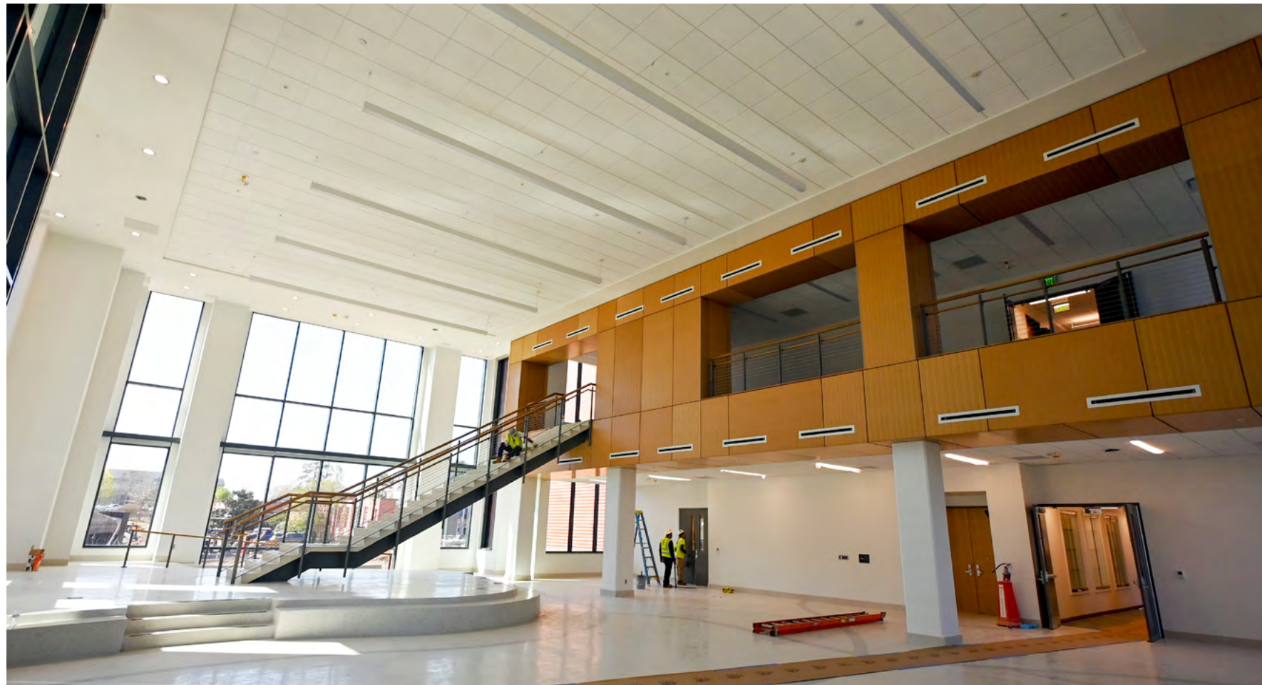
Installation of the flooring and wooden wall panels are complete in the lobby.
