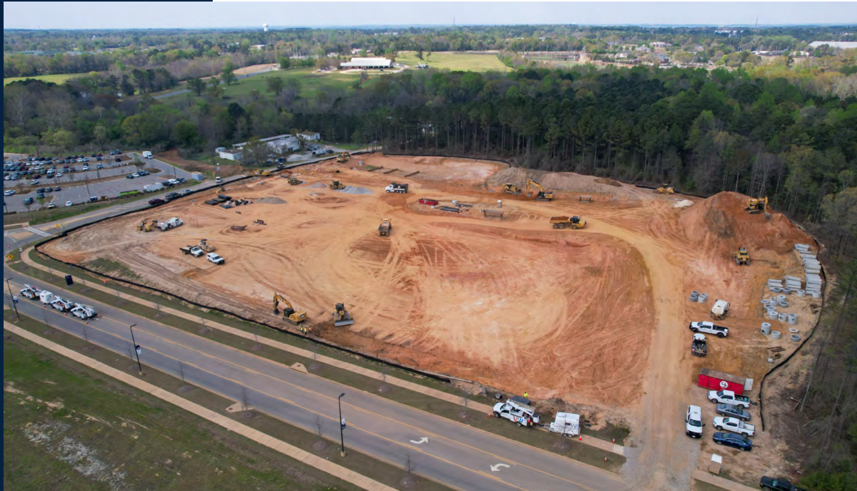
Site preparation is underway for the new building.
