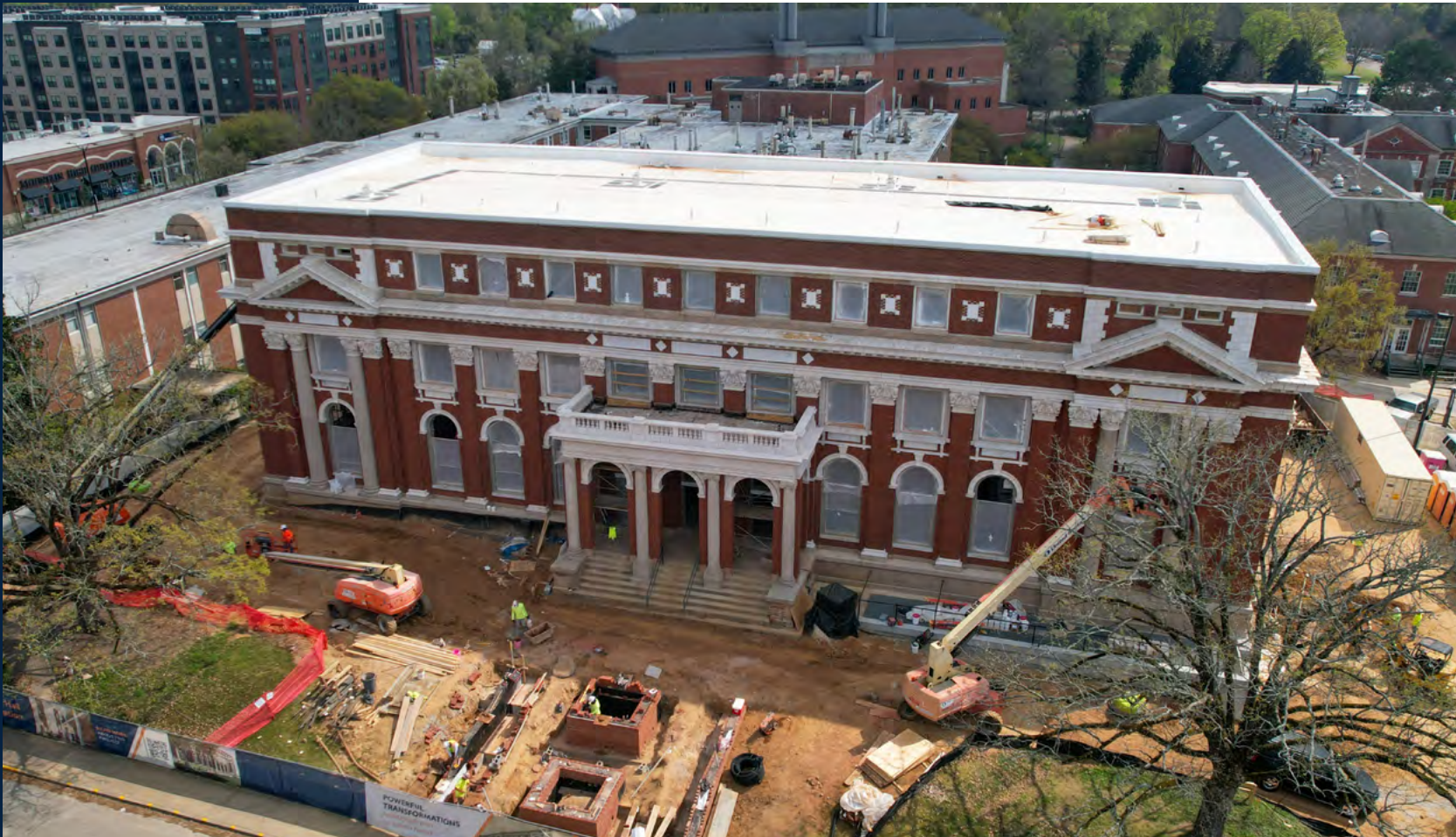
Exterior restoration and site work continue.
