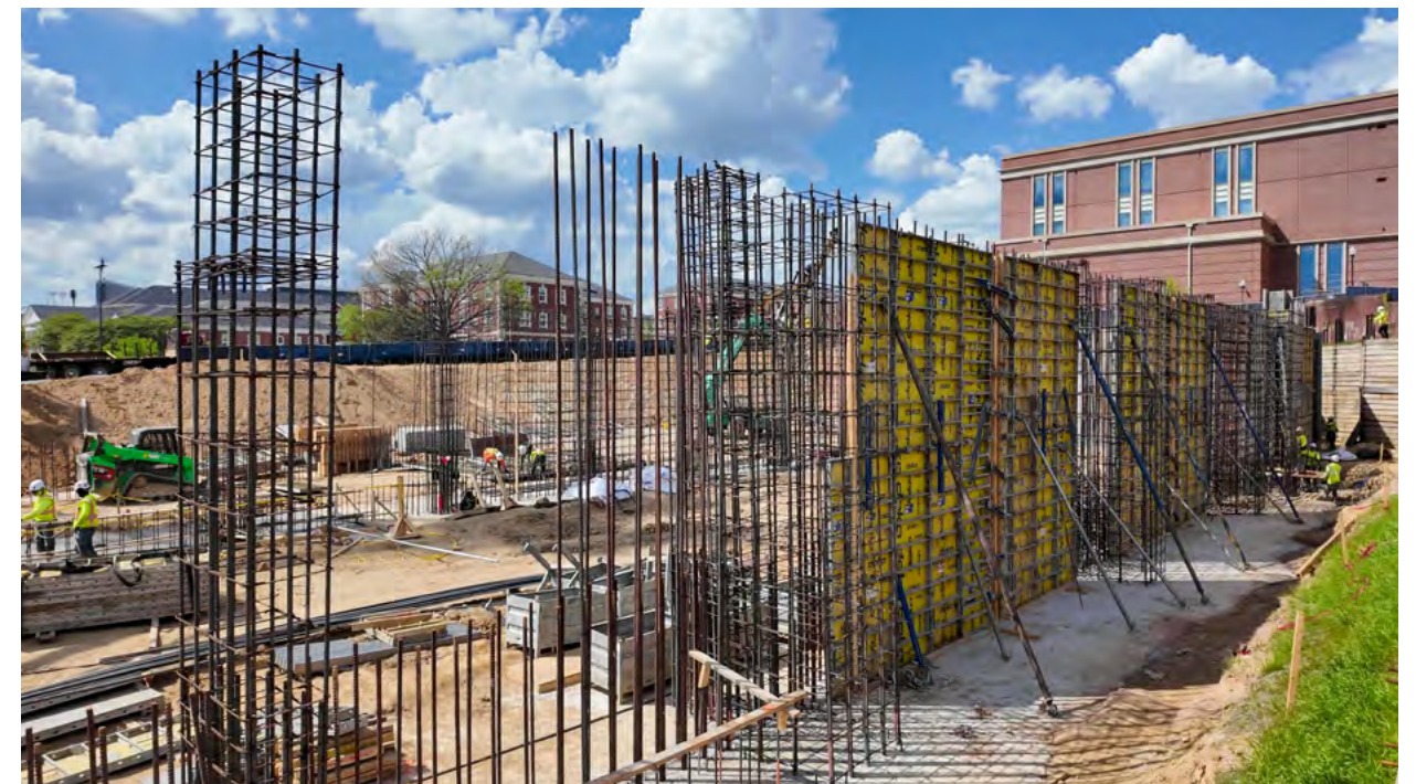
A section of the basement wall is being erected.
