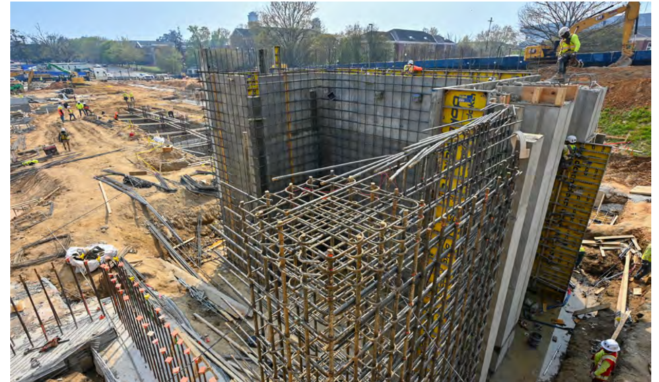
Reinforcement and framework is being erected for the elevator and stair tower.
