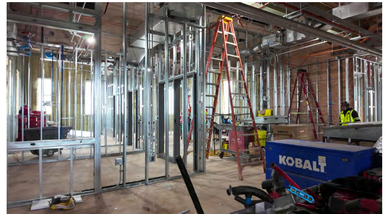
Interior wall framing is taking place on the second floor.
