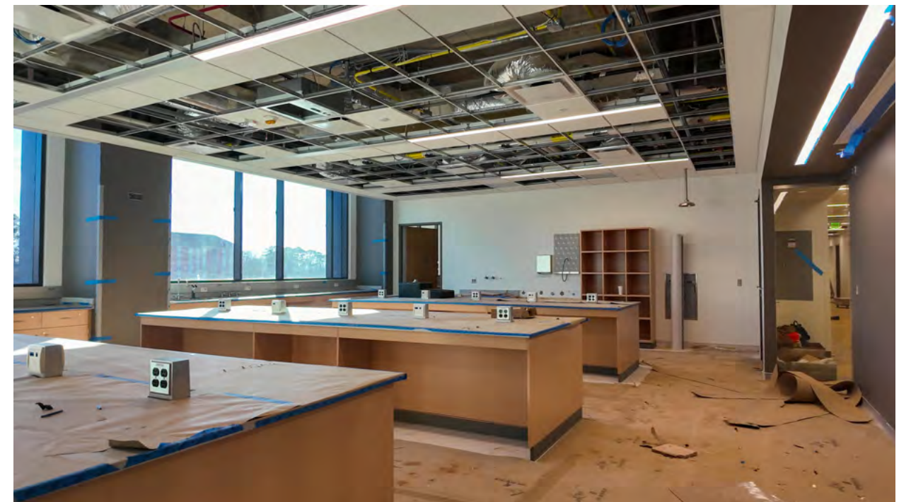
Casework installation is taking place in this teaching laboratory.
