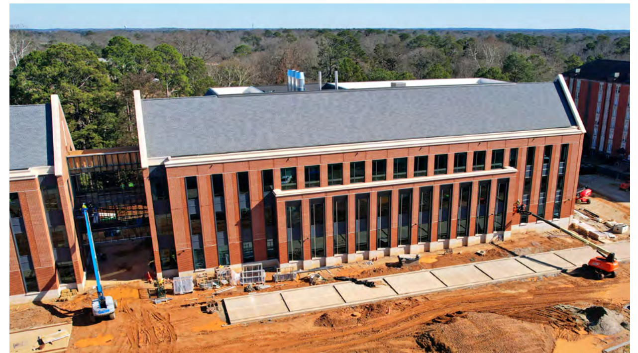
Curtain wall installation is in progress on the bridge between Buildings B and C.
