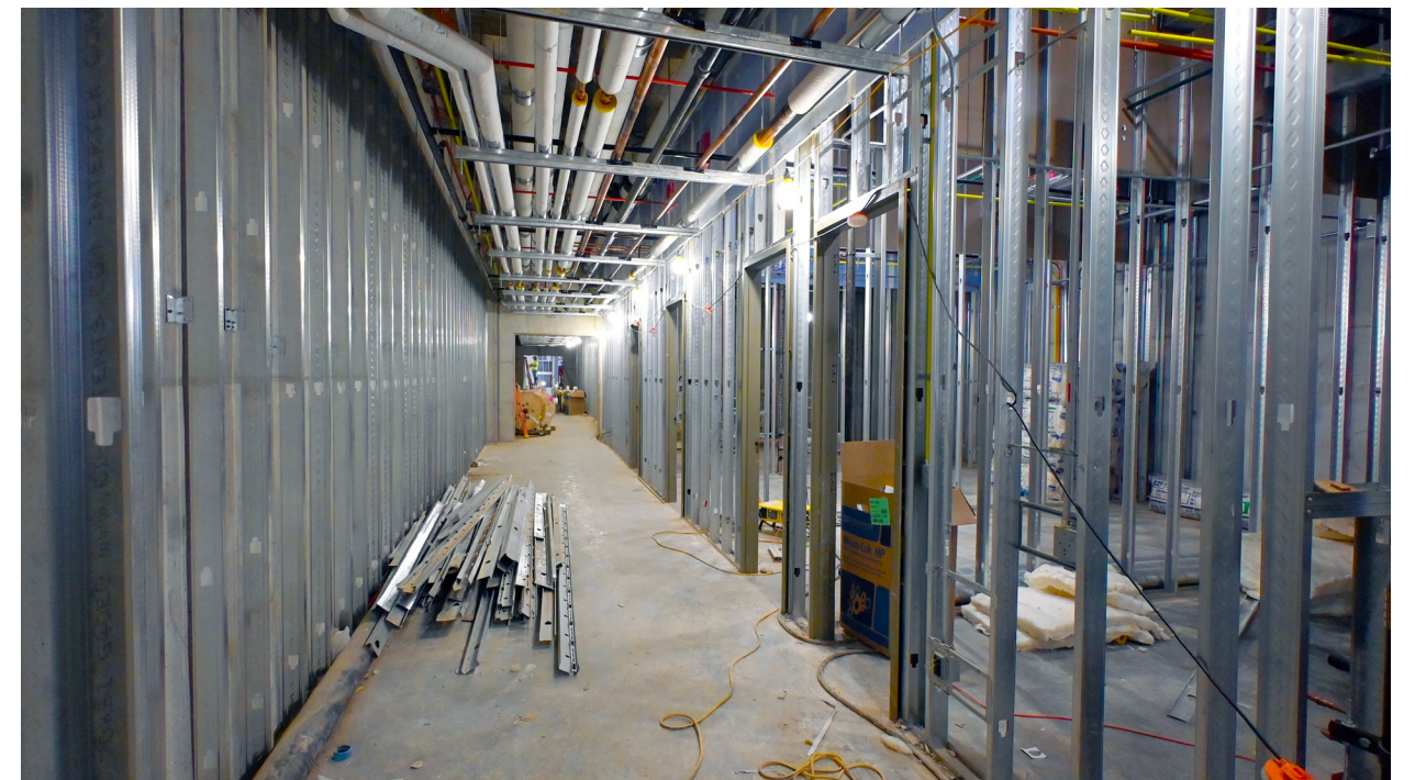
Metal wall framing is complete in this second floor hall.
