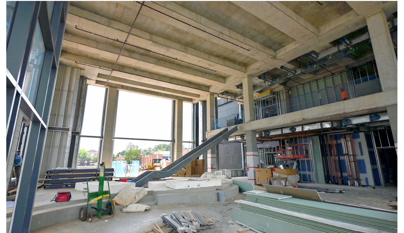
The main staircase is being installed in the atrium.
