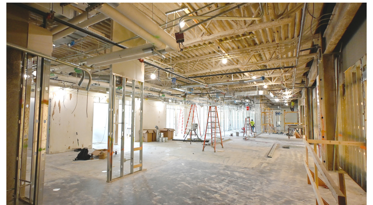
Above ceiling mechanical, electrical and plumbing systems are being installed for the new meeting and office spaces.
