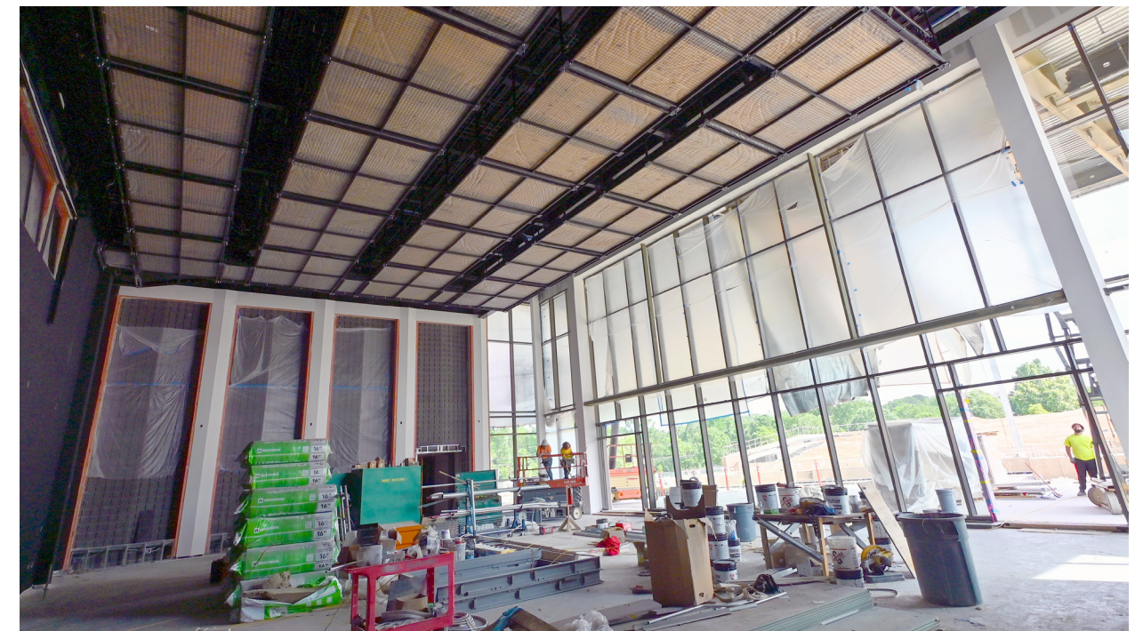
The glass curtain wall is complete. HVAC ductwork installation and drywall work are underway.
