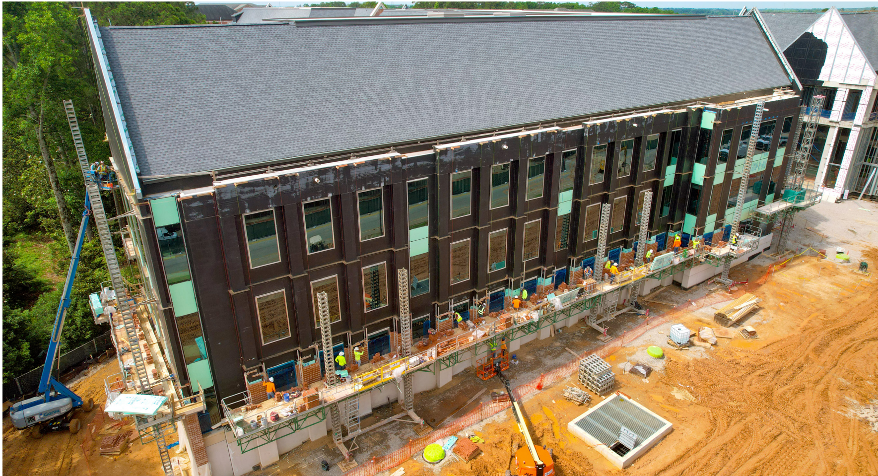
Brickwork is underway on the West Samford Avenue side of Building B.
