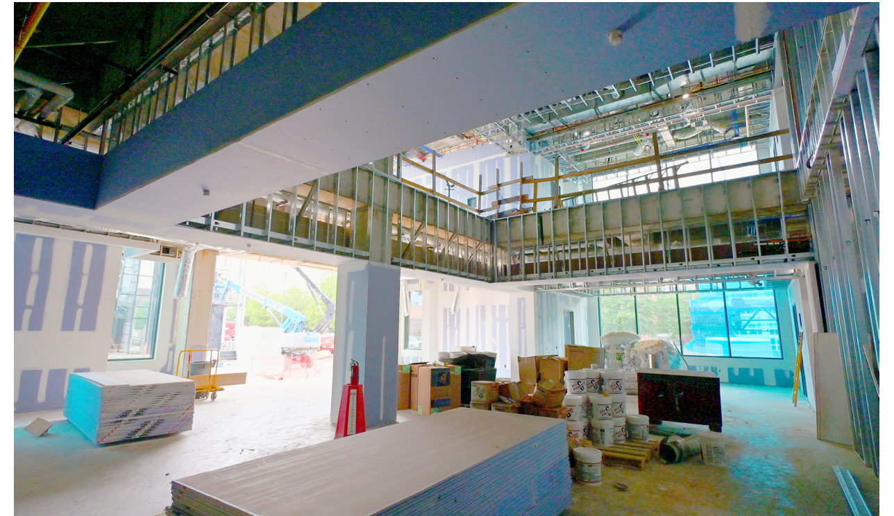
Drywall installation is underway in the atrium of Building B.
