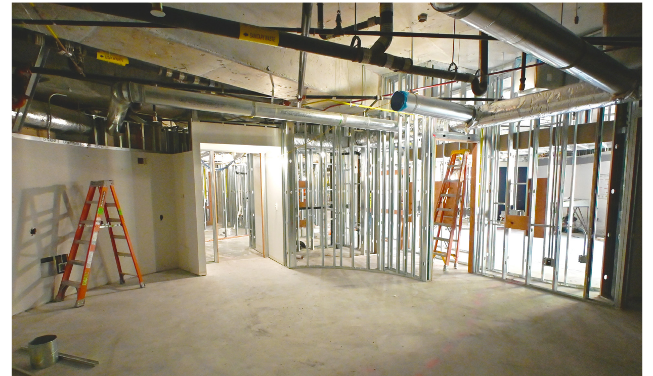
Metal wall framing and mechanical, electrical and plumbing systems in-wall assembly are ongoing.
