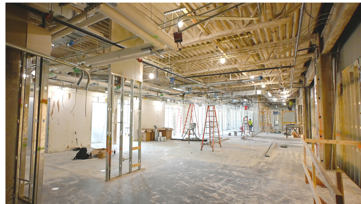
Above ceiling mechanical, electrical and plumbing systems are being installed for the new meeting and office spaces.
