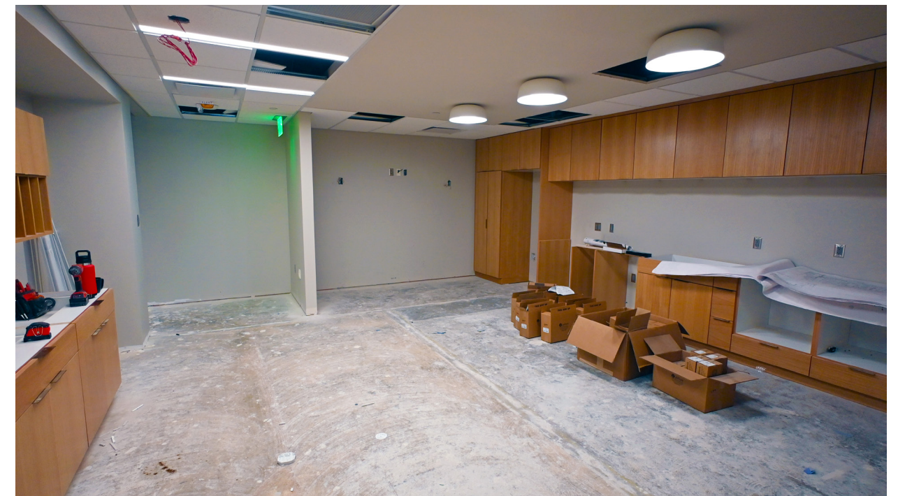
Cabinetry is being installed in the kitchenette.
