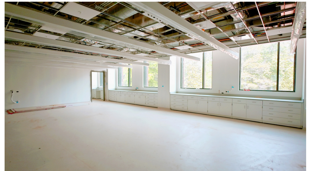
Installation of the cabinetry is underway in this laboratory.
