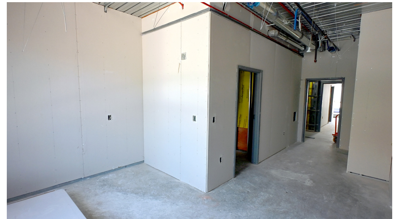
Drywall has been installed throughout the first floor.
