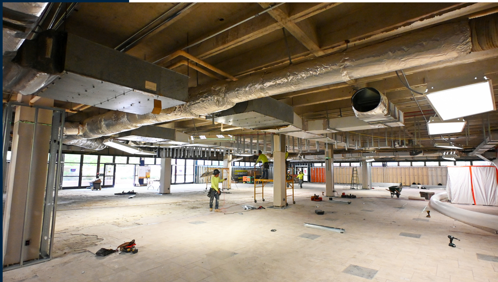
The campus bookstore in the Haley Center is undergoing selective demolition and reframing to transform its existing space.
