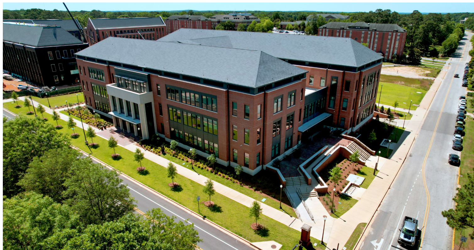
The College of Education building is complete. It features modern amenities and spaces designed to support collaborative learning and teaching innovation. Look in the occupied section of this document to read more.
