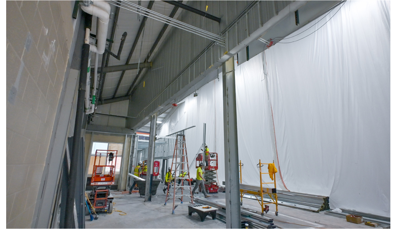
Drywall layout and framing have begun around the future offices for volleyball's assistant coaches, coordinator and director.
