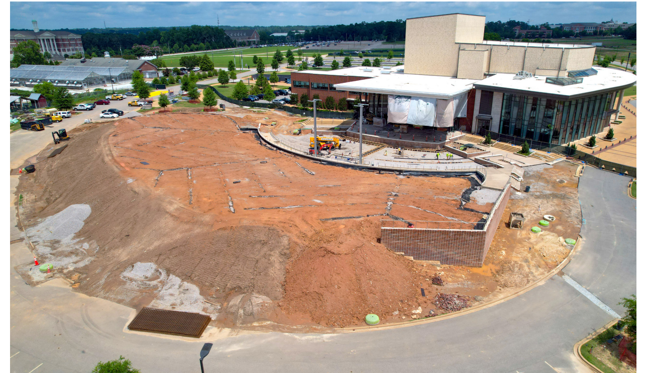
Site grading in the lawn area is complete and is ready for drainage installation, followed by topsoil and sod layers.
