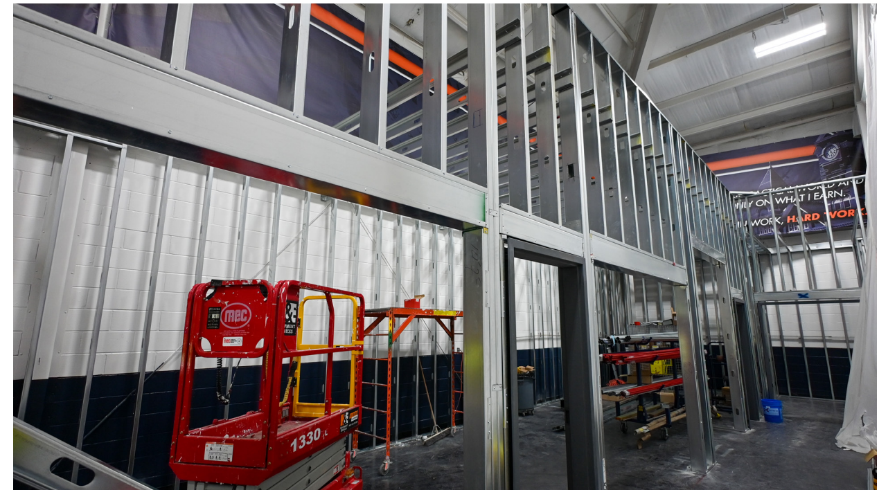
Framing is underway for the head coach's office.
