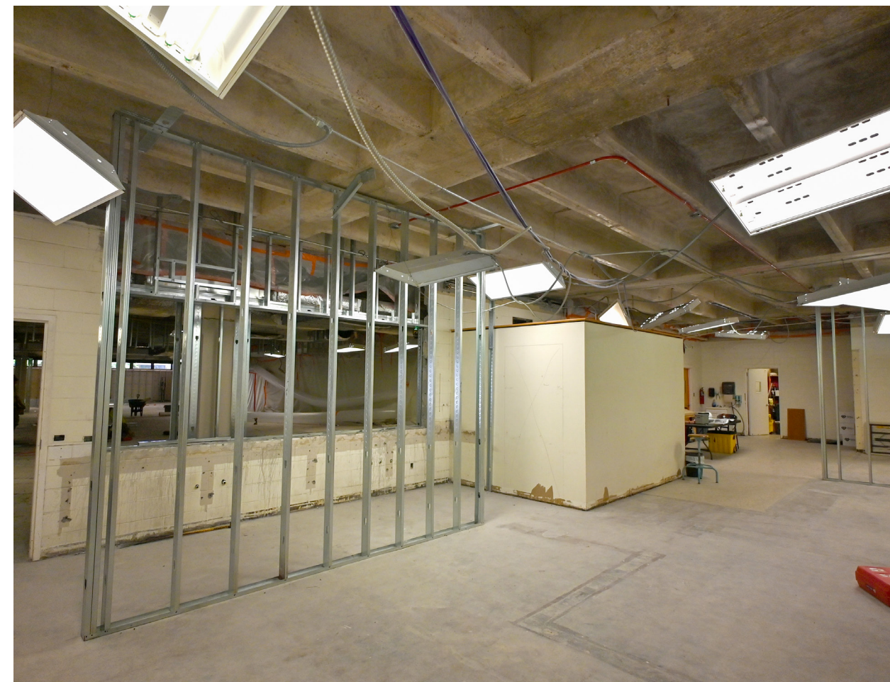
Metal framing is underway near the new book storage area.
