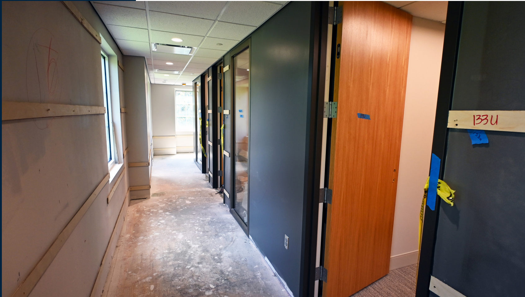
The walls in this hallway are being prepared for wood paneling.
