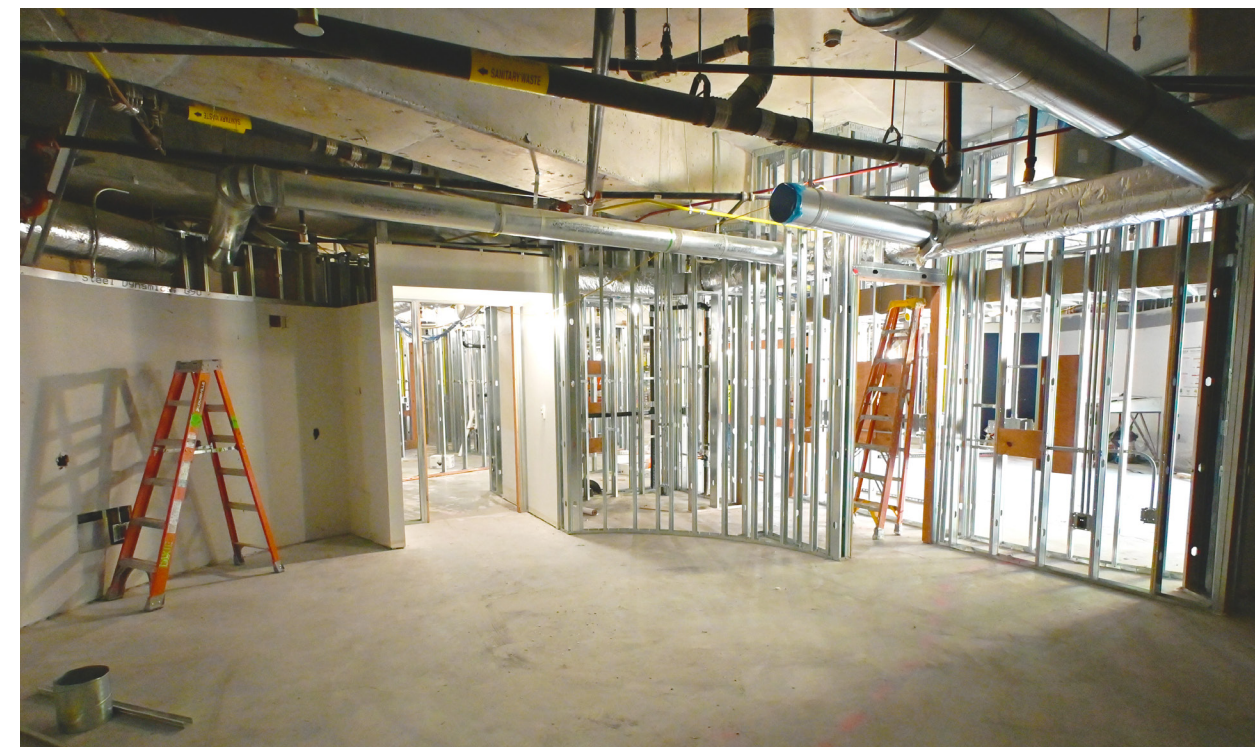
Metal wall framing and mechanical, electrical and plumbing systems in-wall assembly are ongoing.
