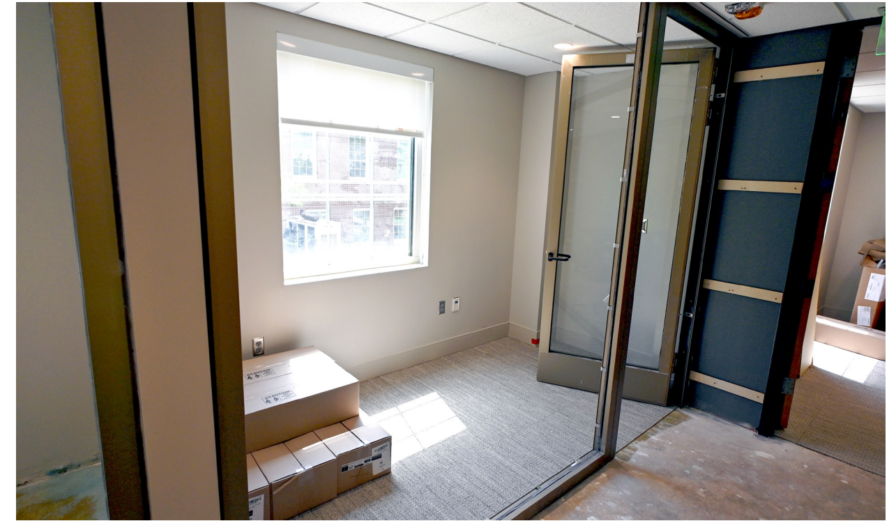
Flooring installation is underway in this meeting area.
