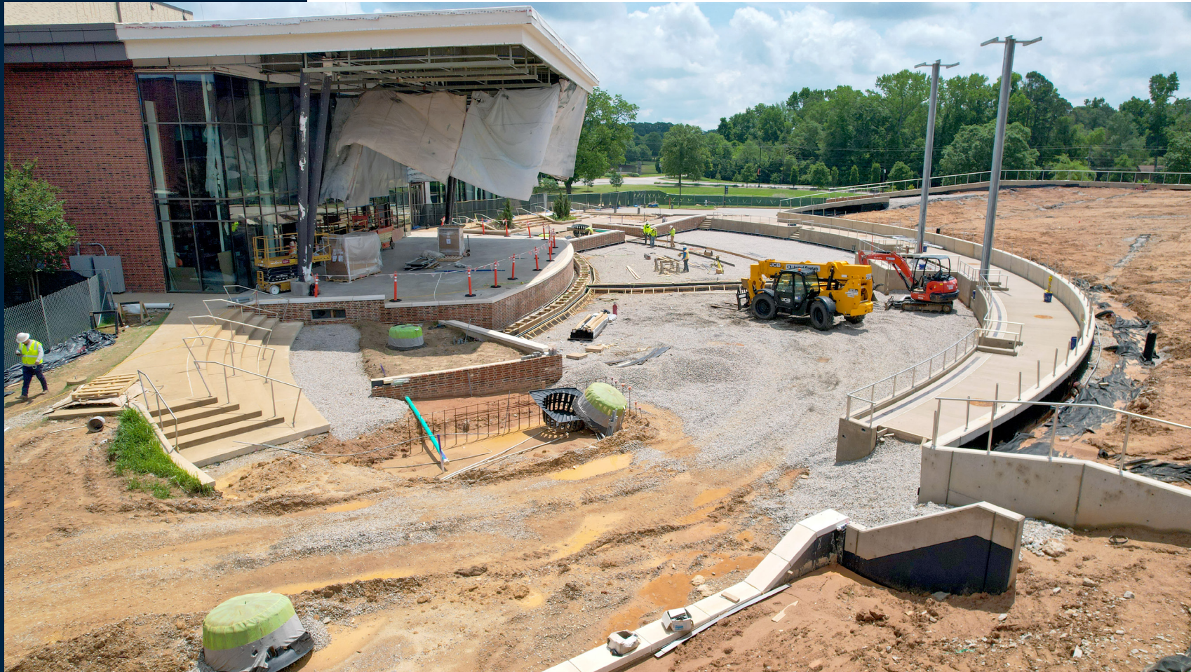
The orchestra area is being prepared for concrete placement.
