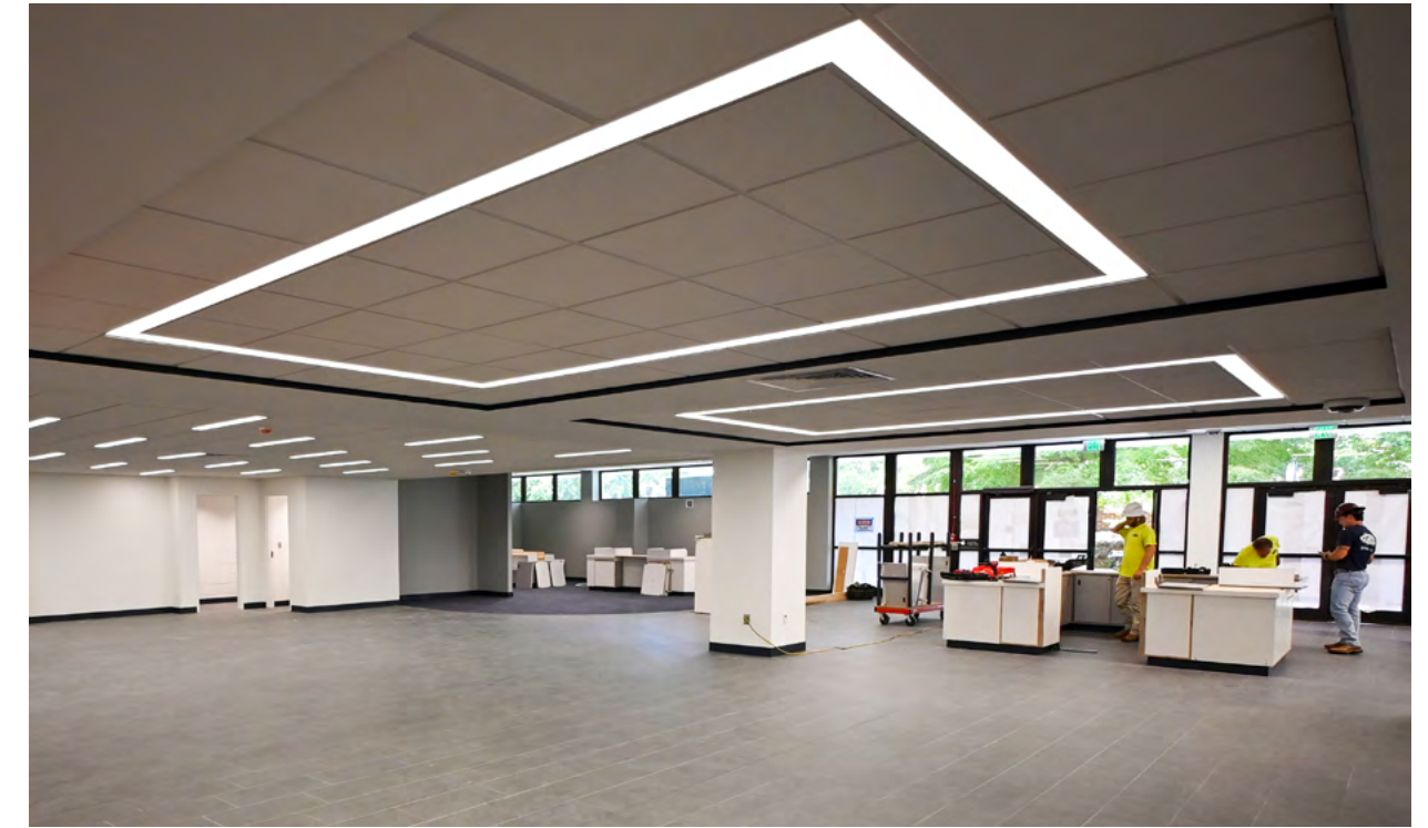
The main retail sales floor includes new recessed LED lighting to replace the previous fluorescent lighting.
