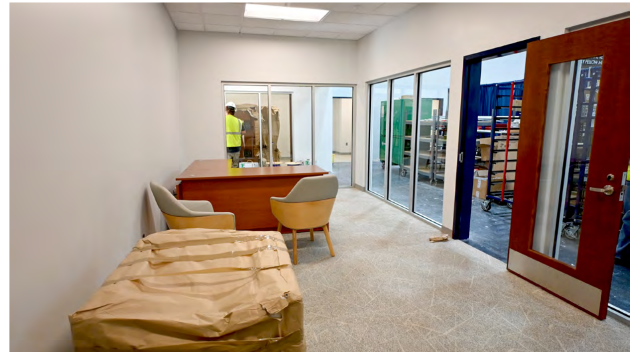
Furniture is being placed in this office.
