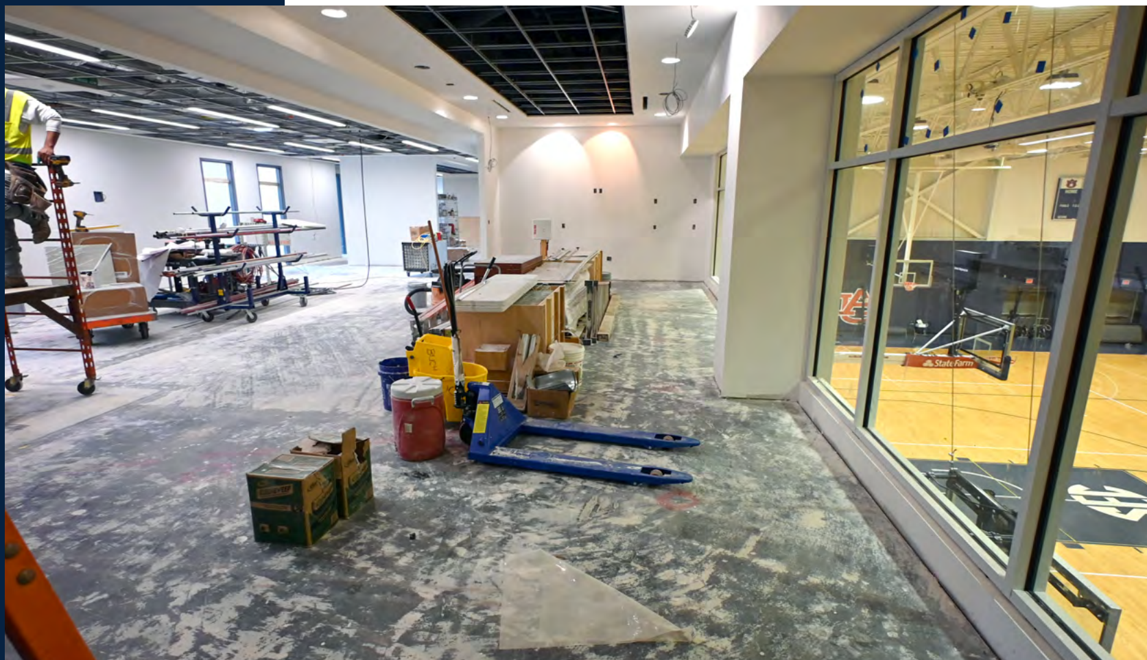
The reception and lounge areas for men's basketball's administration renovation overlooks the practice gym.
