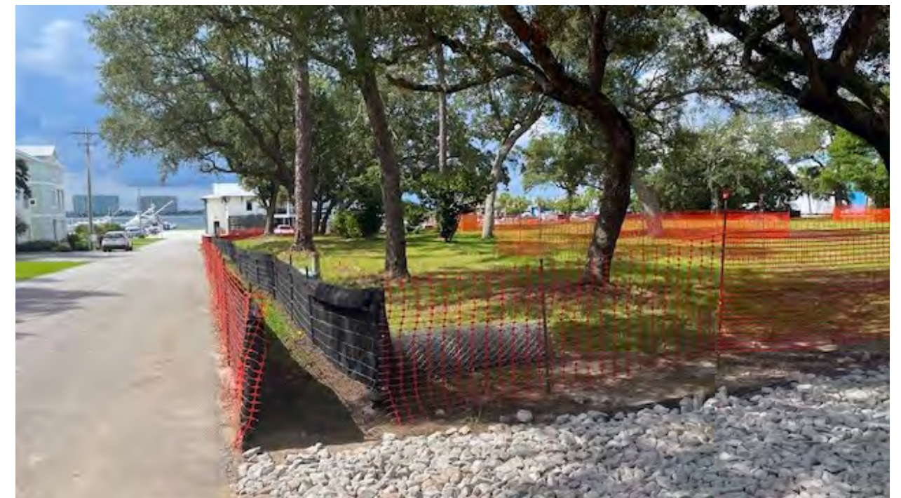
Construction fence installation recently began.
