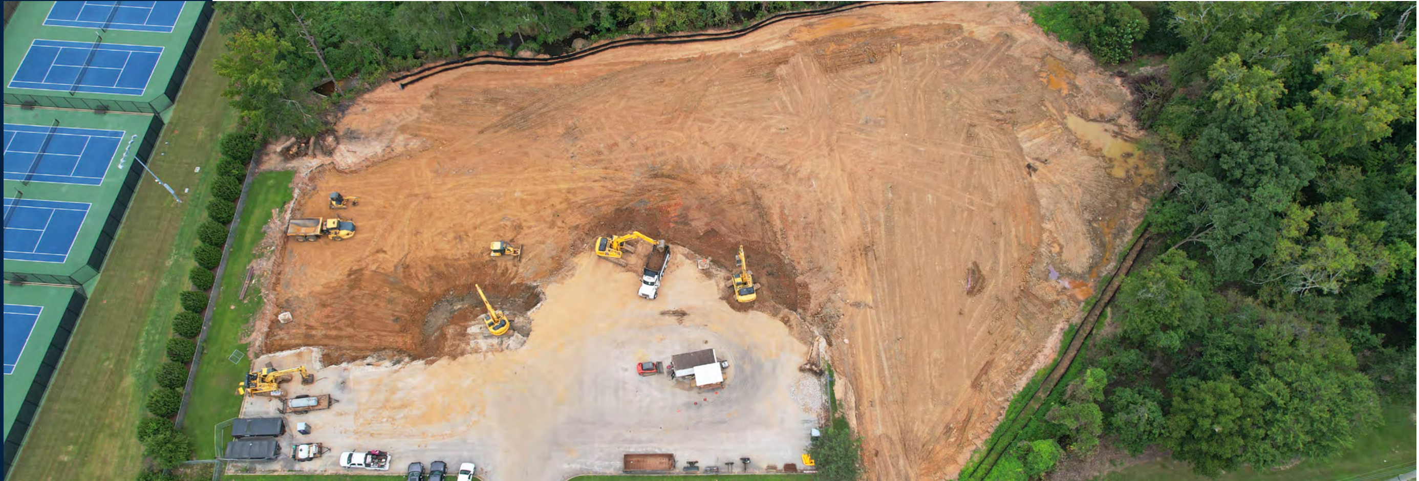
Soil is being removed from a former landfill on Hemlock Drive in preparation for future campus development.
