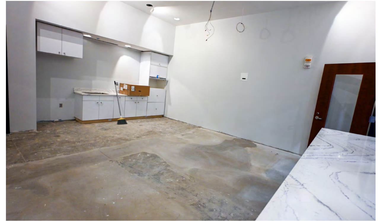
Cabinetry has been installed in the kitchen, with flooring installation scheduled as the next phase.
