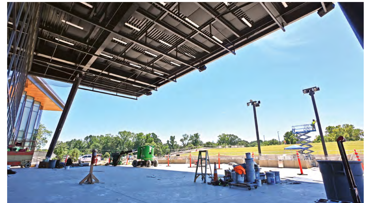
The stage will be complete once the bird netting is installed and the canopy supports are painted.
