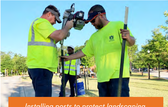
Installing posts to protect landscaping.
