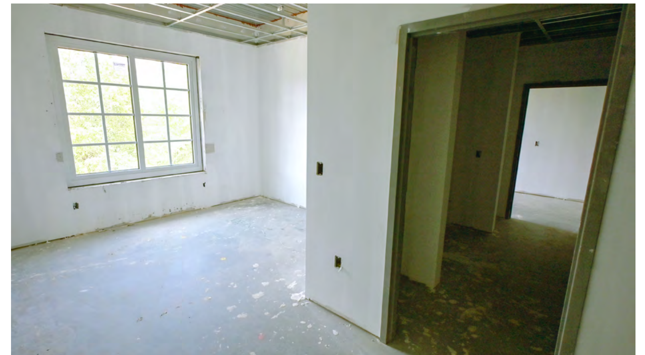
Window installation and the application of the first coat of paint are currently underway in this suite.
