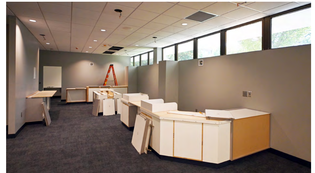
Cabinetry is being installed in the technology and computer repair area.
