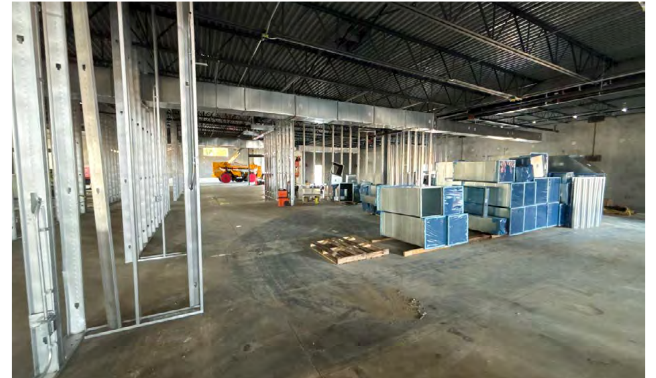
Layout and installation of interior framing, alongside mechanical systems installation.
