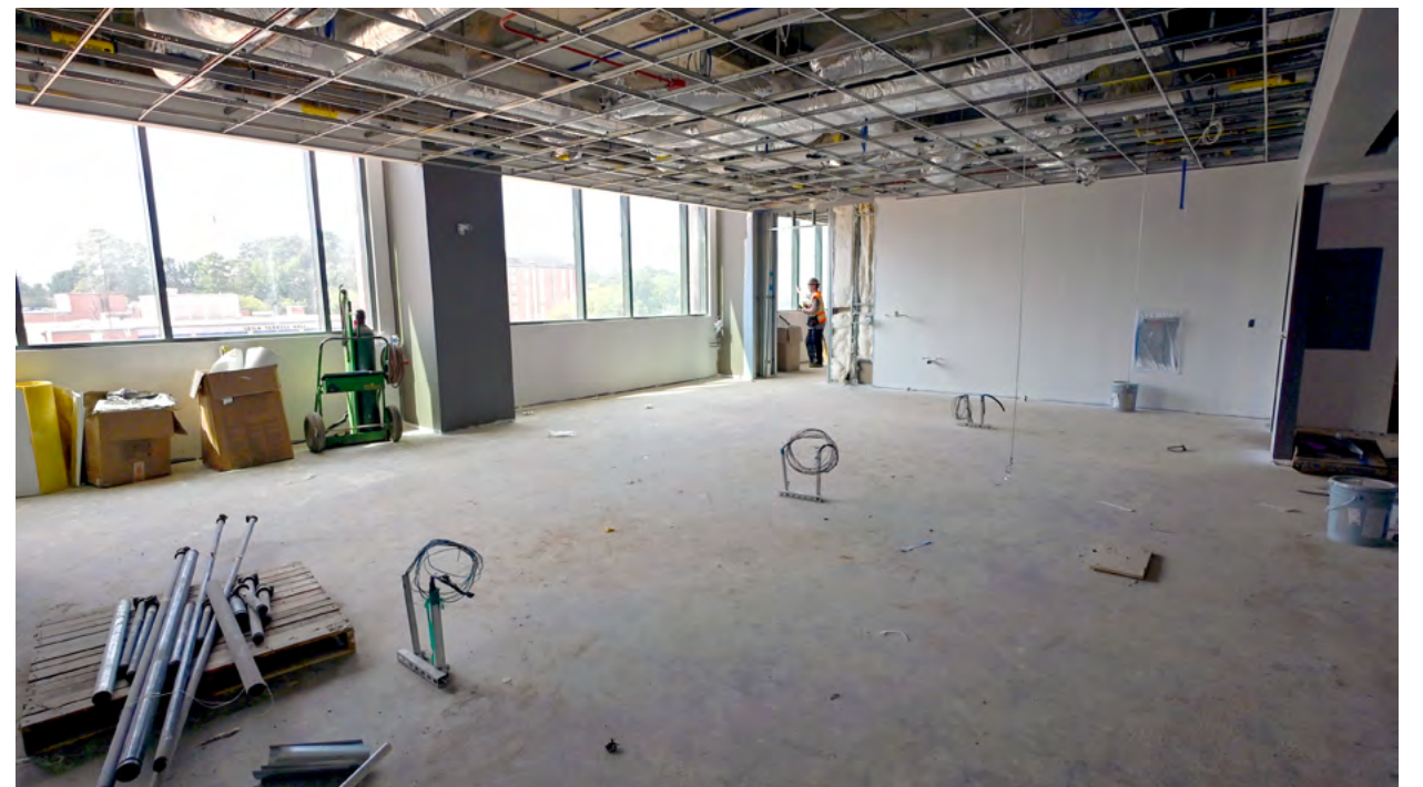
The teaching lab on the second floor of Building A is progressing with electrical and mechanical connections being installed.
