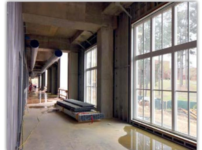
*Windows have been installed along the first floor hallway.*
