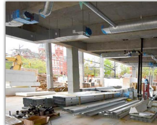
*Overhead mechanical duct work is being installed in the future 1856 Restaurant and Dining Room.*
