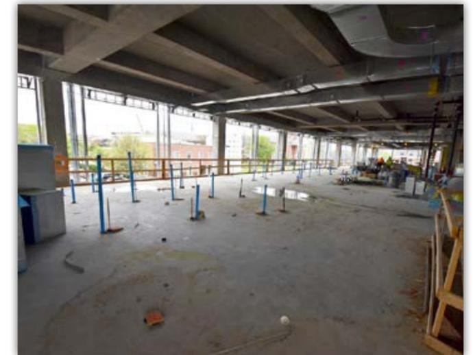
*Plumbing lines in the floor are being installed for the distilled spirits and wine appreciation labs.*
