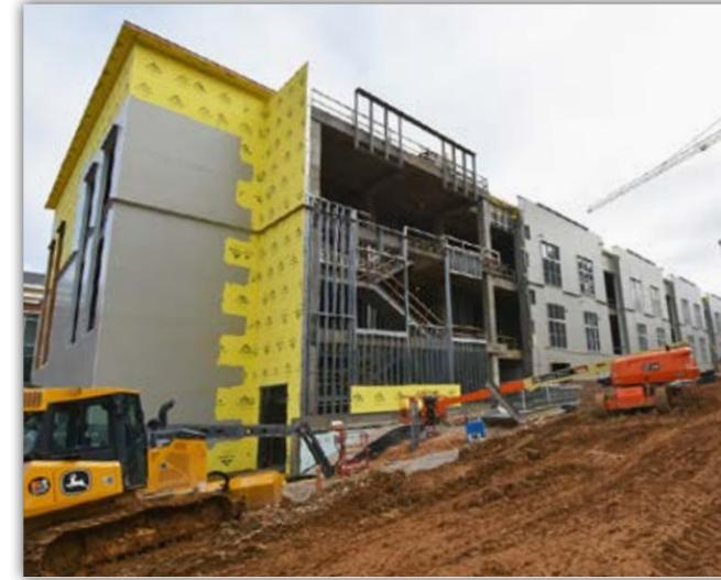
*Waterproofing is nearing completion on the south side of the ACLC.*
