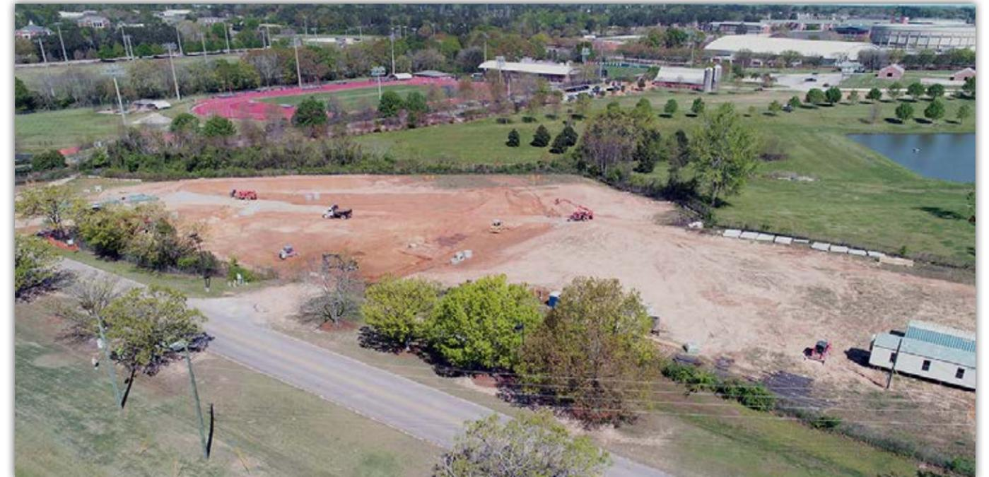
*Site work is underway, which includes underground electrical work and building foundation installations.*
