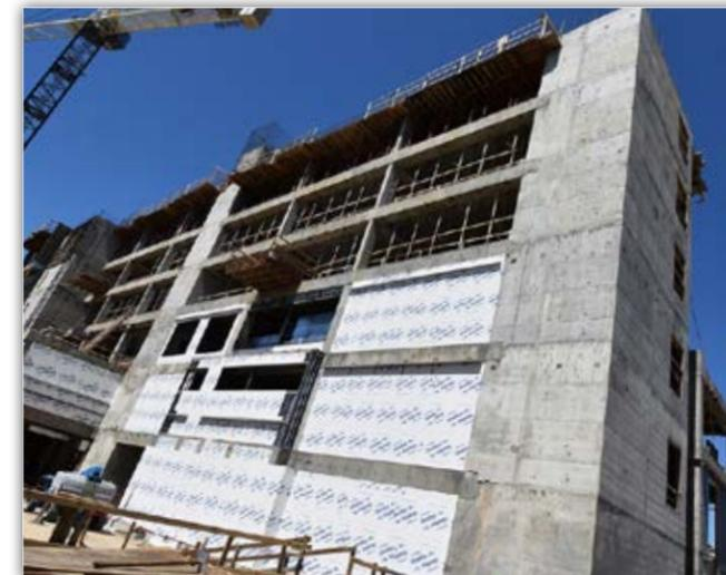
*Exterior barriers for the lower three floors are ongoing. Brick installation will begin in May.*
