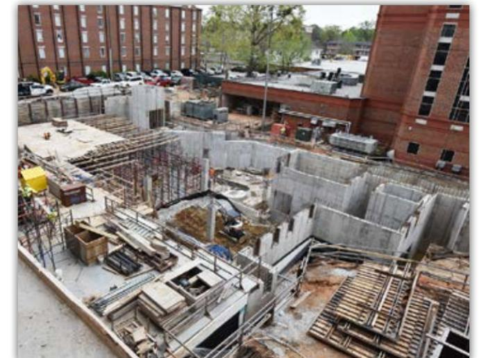
*Concrete formwork is ongoing at the underground loading dock along with preparations for the future food hall concrete slab.*
