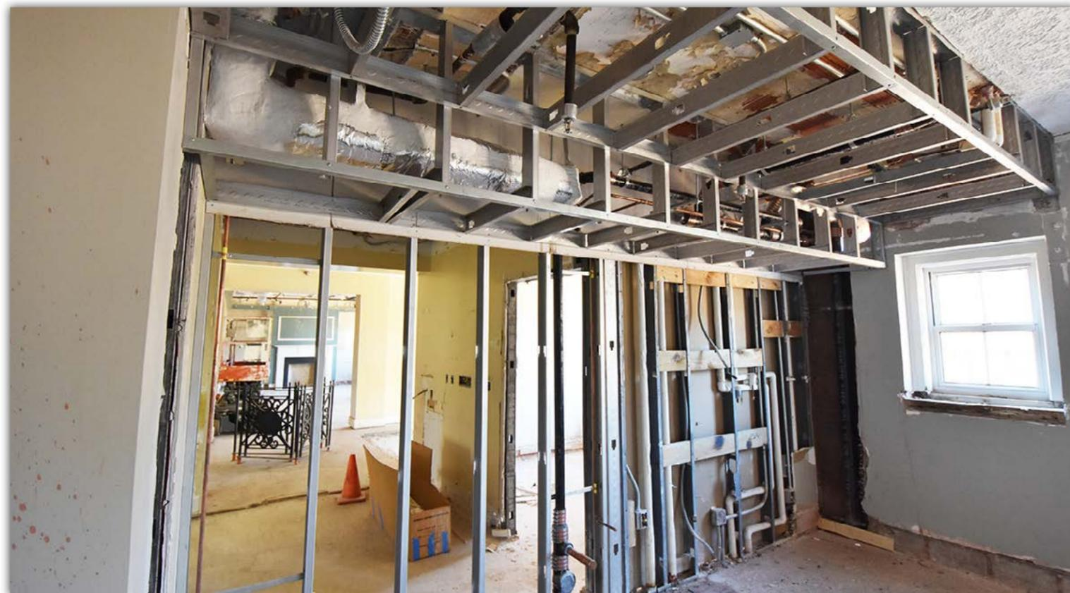
*Wooden wall studs are being replaced with metal framing.*
