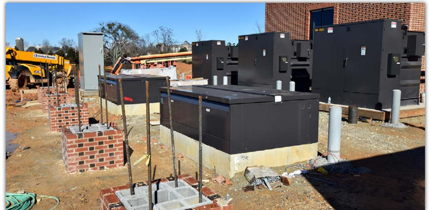
*Primary switches and transformers were recently installed and energized by Facilities Management Electrical Distribution. Construction of the brick columns that will enclose the electrical yard is underway.*
