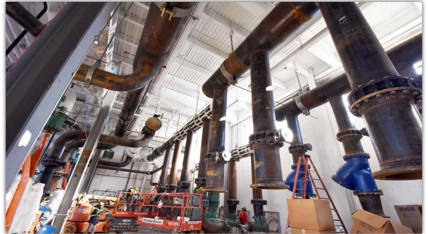
*Installation of the main hot and chilled water distribution piping in the plant.*
