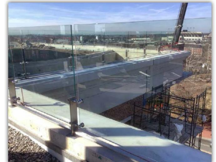
*Installation of the glass hand railing is taking place on the rooftop terrace.*
