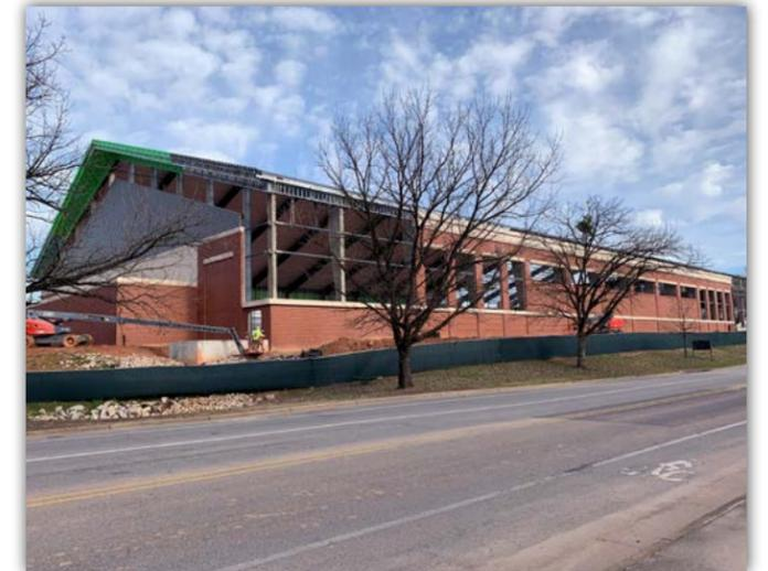
*Installation of precast brick wall panels continues on the indoor practice facility.*
