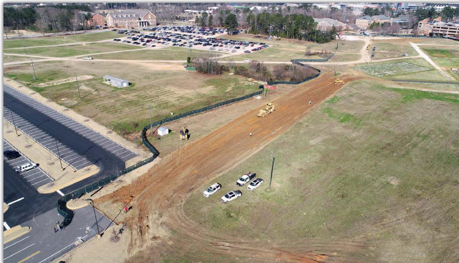
An aerial view of the Duncan Drive extension site where initial site grading and installation of the construction fencing has begun.
