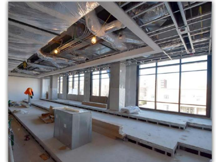
*Final framing and ceiling installation is underway in the culinary exhibition laboratory.*
