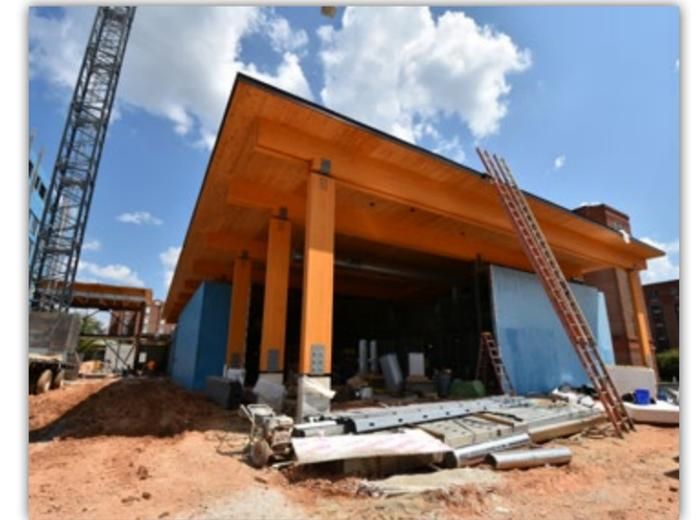
*The cross-laminated timber and glue-laminated column and beam structure of the Hey Day Market nears completion.*
