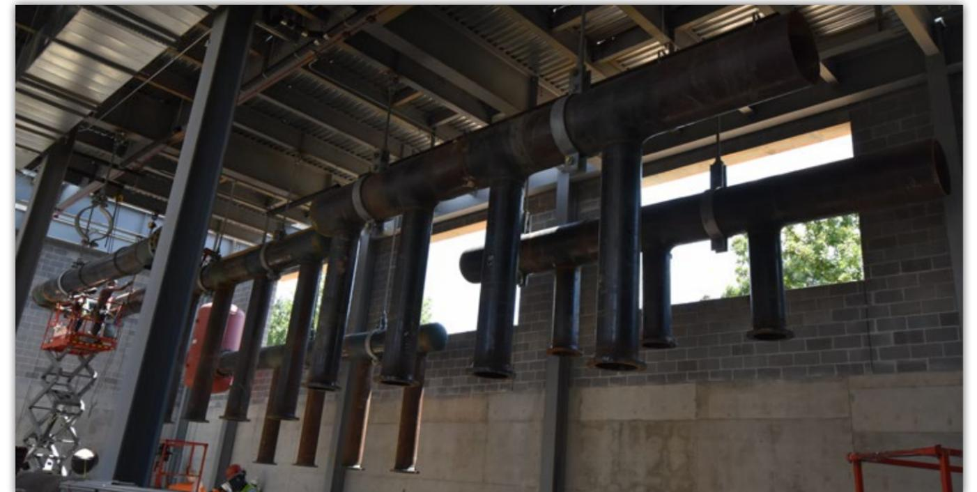
*Piping for the new chiller units is in place awaiting chiller installation.*
