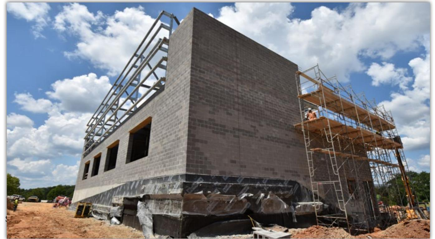
*A close up of the exterior of the building with block installation ongoing to support future brick work.*
