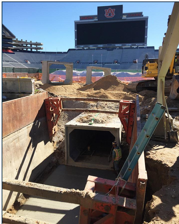
Six-by-8 box culvert being installed underneath the north end zone.
