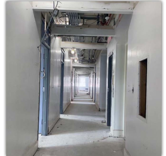
*A Broun Hall corridor has received a first coat of paint and is ready for ceiling tiles to be installed.*
