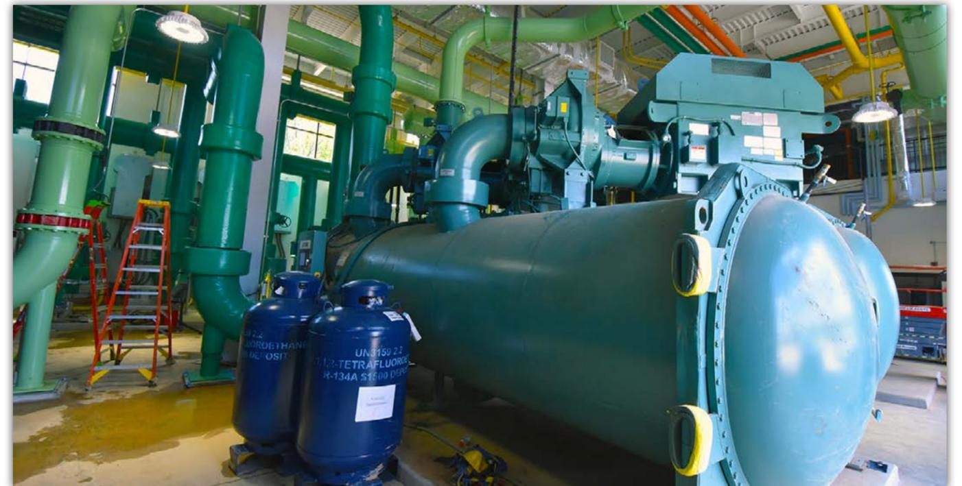
*The two 2,500-ton chiller units have been installed.*
