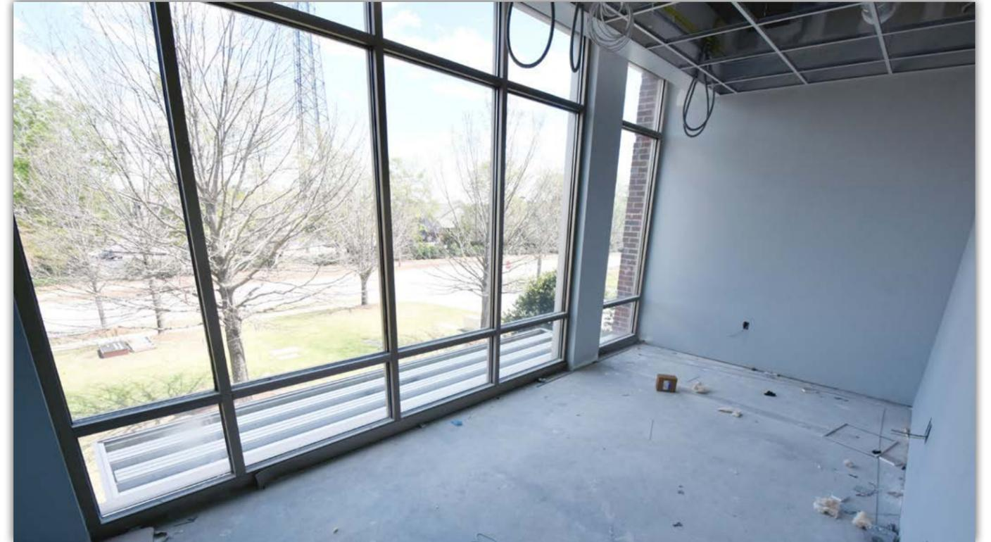
*Walls have been painted and installation of mechanical, electrical and fire protection systems in the ceiling is ongoing.*
