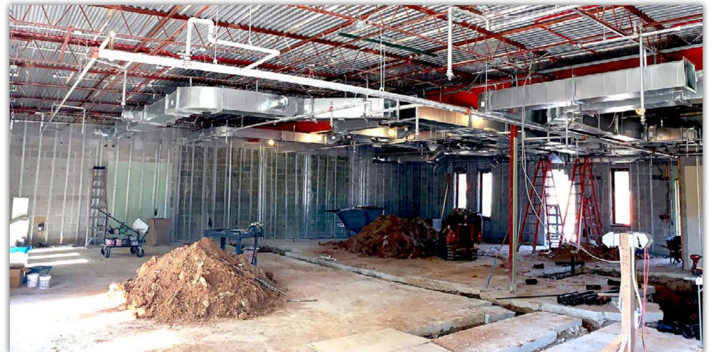
*Installation of overhead mechanical, electrical and fire protection systems is underway inside the Dawson Building.*
