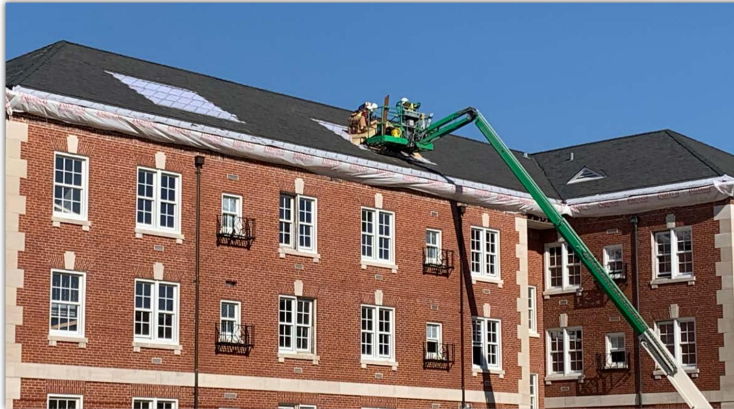
*Roof work on Harper Hall includes installation of vents and gutter repairs.*
