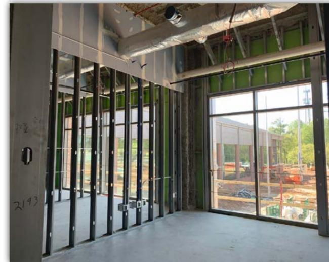
*Metal wall frames have been erected in the office areas on the second floor.*
