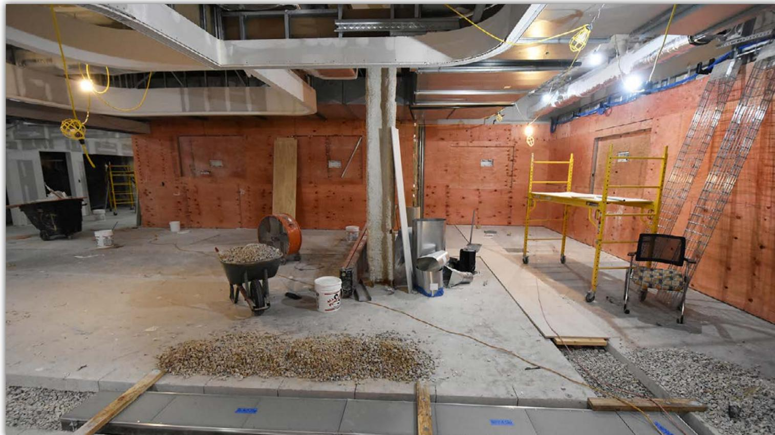
Walls have been framed, and power and data cables are being placed in the floor ducts.
