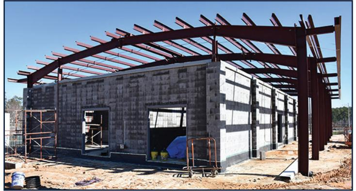
The masonry and metal are complete on the storage building.
