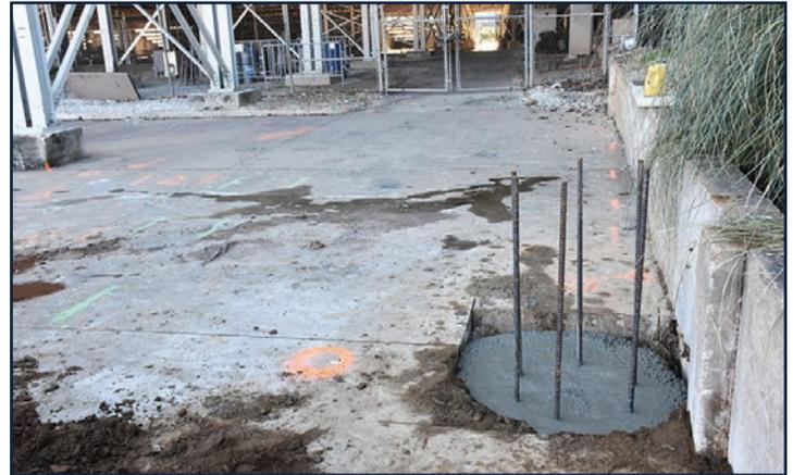
Installation of drilled columns for new structural steel has begun.
