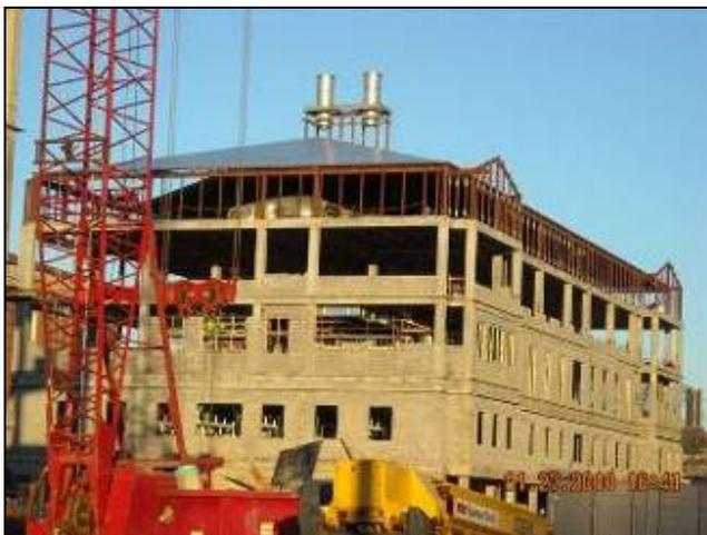
Concrete frame, exterior block and roof structure underway.
