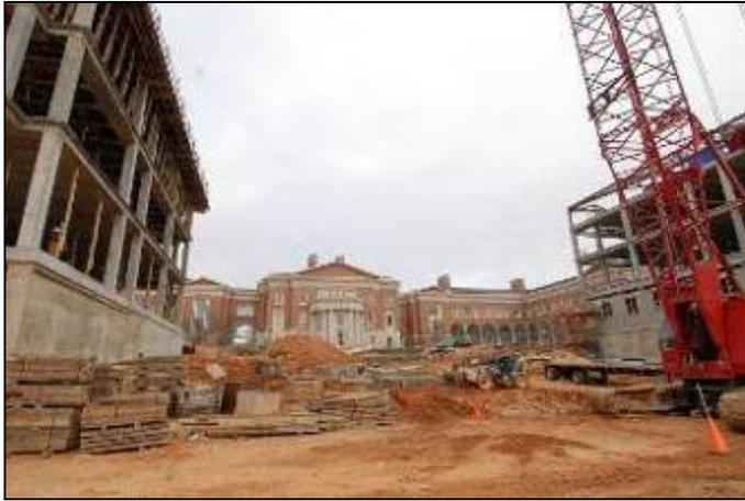
Reinforced concrete frame construction looking north towards Shelby Center Phase I. #
