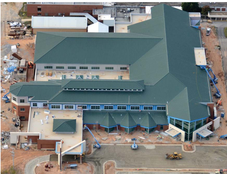
Aerial view of Small Animal Teaching Hospital - Phase II
