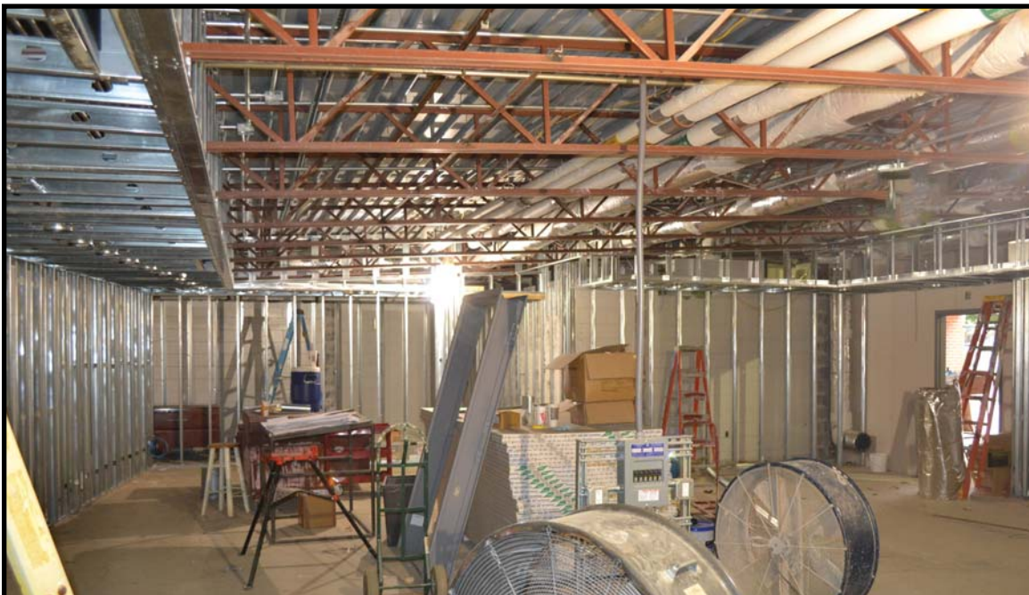
Locker room interior
