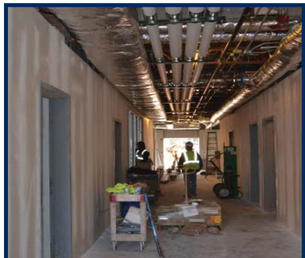
Hoerlein Hall Interior Renovations
