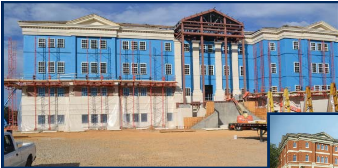
Front Elevation - Installation of Exterior Masonry and Pre-cast Concrete Panels
