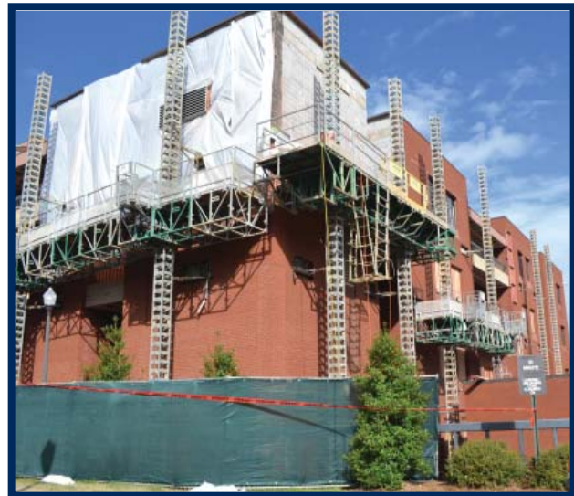
Brick Removal on East Side of Building
