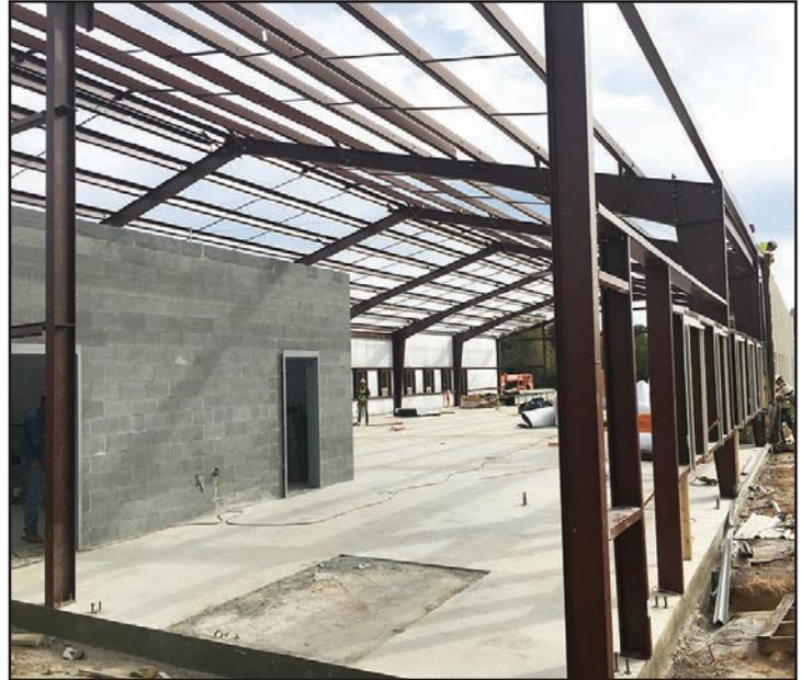
Concrete block restroom enclosure nears completion.
