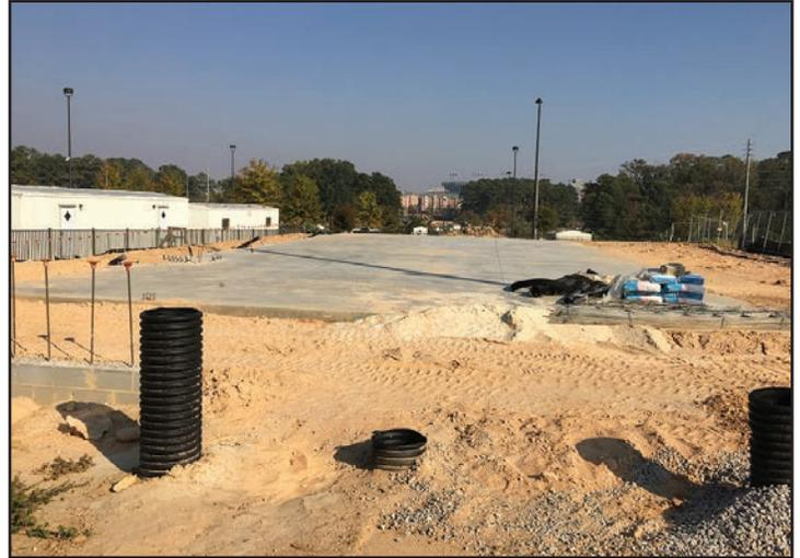
The storage building's concrete pad is complete.
