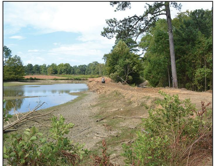
Compactor works to repair the pond dam.
