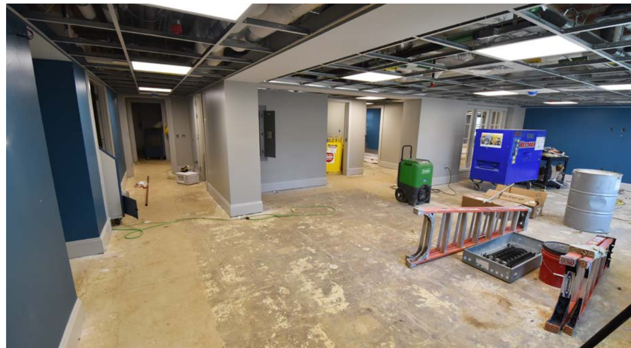
The basement walls have been painted. The space is ready for ceiling tiles, followed by flooring.
