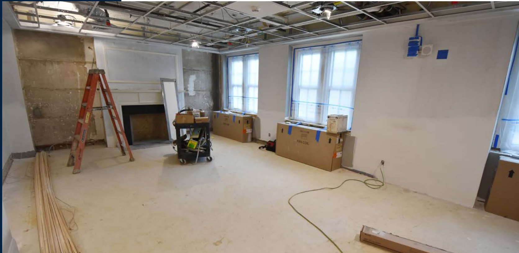
Drywall is being installed in the Harper Hall common area.
