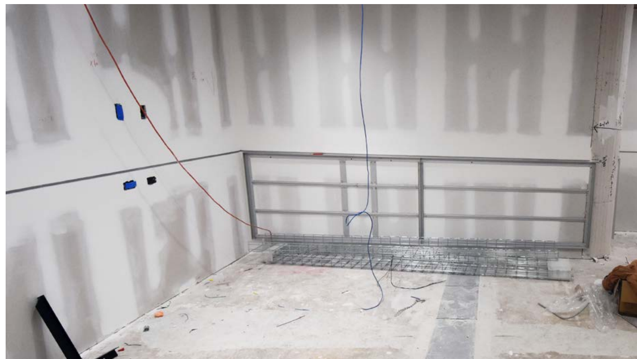
The wall protection framework is being installed in the Tiger Lab.
