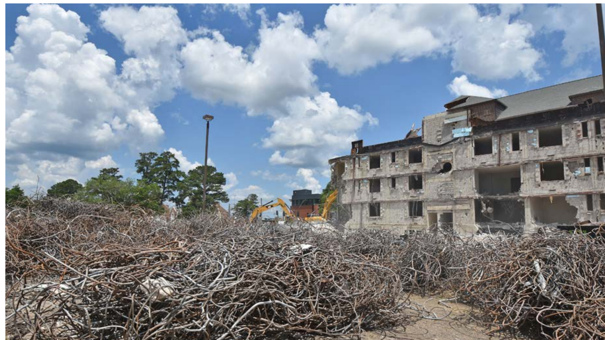
Metal from each building is collected and sent to a local recycling center.
