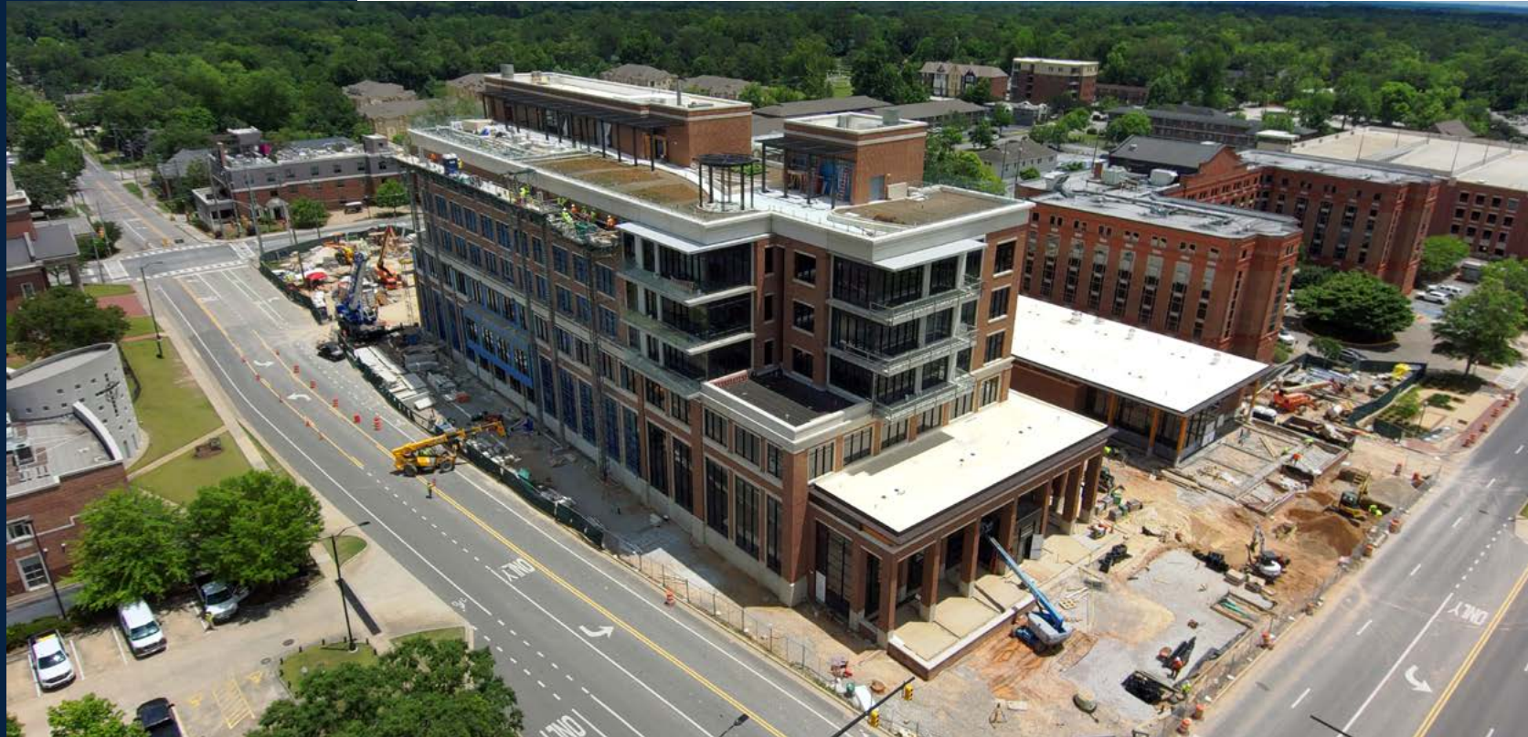
Concrete walkways are being poured in front of the Tony and Libba Rane Culinary Science Center, while brick work continues on the Thach Avenue (north) side of the building. Photo: Multivista
