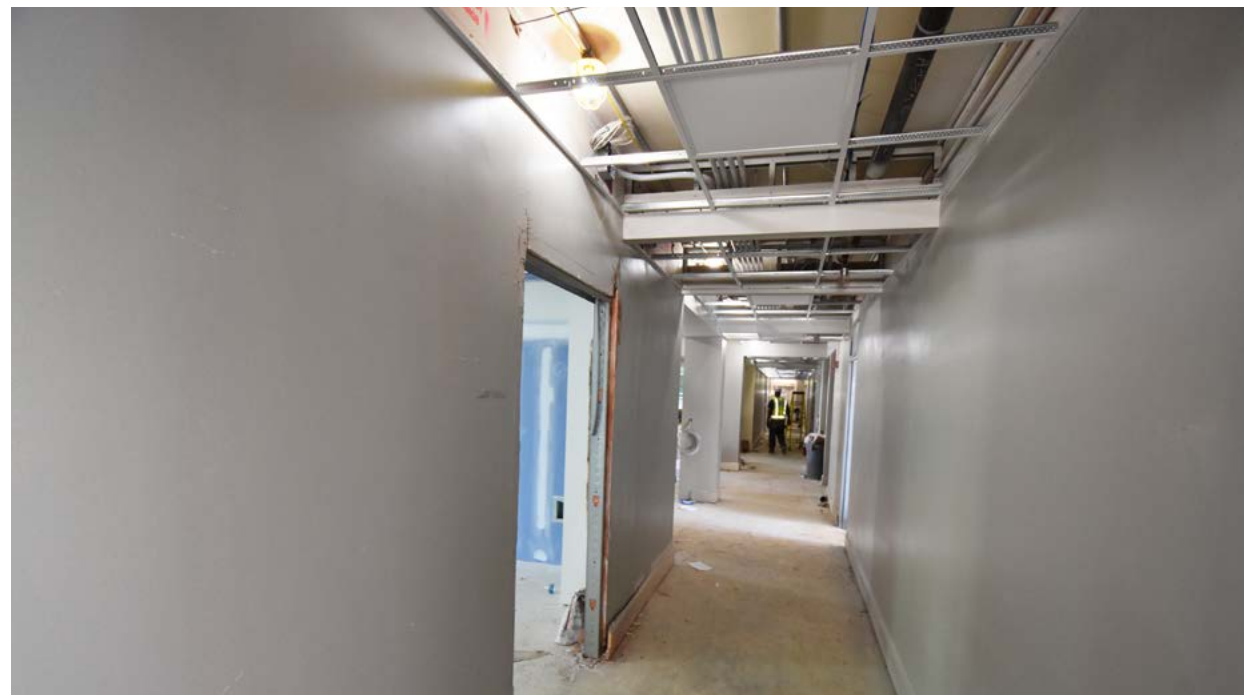
First coat of paint has been applied to the hallway walls on the first floor. Floor and door trim will soon be installed.
