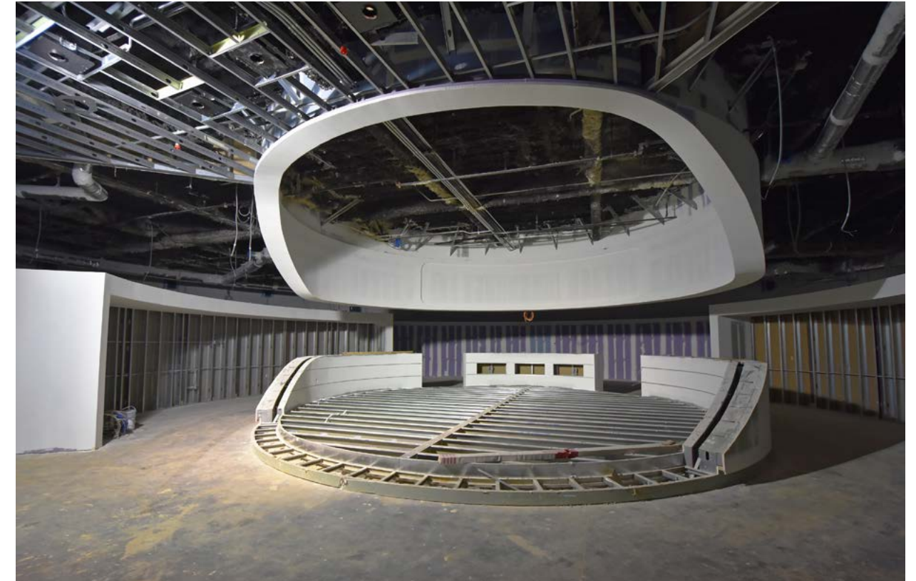
Framing for a feature ceiling that mimics eagle feathers and rolled Auburn Oaks is underway in the Huddle Locker Room.
