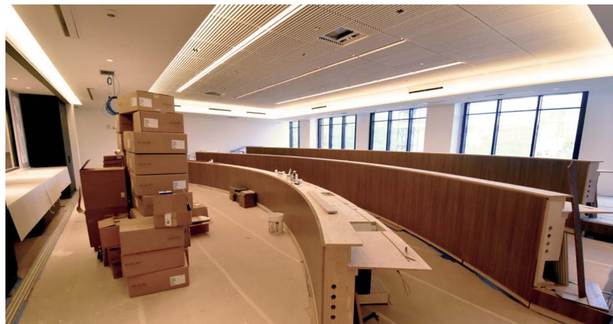
Wood panels are being installed in the culinary exhibition laboratory.
