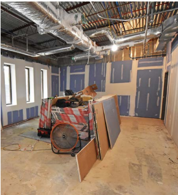
Sheetrock installation is ongoing in the Dawson Building, which will house the Early Learning Center.
