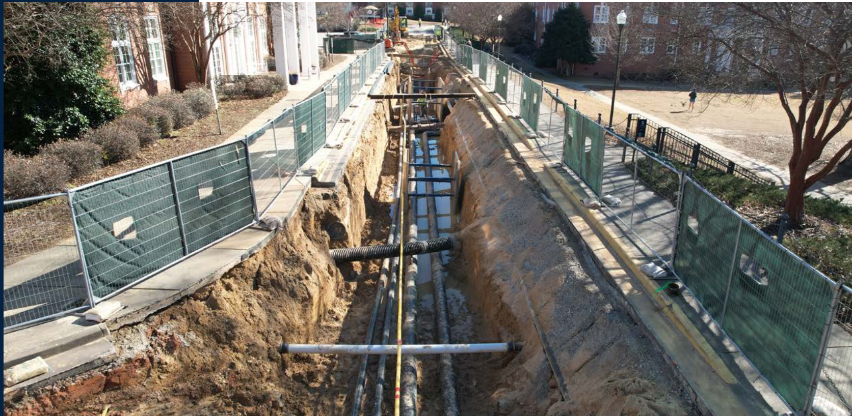
Underground hot water and chilled water line installation continues along Quad Drive.
