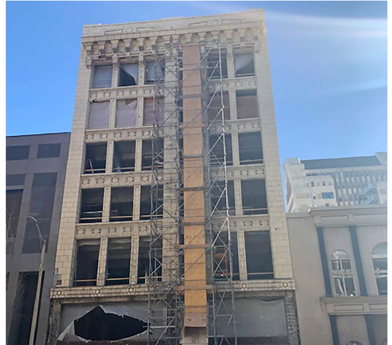
The front sign has been removed, and restoration work has begun on the terracotta facade.
