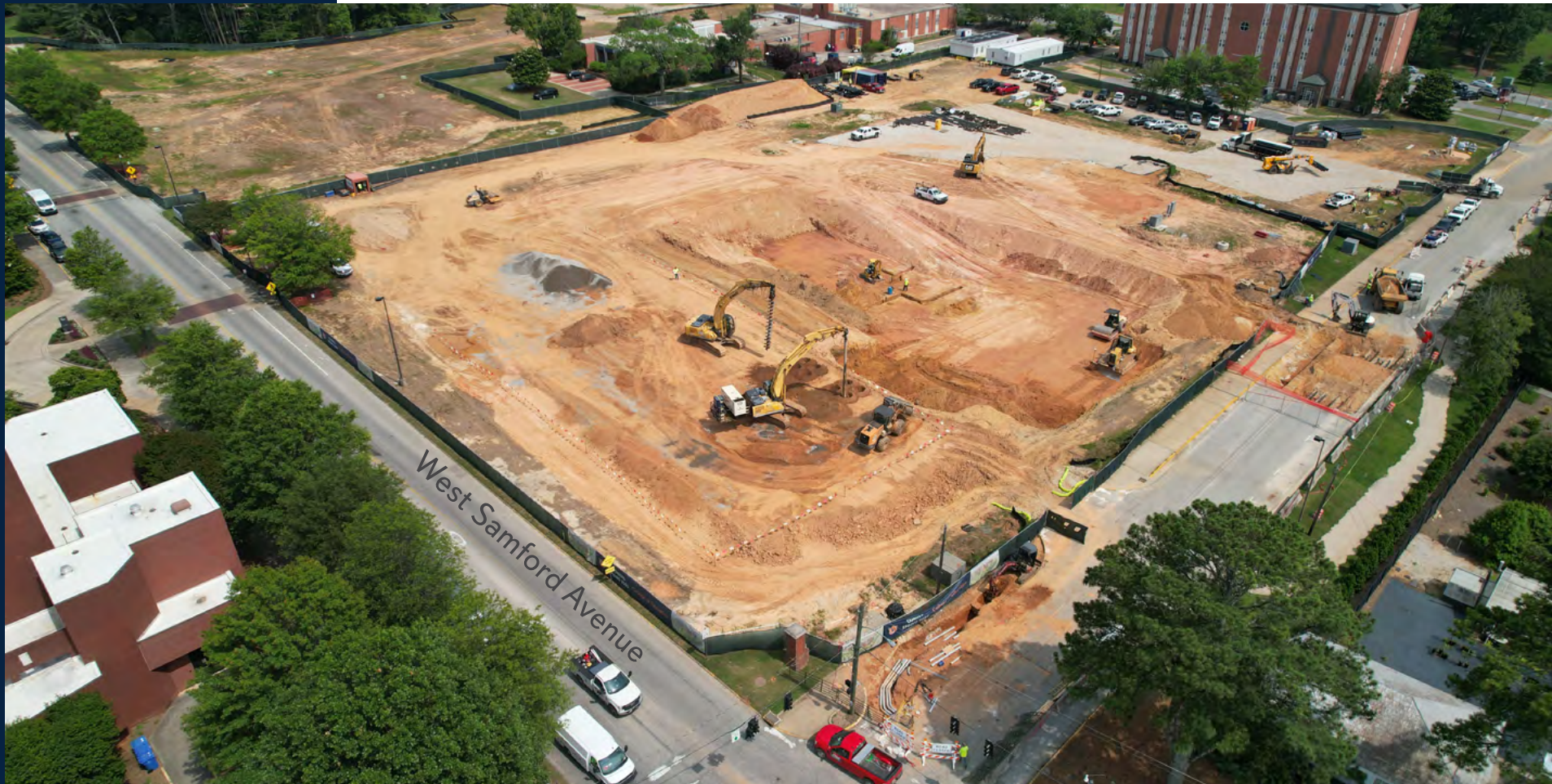
Building pad preparation and basement excavation has begun at the College of Education building site.
