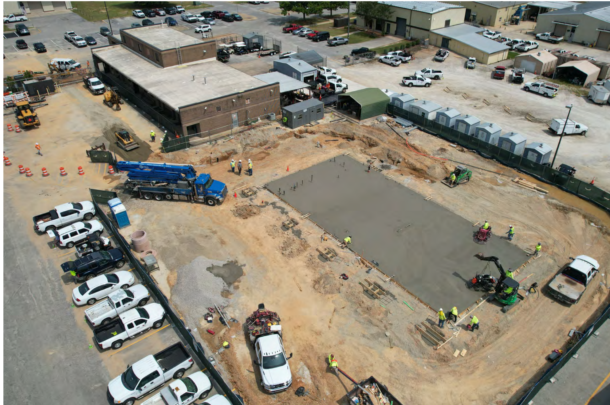
An aerial photo of the Facilities Management Training Center site where concrete is being poured for the building's foundation.
