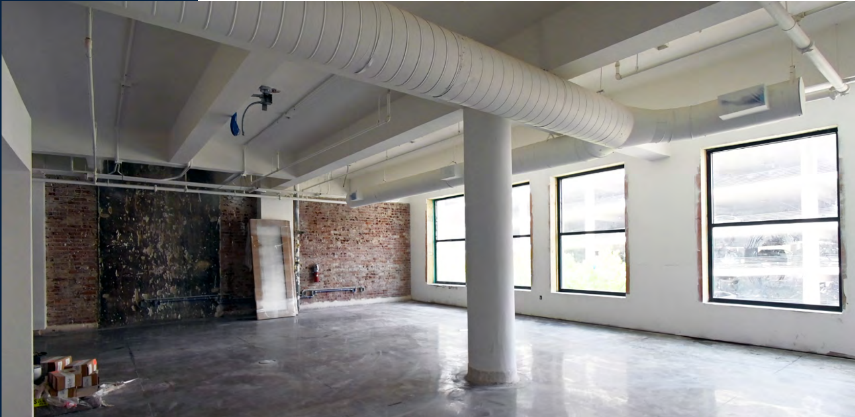
Ground and polished floors are in progress on the north side workspace.
