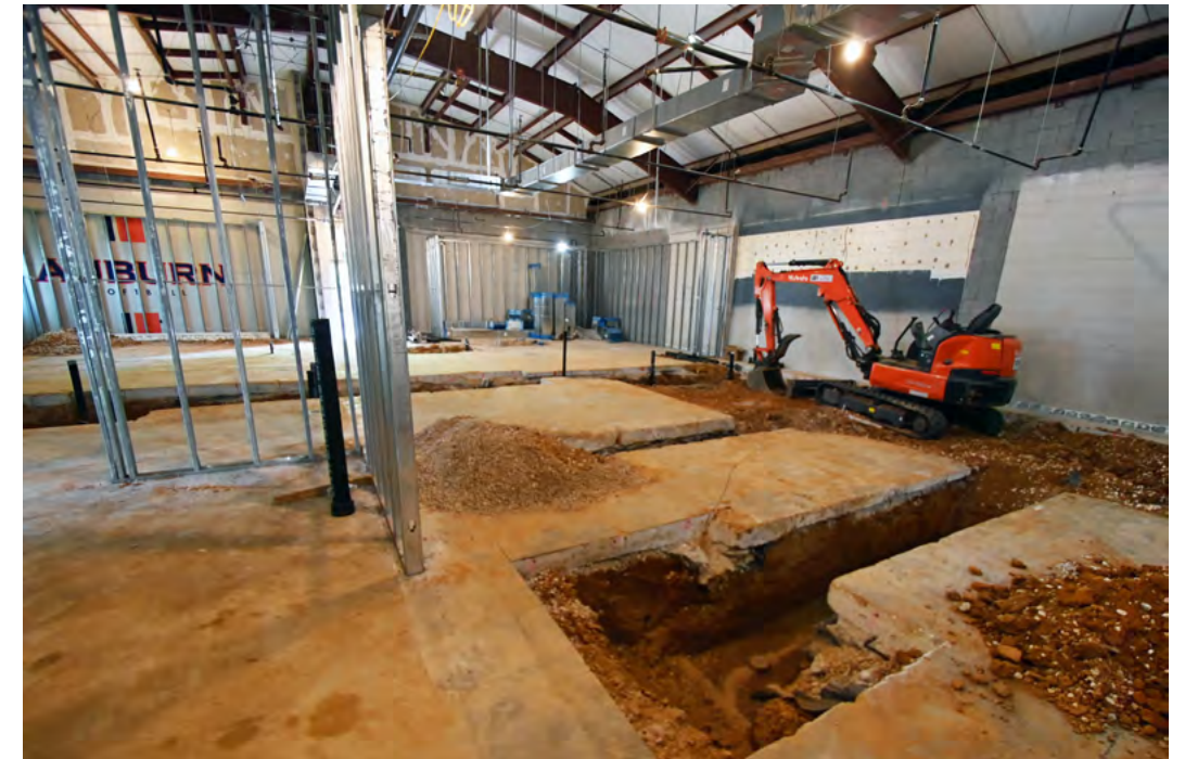
Trenches are being dug for installation of plumbing lines in the new locker rooms.
