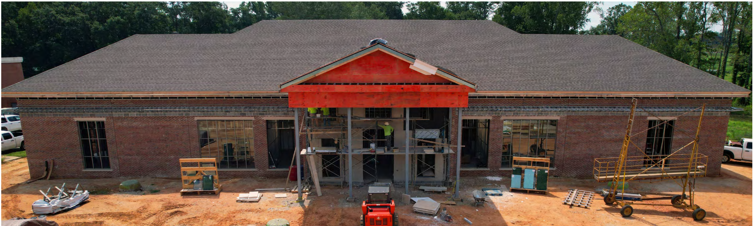
Installation of the brick and stone work continues on the exterior of the building.
