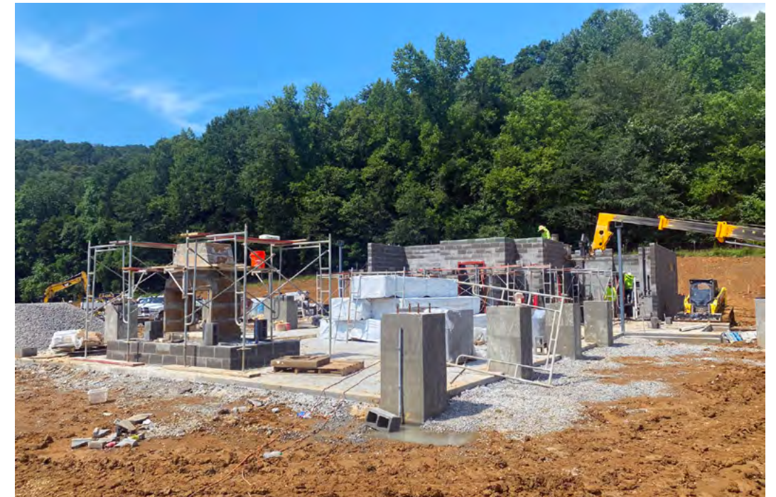
The lower part of the concrete support columns for the outdoor area of the pavilion are complete.
