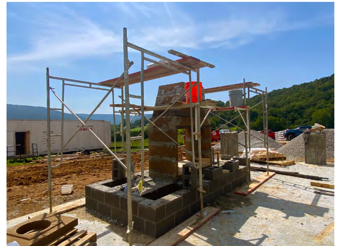
The foundation and structure for the 28-foot-tall fireplace nears completion.
