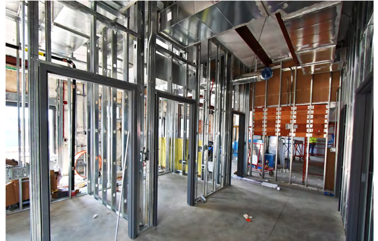
Walls are being framed for the two meeting spaces and restrooms.
