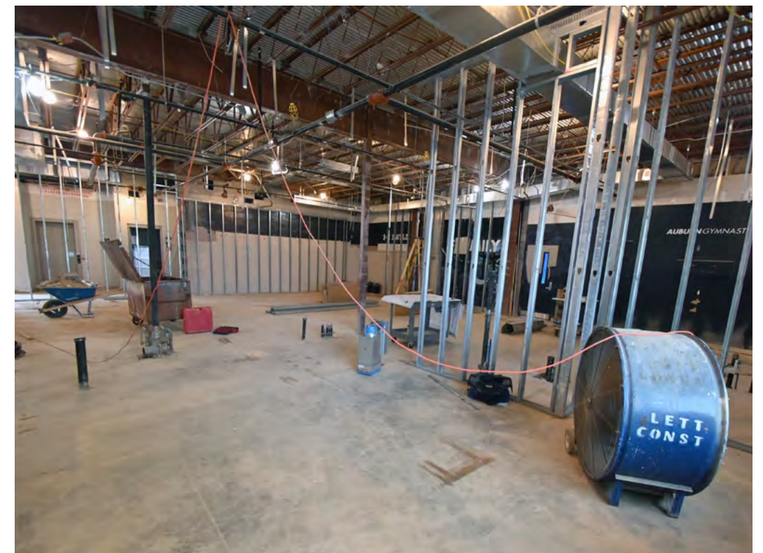
Wall framing is taking place in the new locker rooms.
