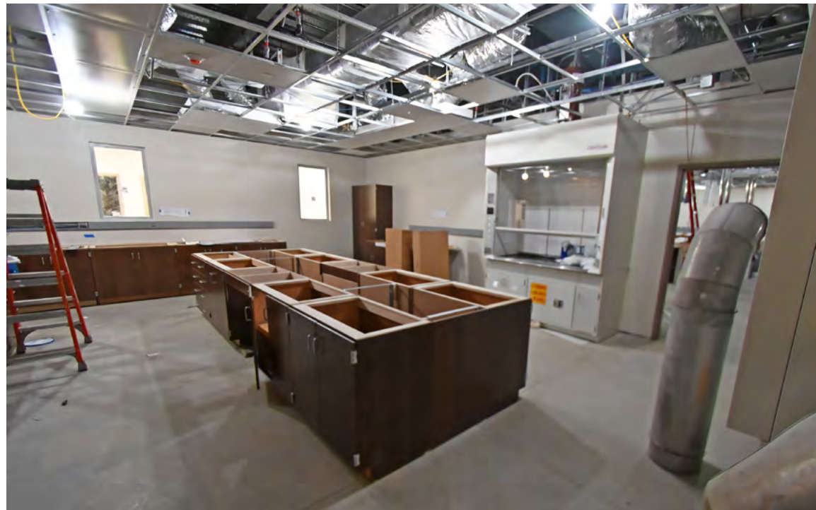
Casework is set and build-out of lab spaces is underway.
