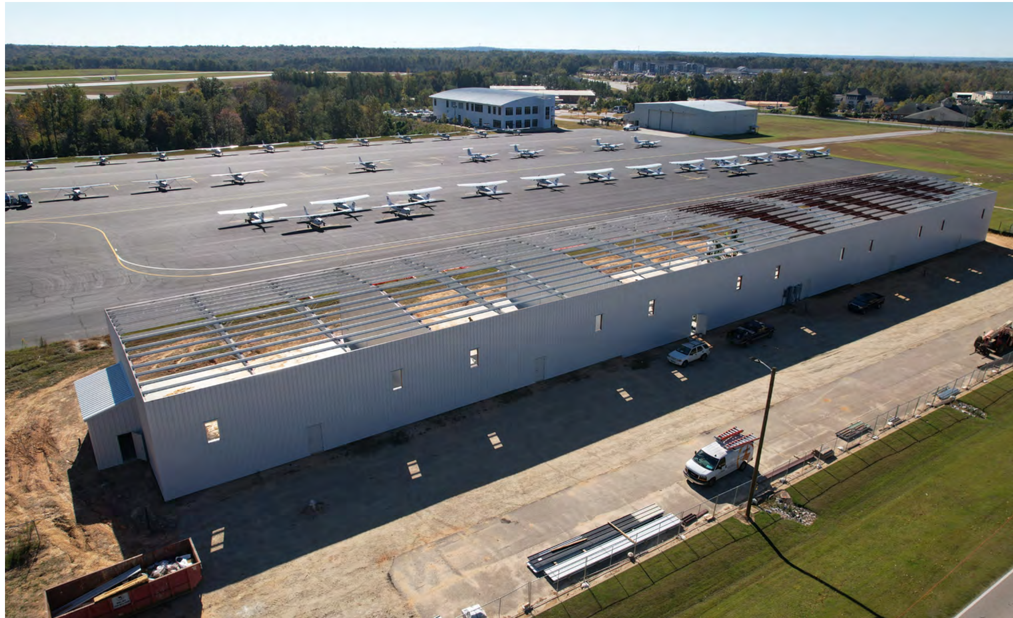
Three sides of the exterior walls are in place for the pre-engineered metal building. Next steps include installation of the hangar doors and roof panels.
