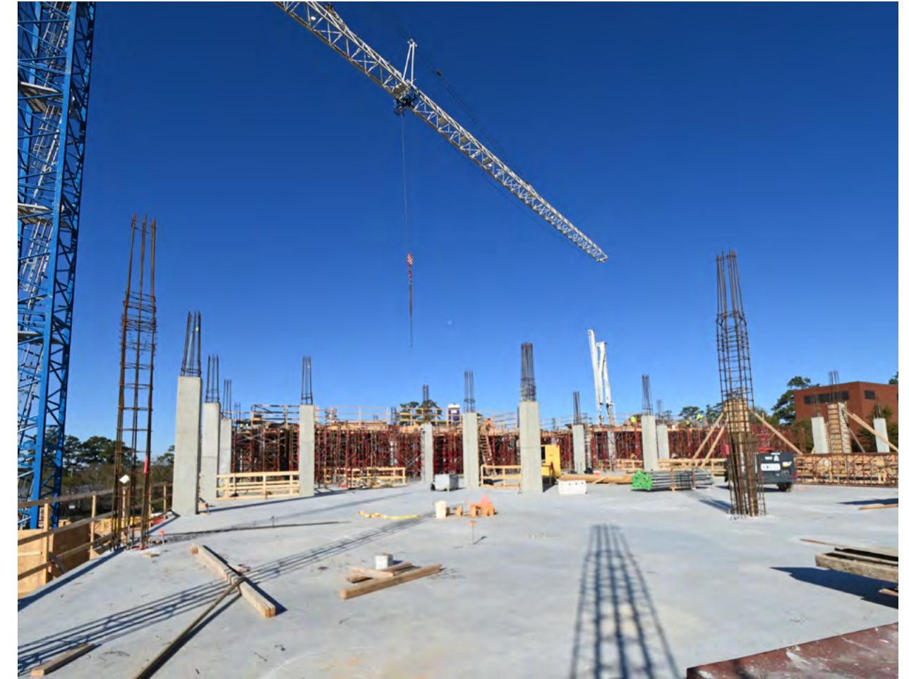
This second-floor area will house computer labs and a conference room upon completion. Concrete was recently placed along with rebar and structural concrete columns for the third floor.
