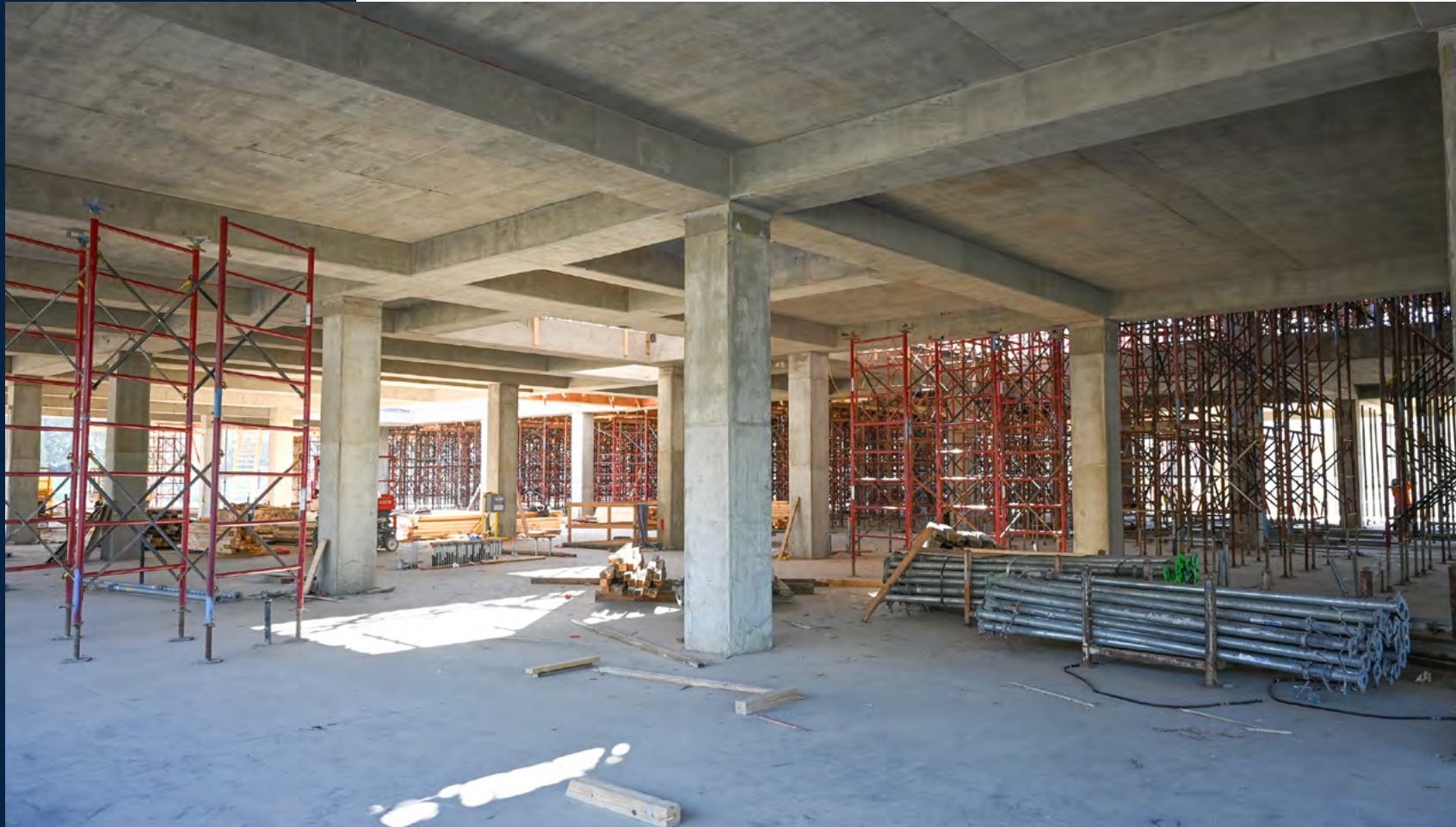
This section of the College of Education building's first floor has all structural concrete placed and will house the EAGLES program upon completion.
