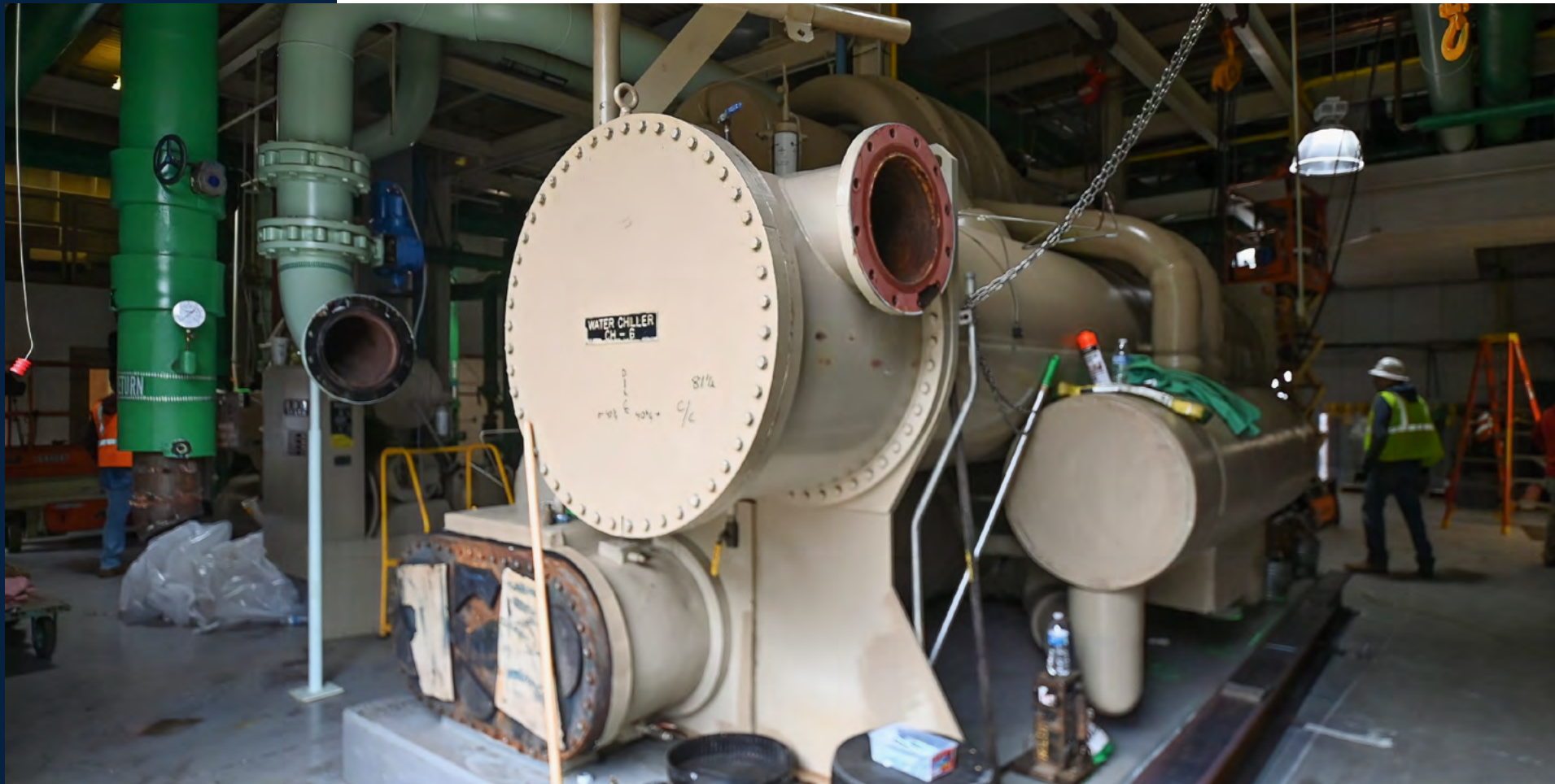
A 1,000-ton chiller at Chilled Water Plant 3 is being prepped for removal and replacement.
