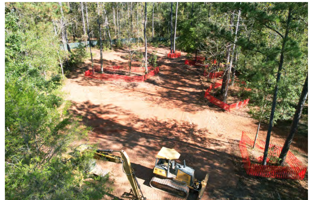
Clearing and grading of the project site has begun in preparation for the new facility.
