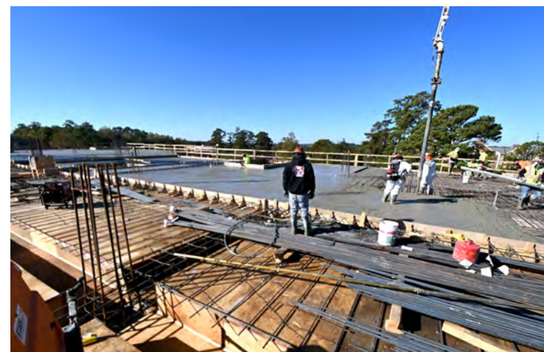
Concrete is being poured for a third-floor section of the building. This section of the building will house several faculty and administrative offices.
