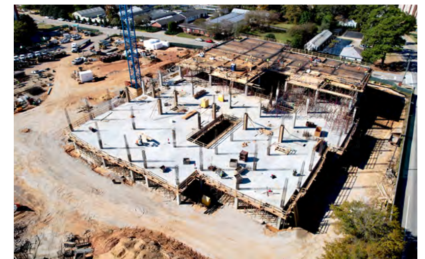
An overhead view of the completed concrete sections of the building. More concrete will soon be poured for the basement entrance and completion of the third-floor sections.
