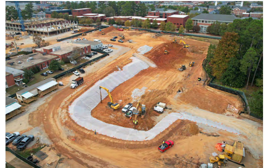
Excavation for the building C basement is nearing completion. All three buildings will be connected via a basement level.
