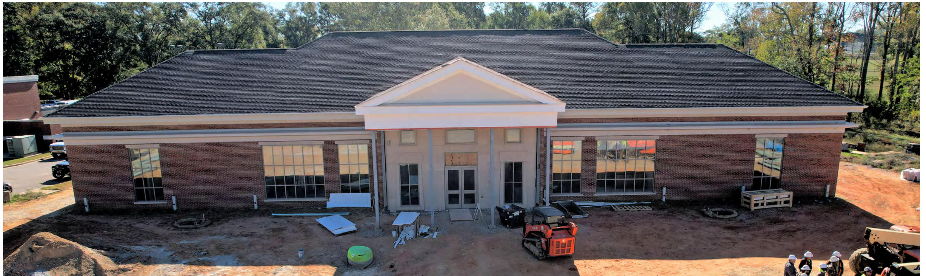
Brick installation is complete, and the remaining exterior materials are being installed.
