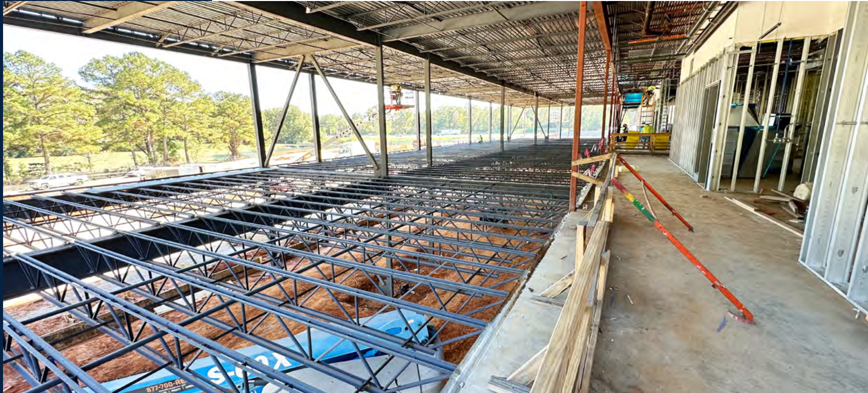
The building addition is now framed. Next steps include pouring concrete and installing metal decking.
