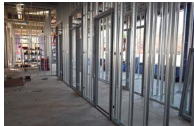
Interior walls are being framed throughout the facility.
