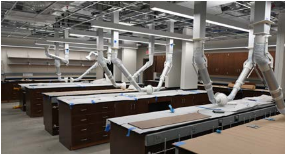
Lab installation is nearing completion with the mechanical, electrical and plumbing installed.
