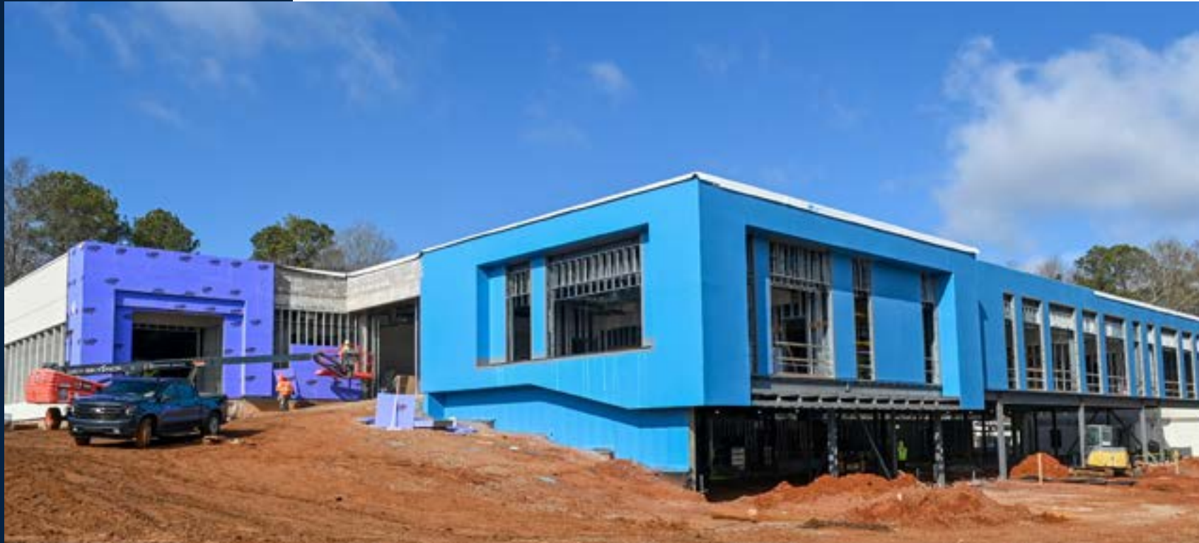
A protective waterproof barrier has been installed on the outside of the building.
