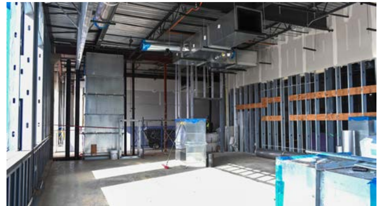
In-wall and overhead mechanical, electrical and plumbing systems installation continues in this new lab room.
