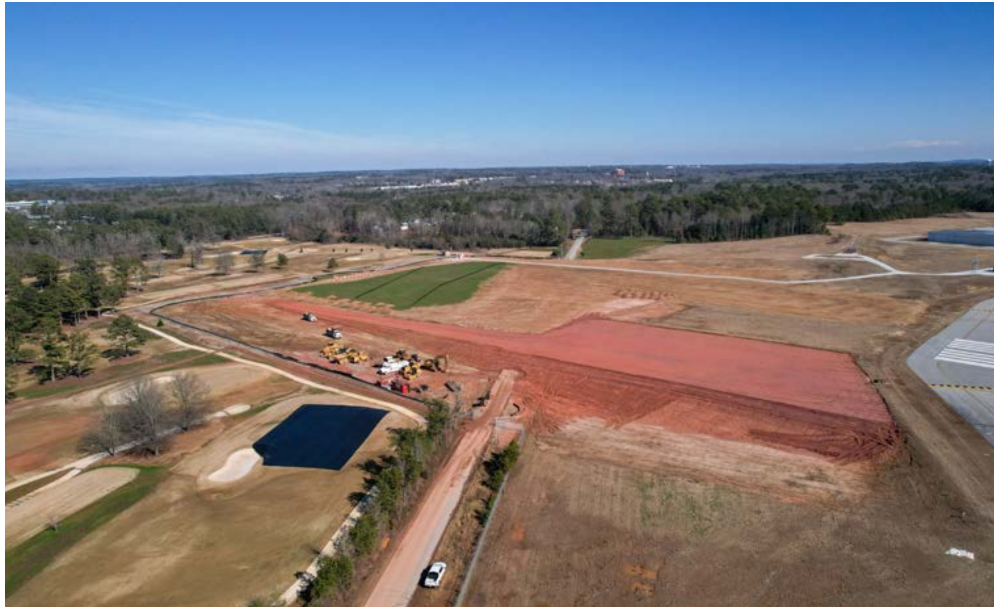
Dirt fill continues to be hauled in and placed. Site preparation for the new localizer antenna platform is underway.
