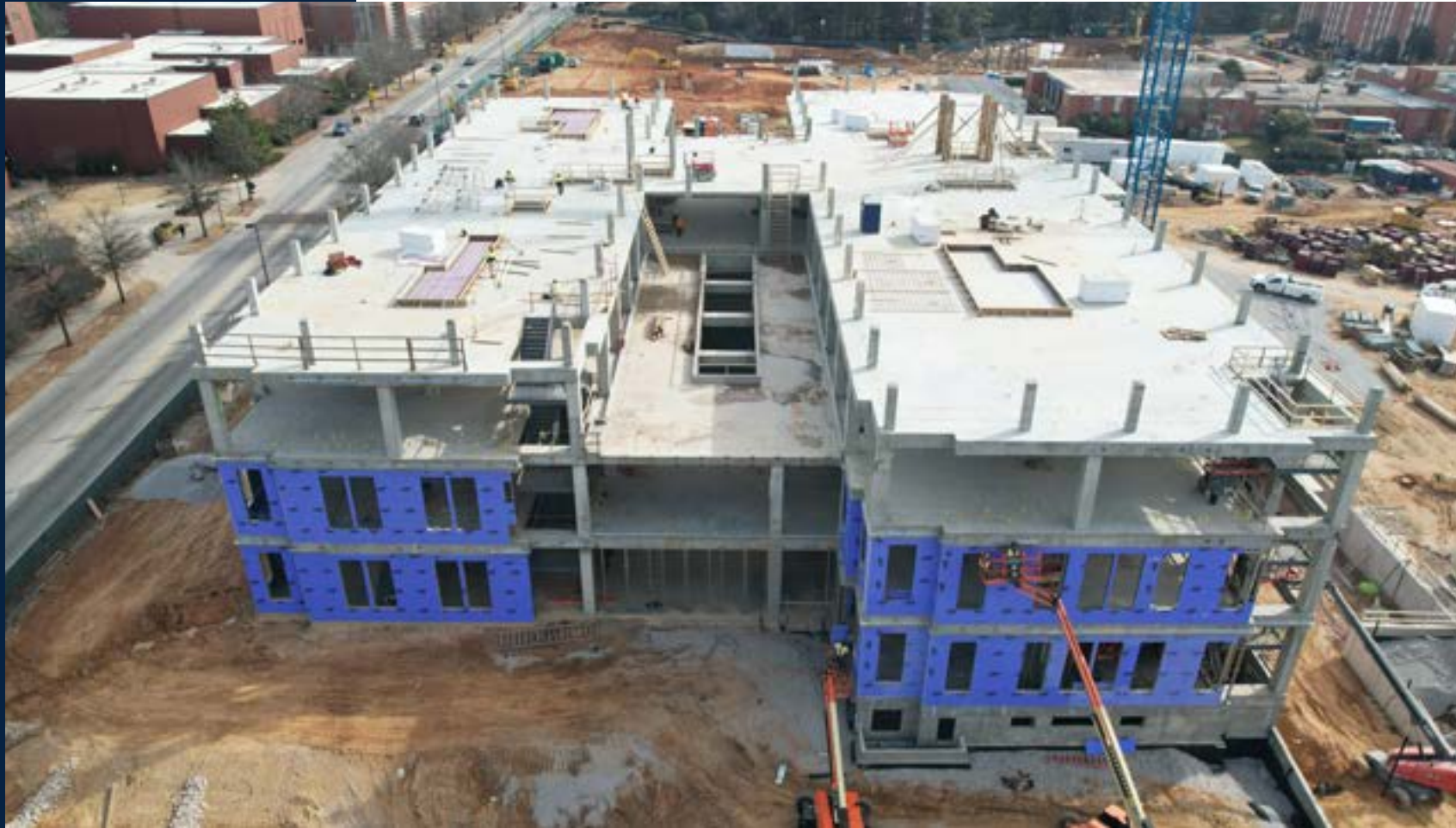
The exterior barrier is being placed on the first and second floors.
