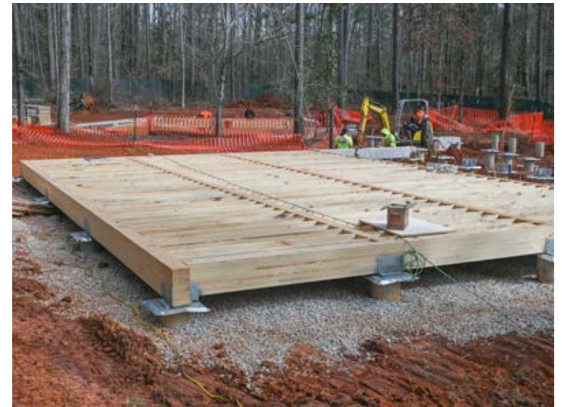
Platform framing is complete for both structures.
