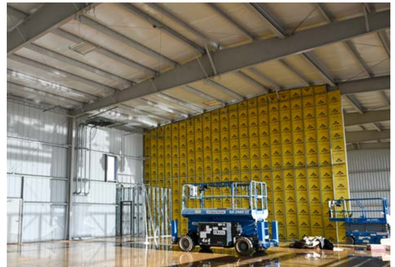
A separation wall is being constructed between the fourth and fifth bays of the hangars' pre-engineered building frame.
