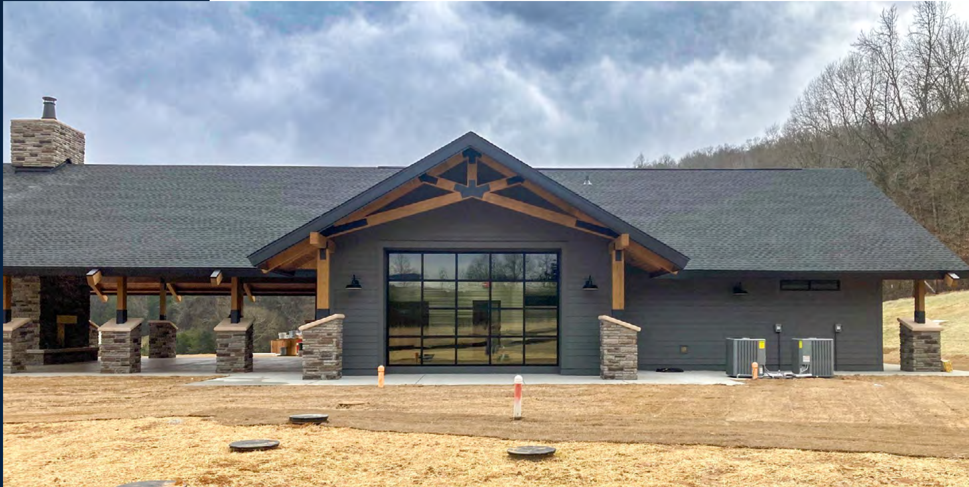
Construction of the ACES Graham Farm and Nature Center Pavilion in Jackson County, AL is complete.
