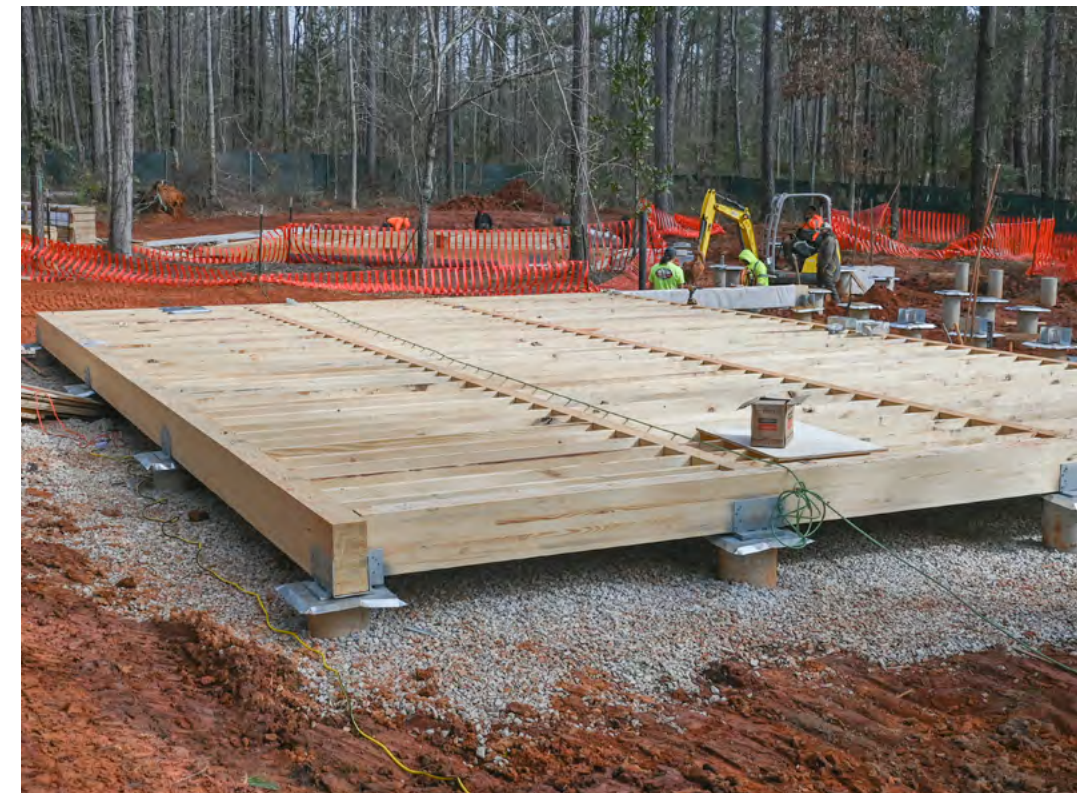
Platform framing is complete for both structures.
