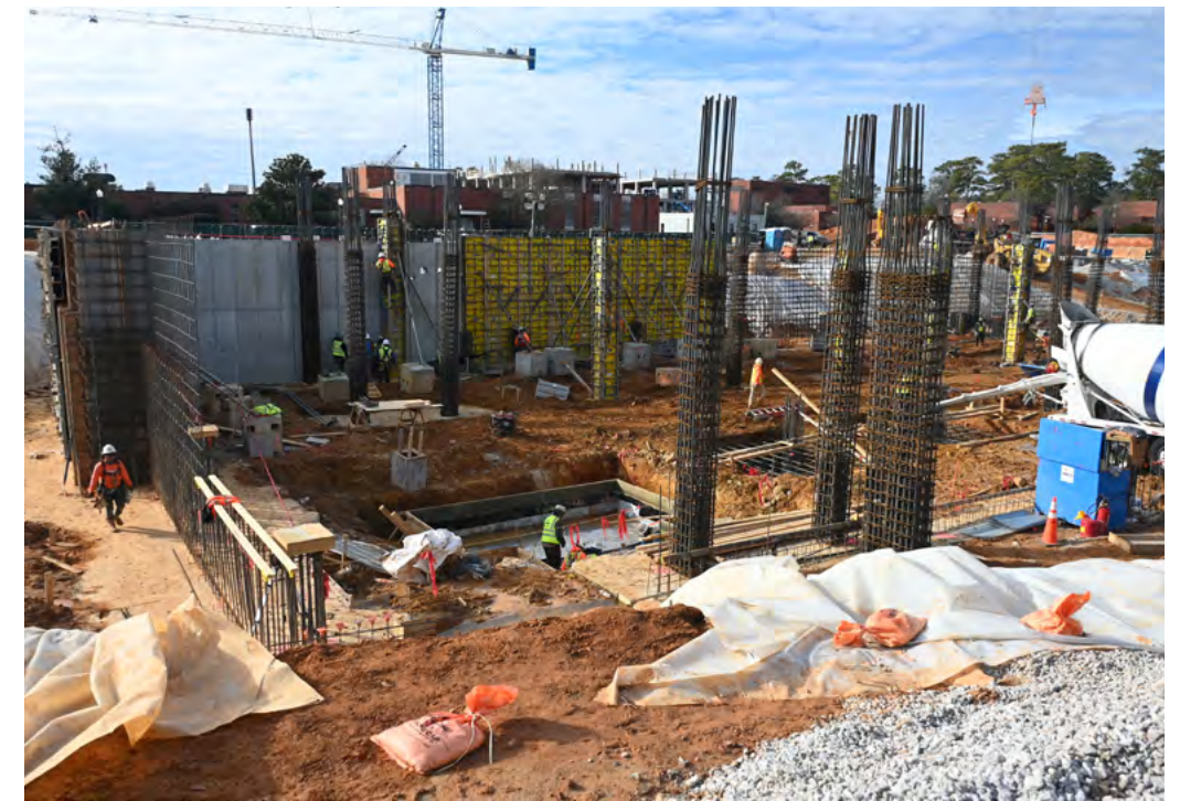
Basement walls in Building C are being formed.
