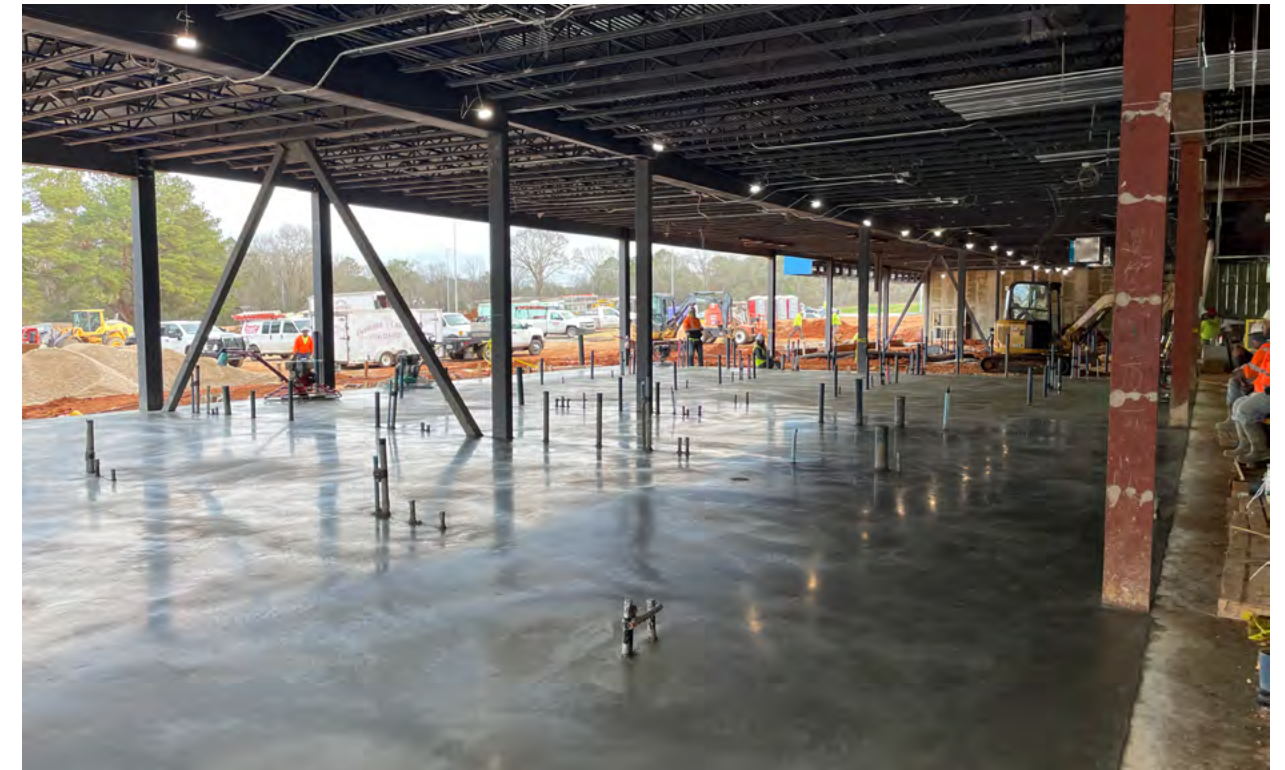
Concrete has been poured for the building's first floor addition.
