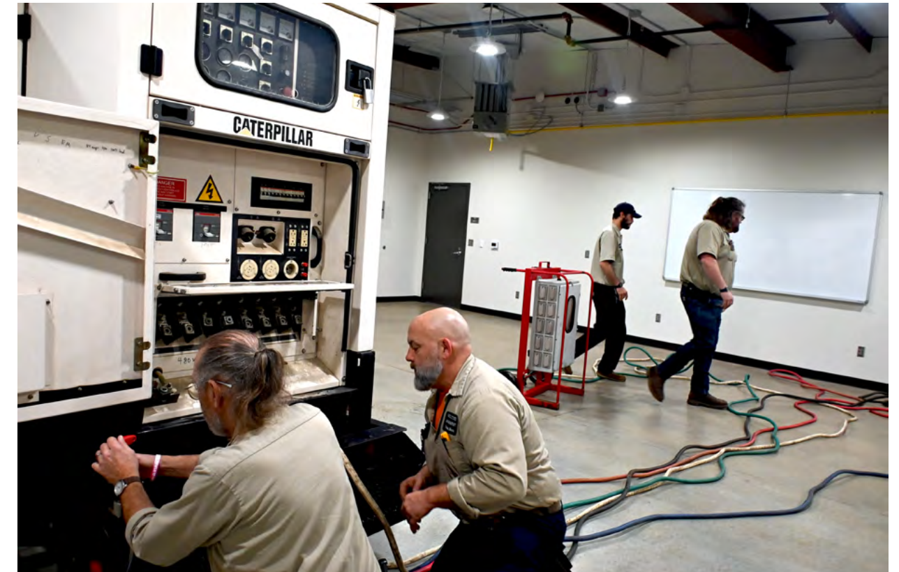
Electricians train on a portable generator inside the center's demonstration room.
