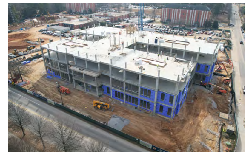
The concrete structure is complete on all three floors.
