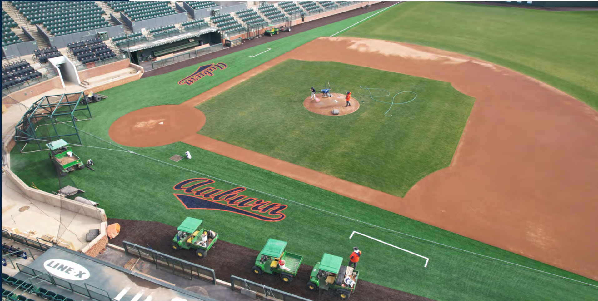
Artificial turf has been installed along the baselines and behind home plate.
