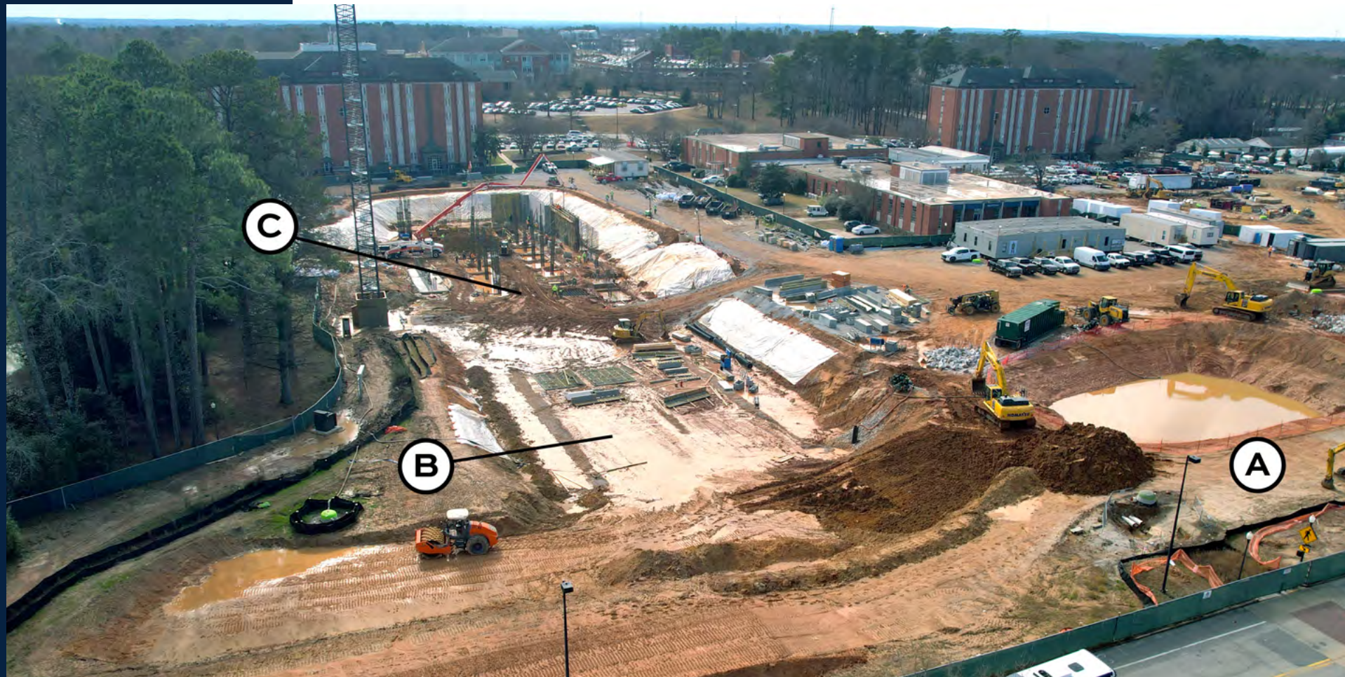
Basement walls in Building C are being formed.
