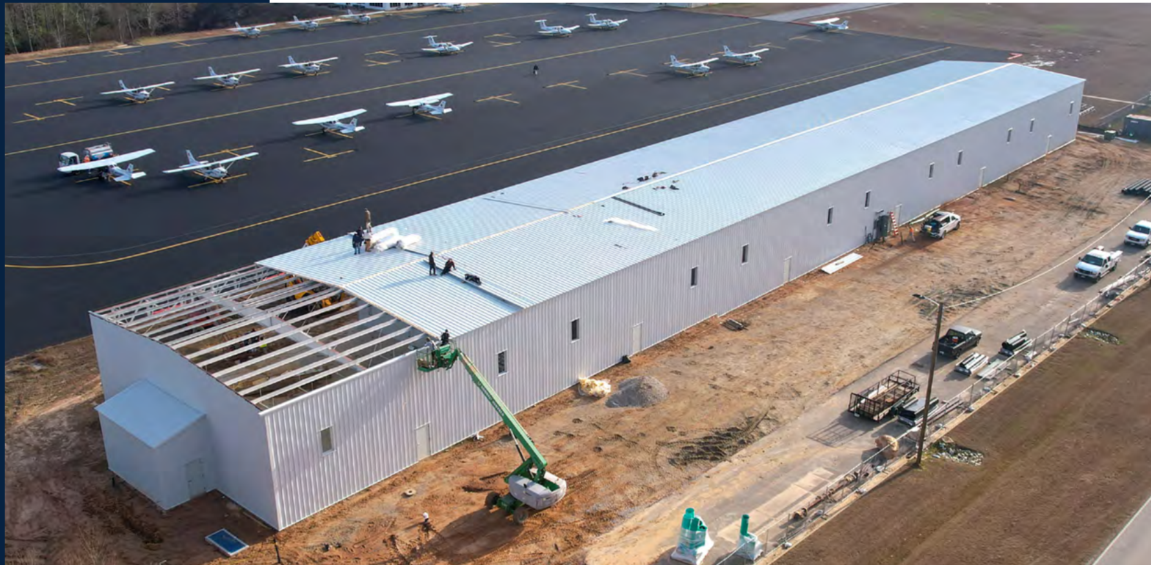
The roof is being installed on the new corporate hangar.
