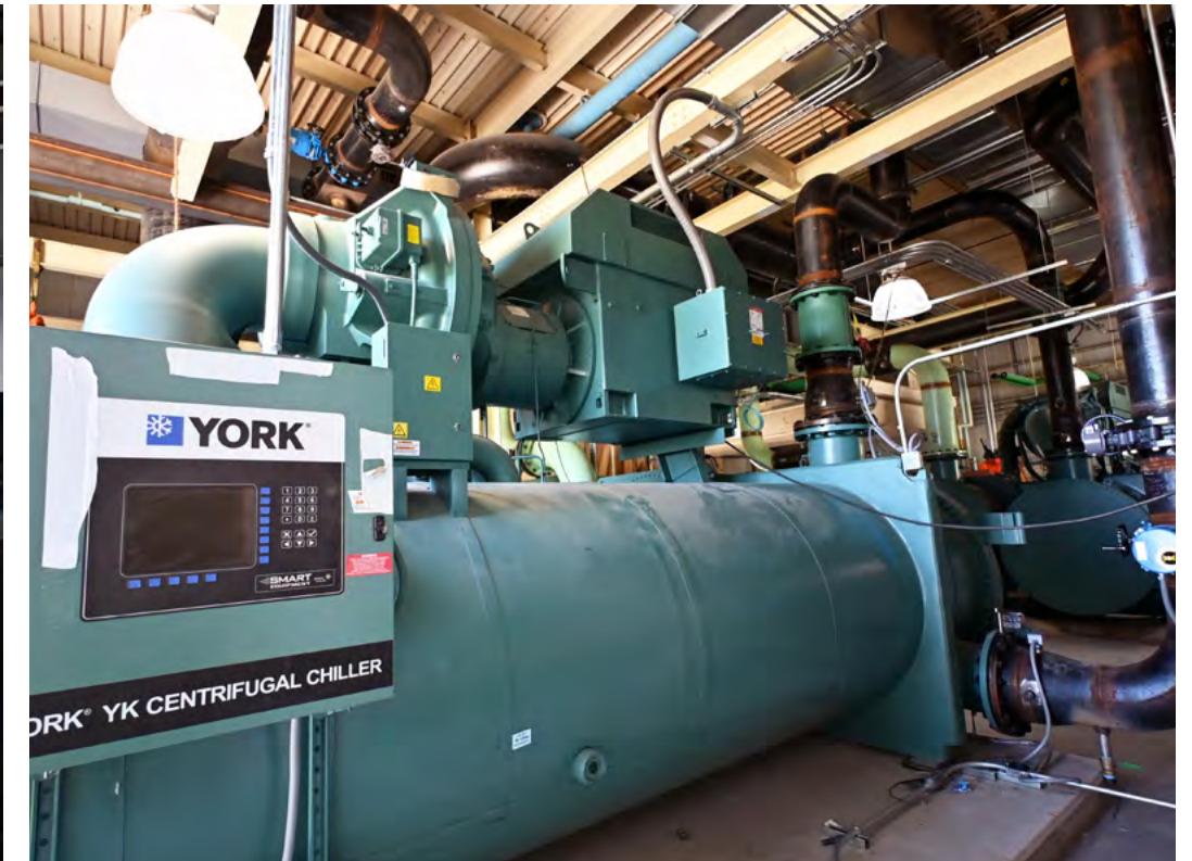
The new chiller has been installed.
