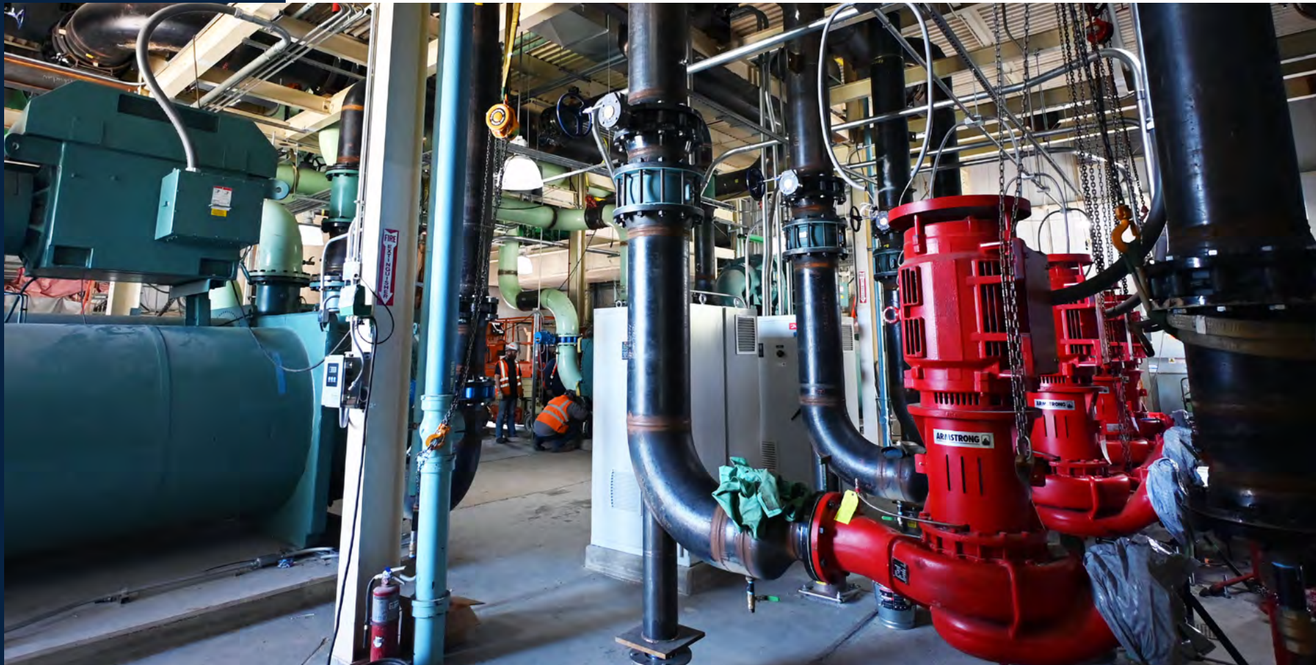
Reconfiguration of the new piping system is underway.
