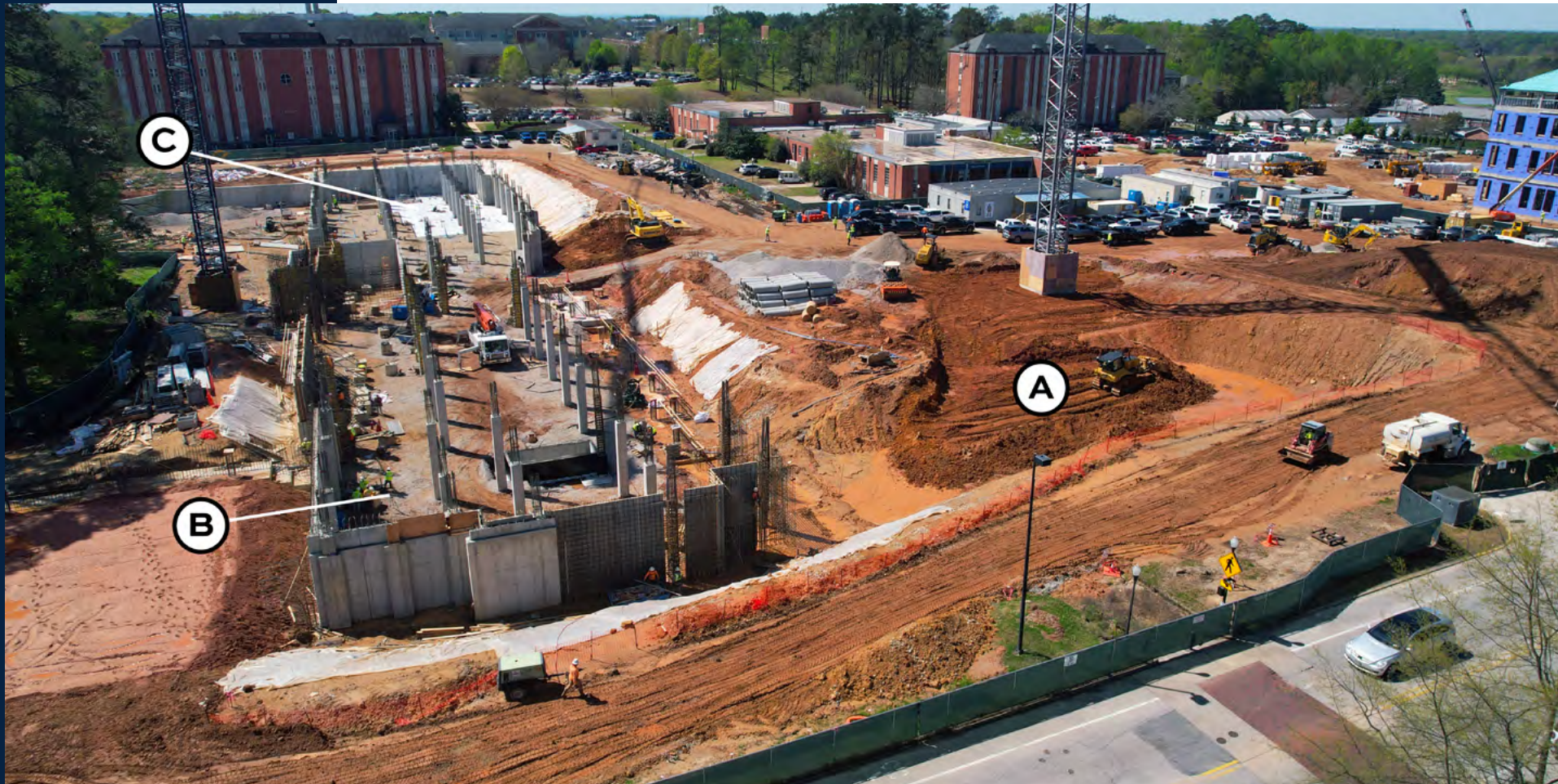
Structural concrete columns are in place to support the first floor of Building C.
