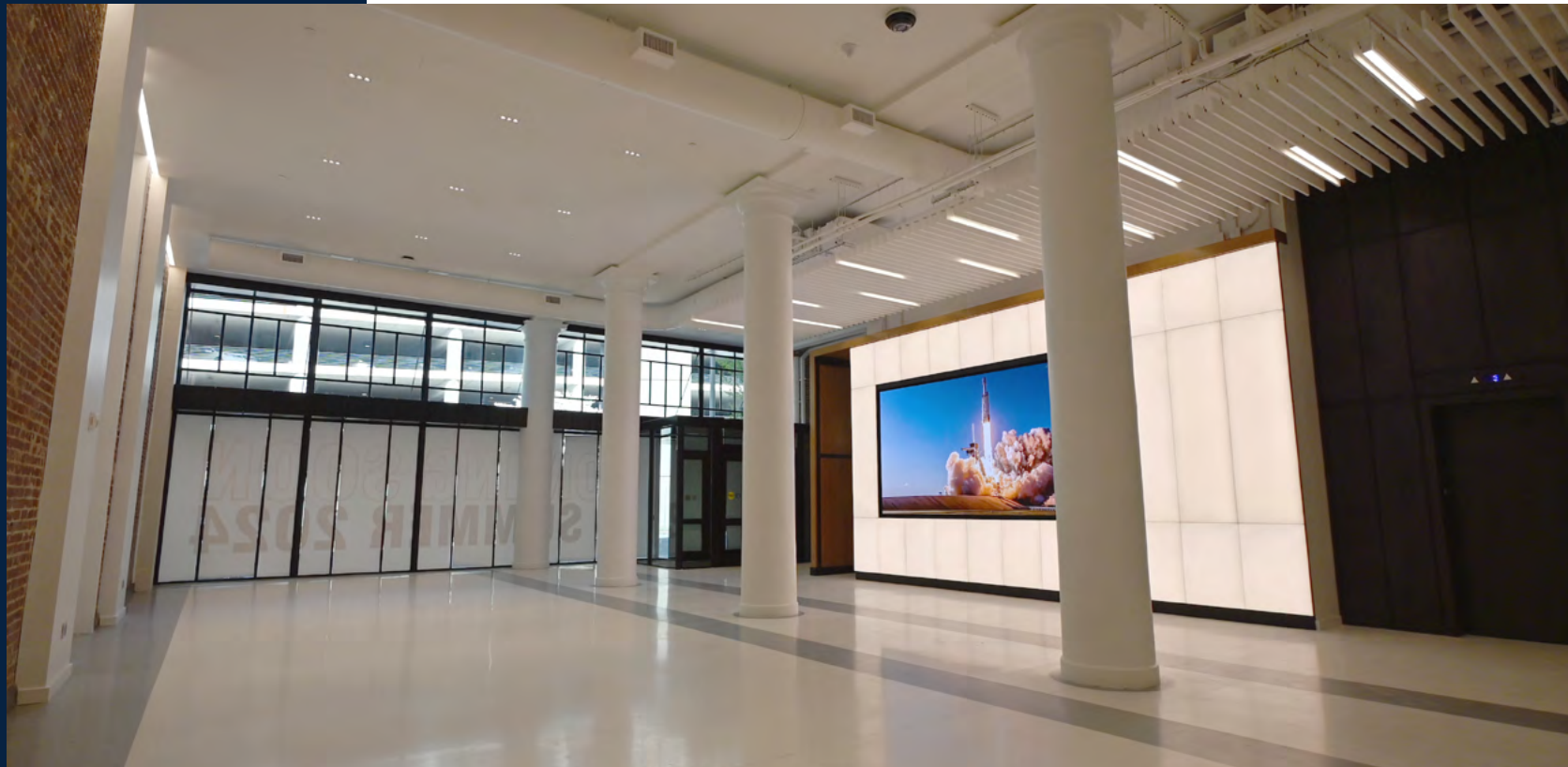
View of finished first-floor lobby with audio visual wall and back-lit glass panels.
