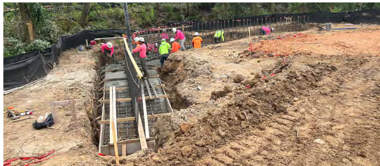
Pouring concrete foundation for the pedestrian bridge.
