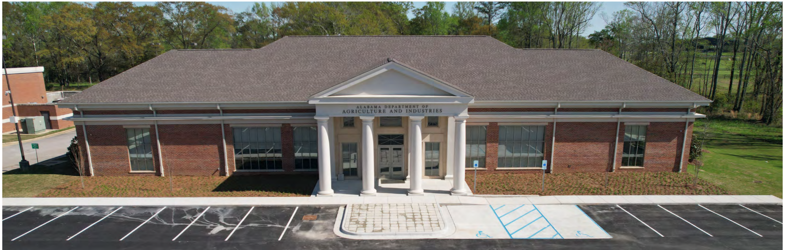
Construction of the State of Alabama Pesticide Residue and Chemical Laboratory is complete.
