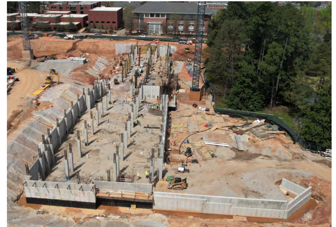
Structural concrete columns are in place to support the first floor of Building C.
