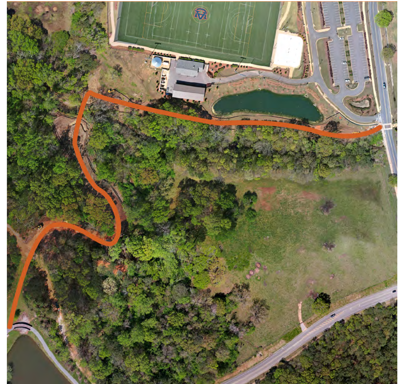
Site grading is currently underway for the new path.
