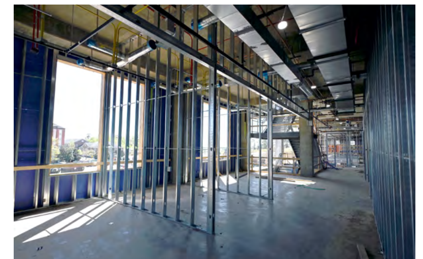
Metal wall framing is in progress for second floor huddle spaces.
