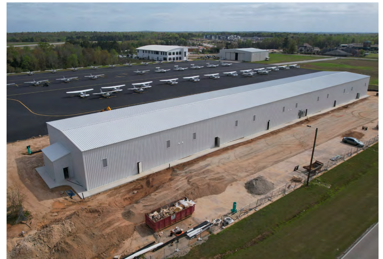
Site work continues outside the hangars.
