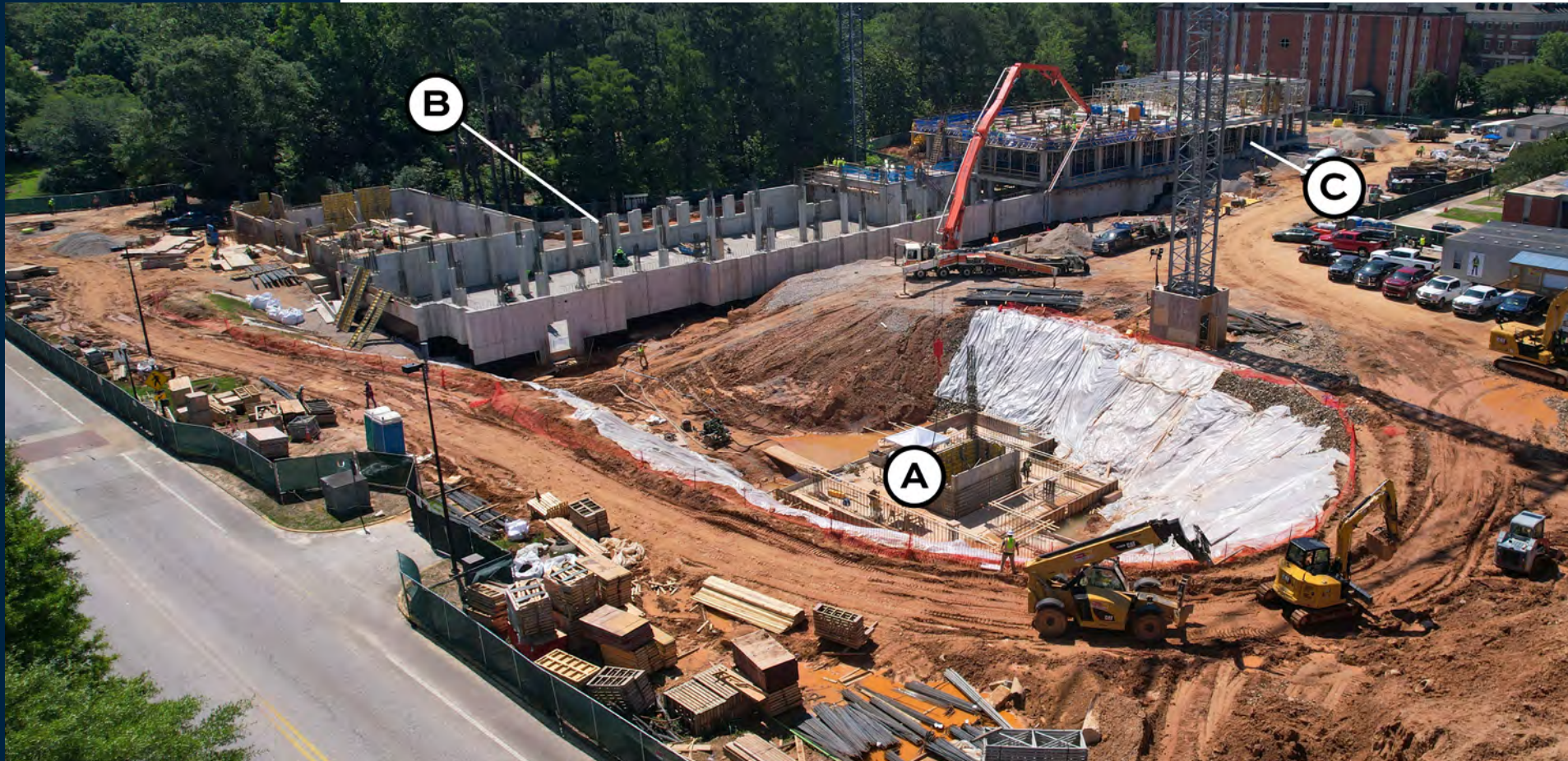
Building A elevator pit and foundation work is underway.
