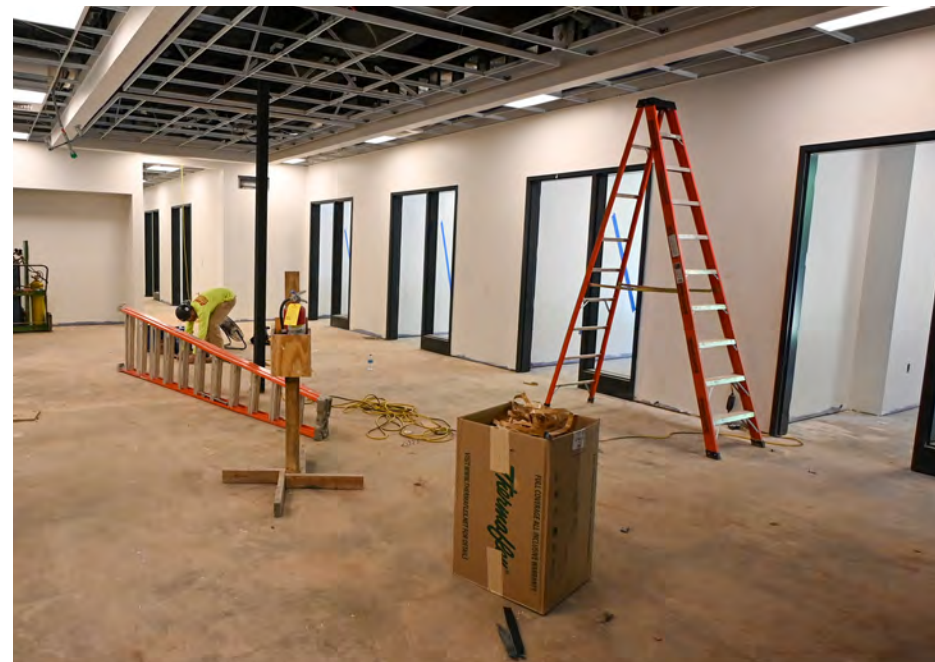
Ceiling mechanical systems near completion in the first-floor office area.
