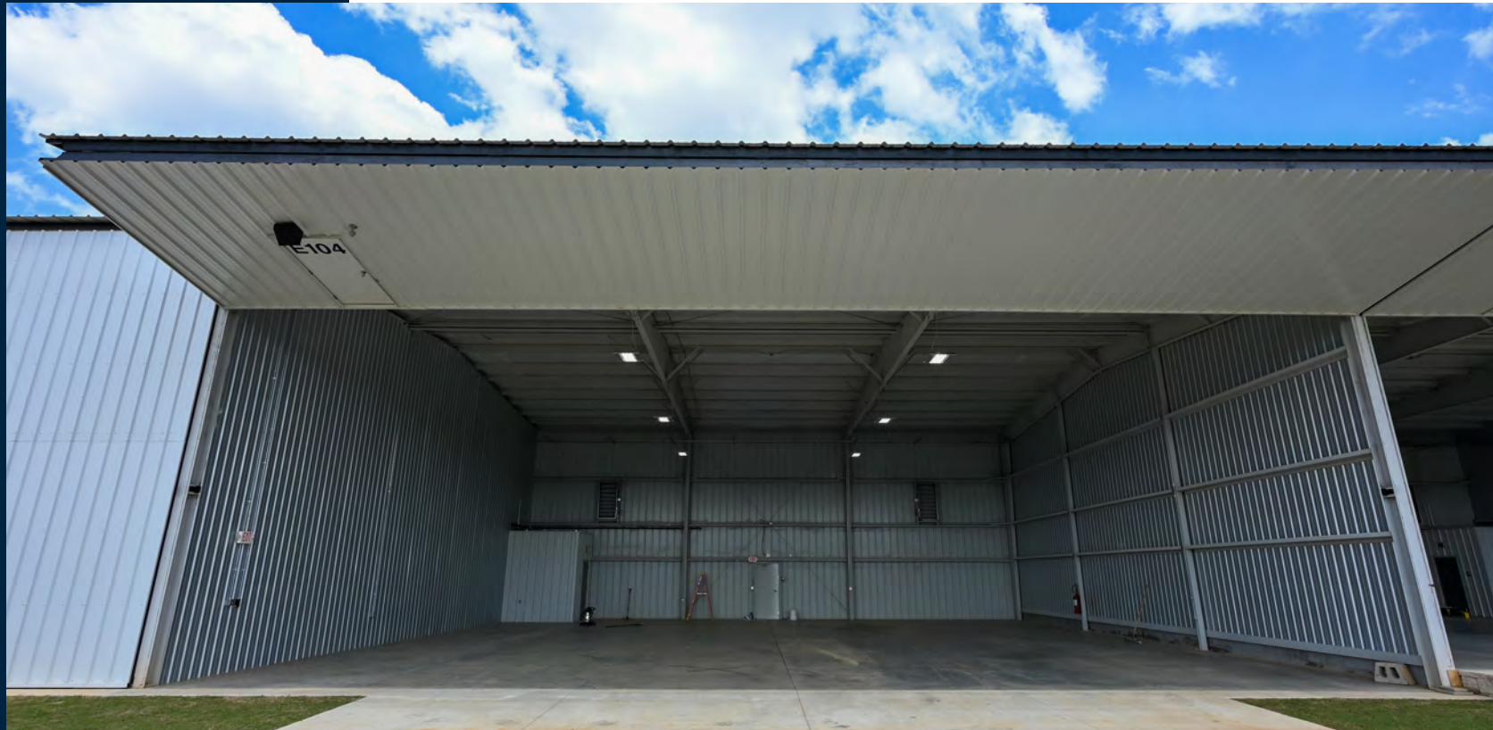
Each individual bay is equipped with a restroom and a motorized bi-folding door.
