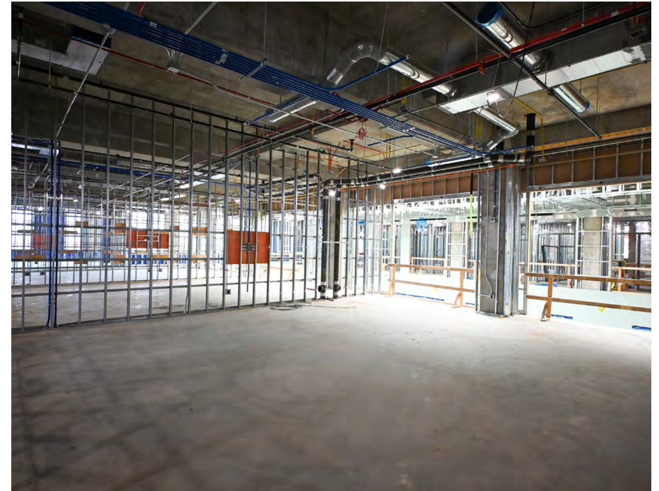
Metal wall framing installation is in progress for the second-floor classrooms.
