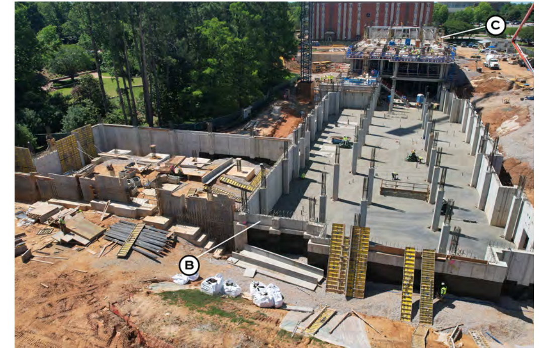
Building B basement concrete foundation, columns and foundation walls are complete.
