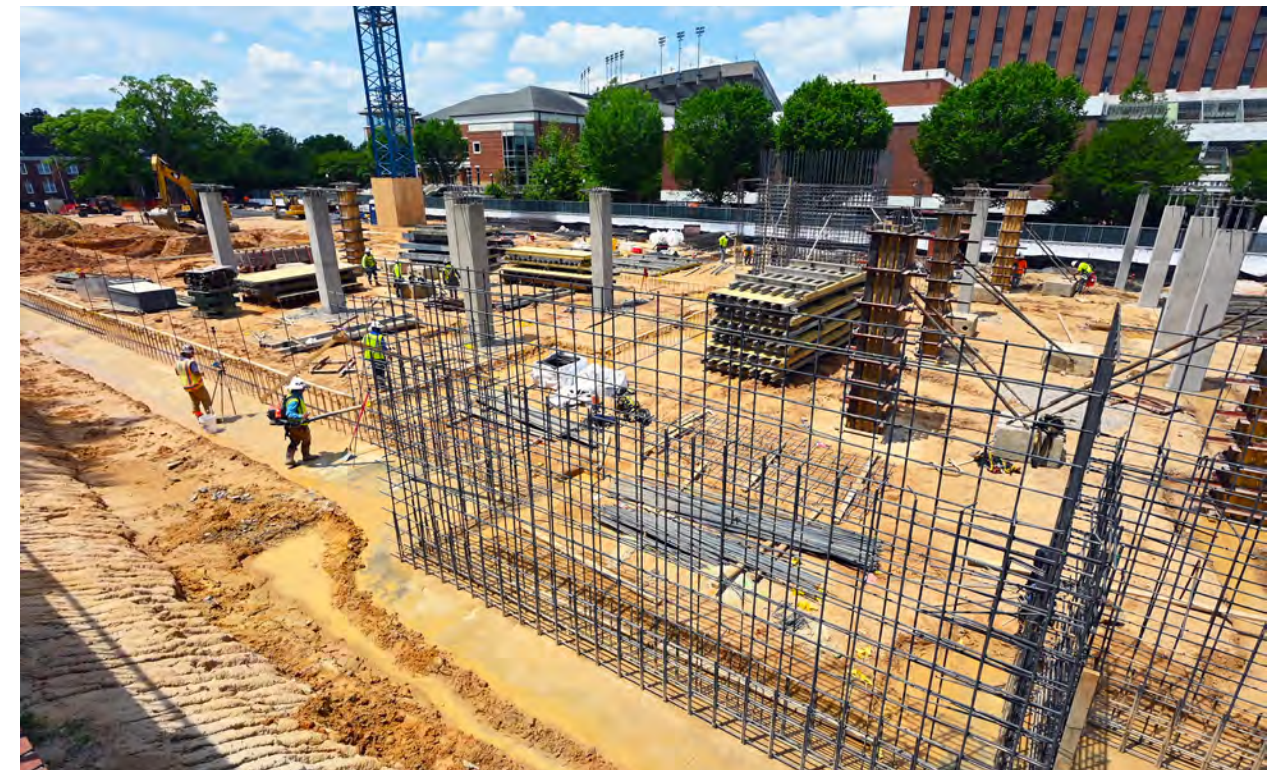
First-floor support columns are being erected at the site.
