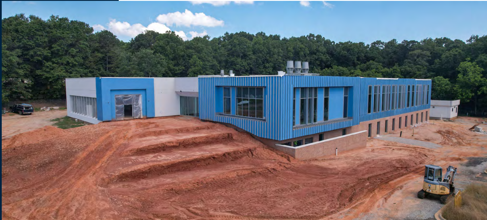
Site grading is underway for the sidewalks and other hardscapes.
