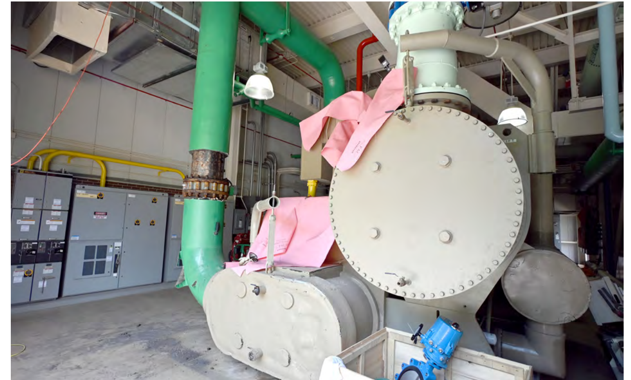
New chillers have been installed while older chillers are being reconfigured.
