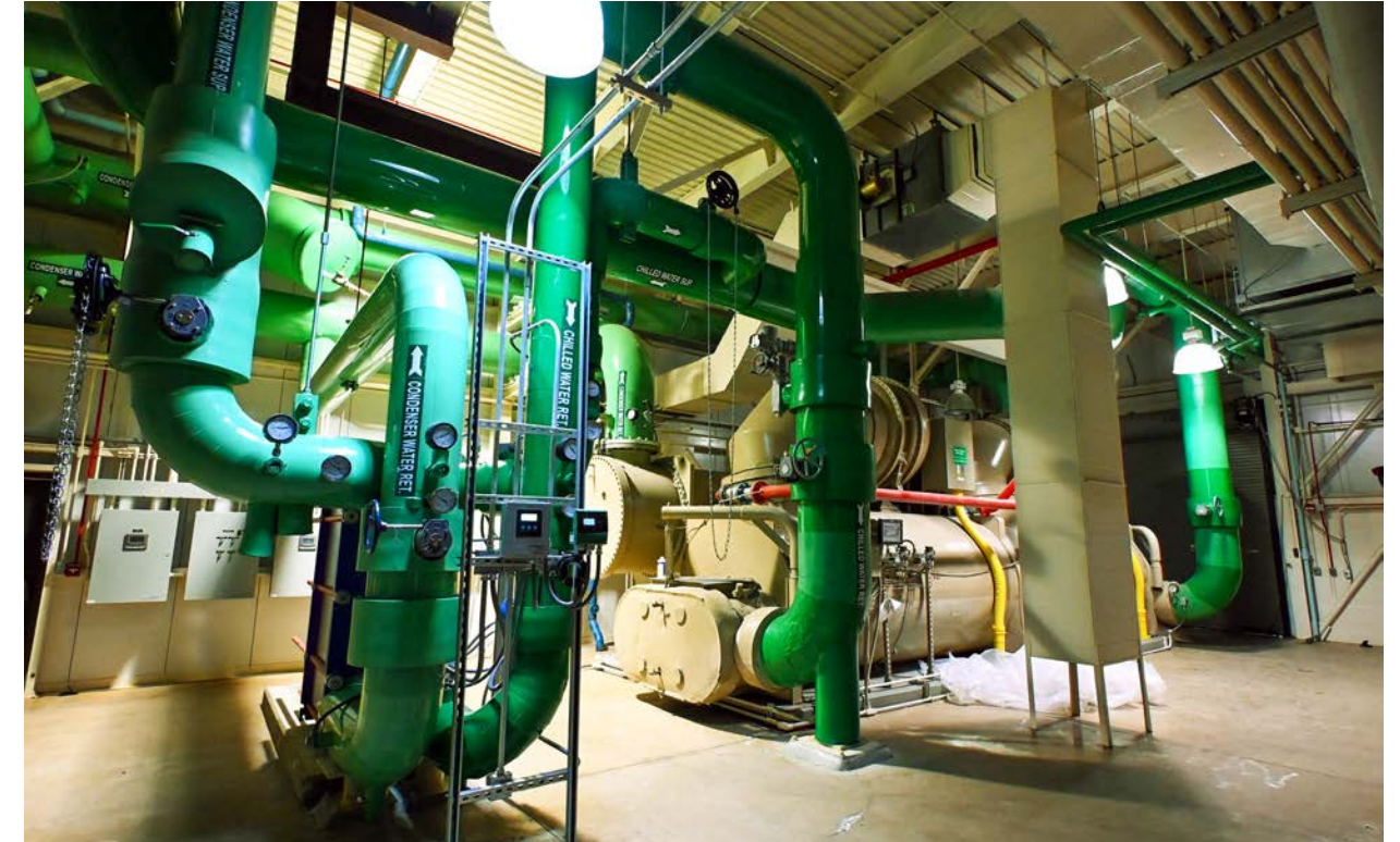
New upgrades in the plant allow for increased water capacity and plant efficiency, allowing the circa 2007 2,500-ton chiller to be saved.
