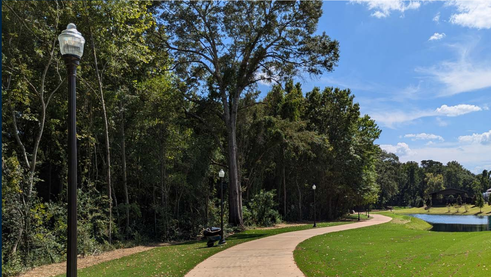
The 12-foot-wide concrete pathway has been completed along the Greenway, connecting Lem Morrison to the VCOM pathway.
