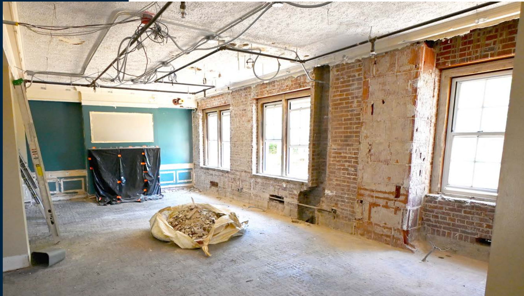
All finishes in the common areas have been fully demolished.
