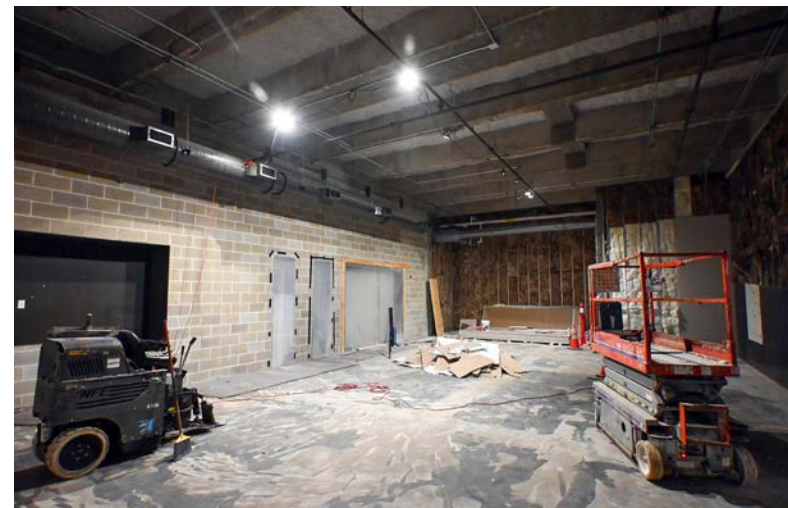
Renovations to the personal training space are underway.
