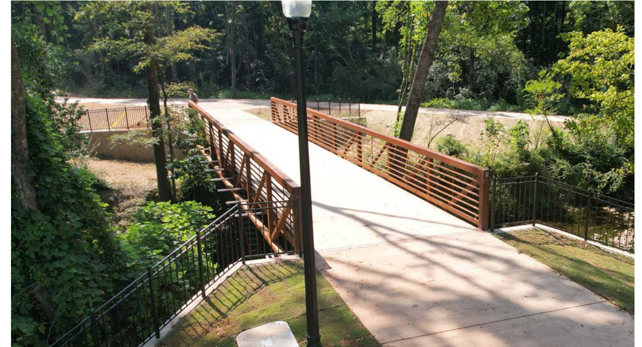
The pre-manufactured truss bridge (span 70-feet) sits across Parkerson Mill Creek, connecting two sections of the Greenway.
