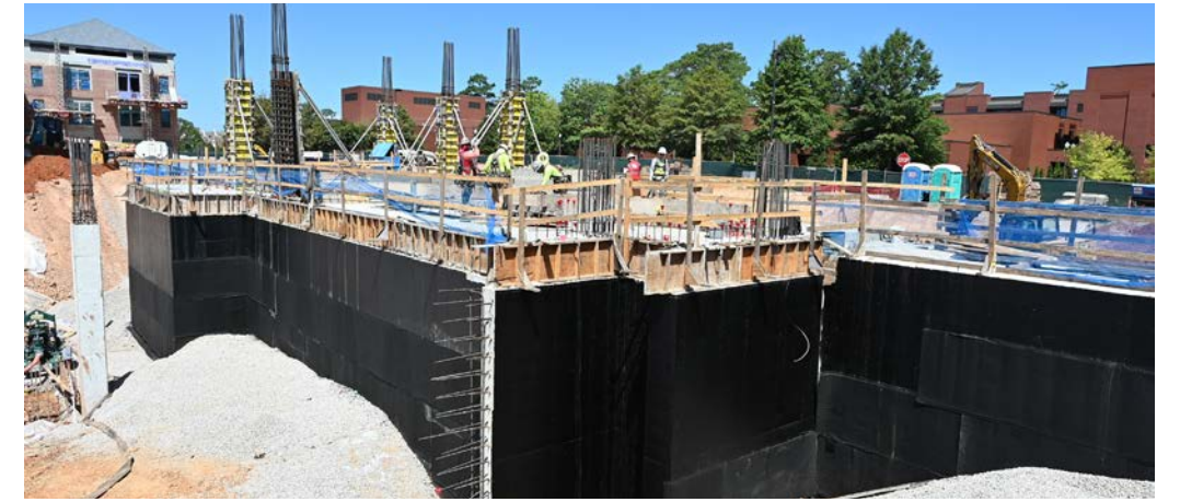
Building A foundation wall waterproofing continues at the basement level.
