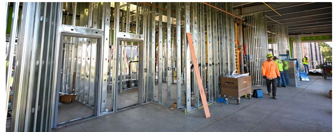
Metal wall framing continues for the new kitchen space.
