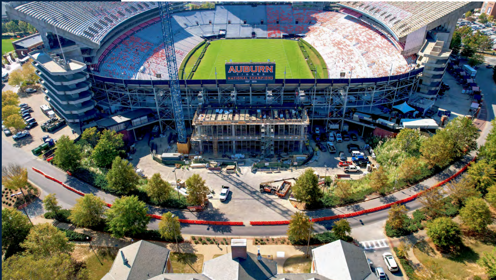
Preparations are underway for level three concrete slab.
