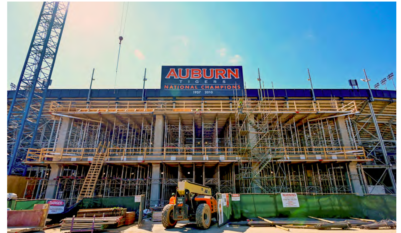
Preparations are underway for level three concrete slab.
