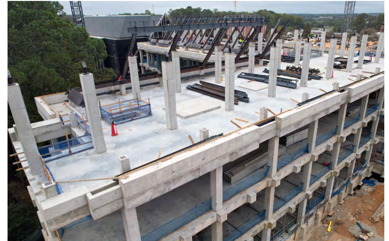
Columns have been formed for the fourth level of Building B.
