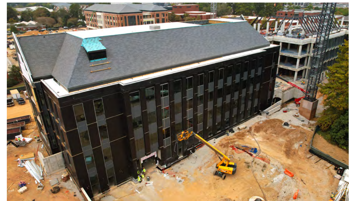
Sheathing and glass are being installed on the outside of Building C as the full structure has taken shape.
