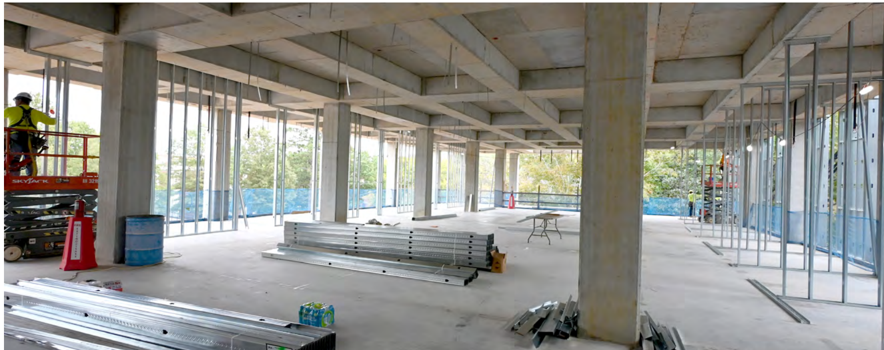
Metal framework currently is being installed on the upper floors of Building B.
