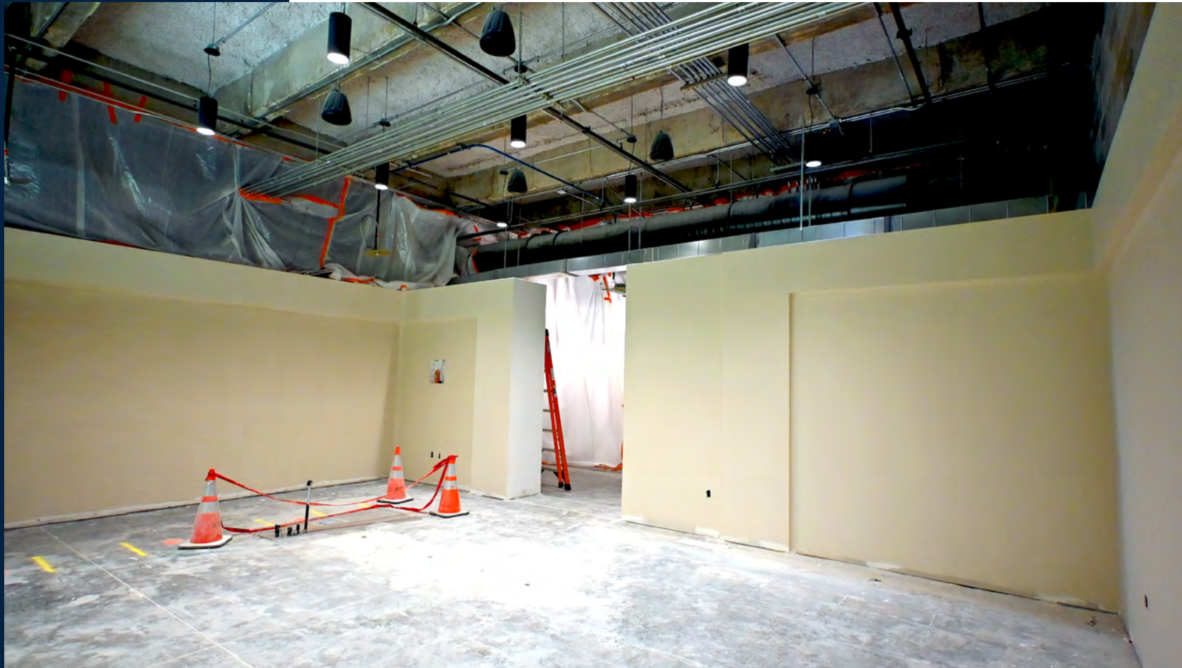
Drywall is complete and the first coat of paint has been applied in the reception area.
