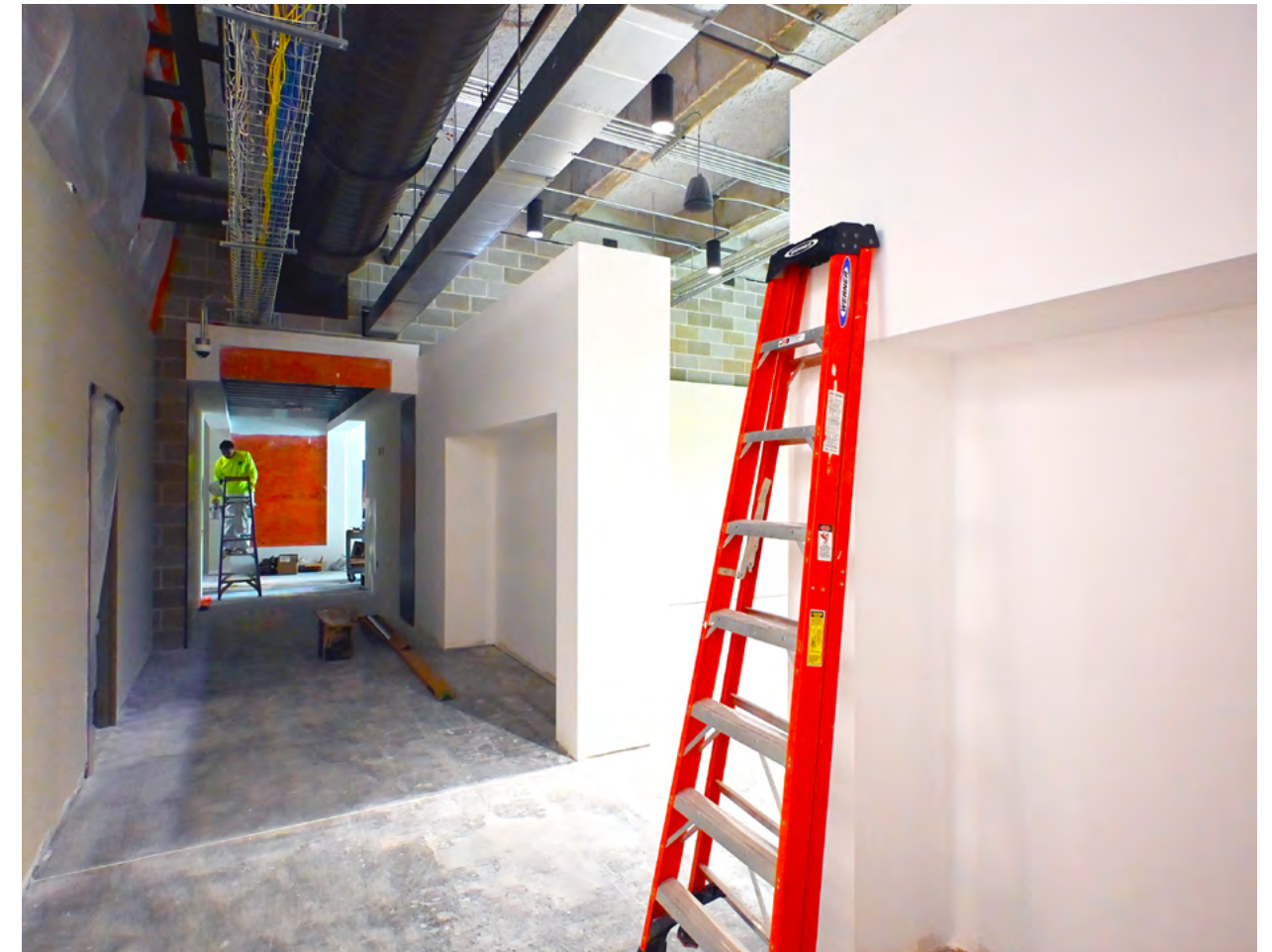
Drywall installation is complete in the hallway leading to the new office spaces.
