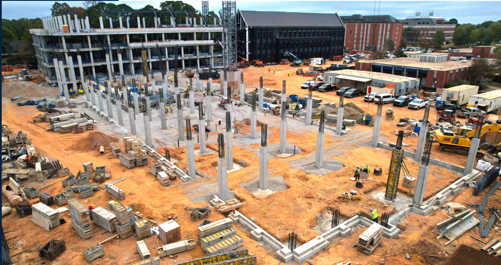
Columns have been formed for the fourth level of Building B.
