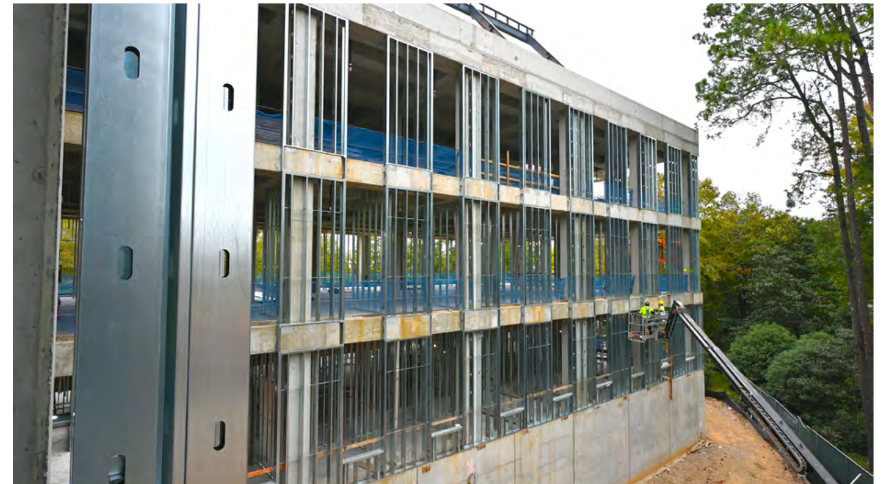
Exterior wall framework is being installed from the ground up outside Building B.
