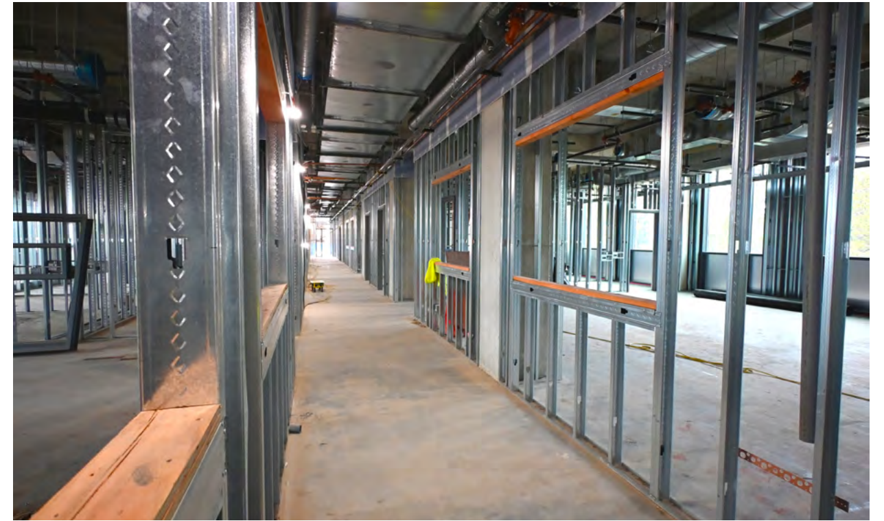
Individual rooms have received their framework on the upper floors of Building C as they prepare for electrical installation.
