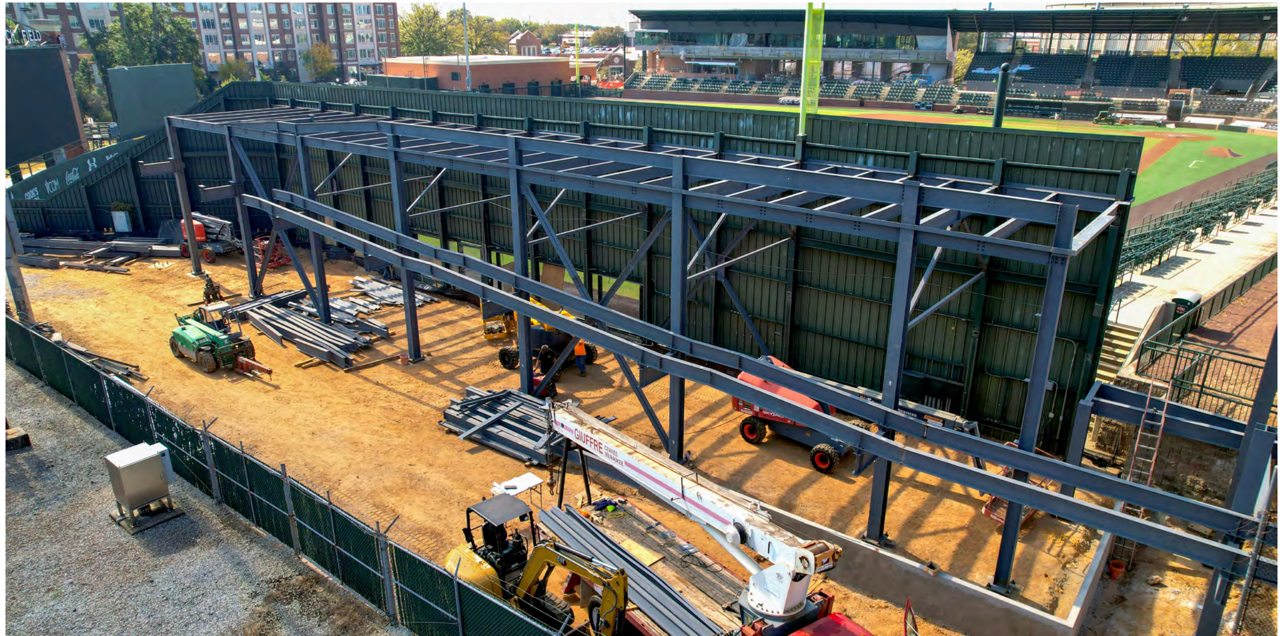
Structural steel installation is taking place for the War Eagle Wall expansion in left field.
