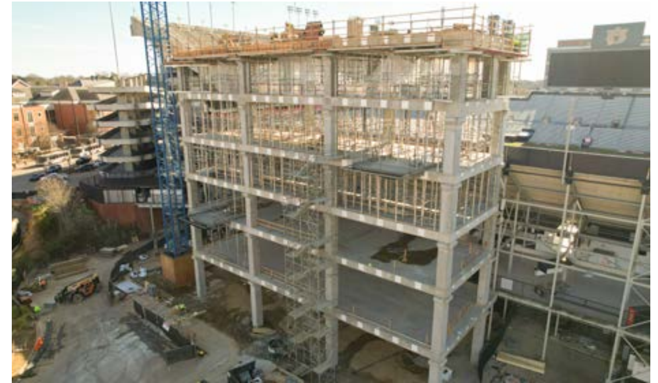
The temporary shorings placed between the concrete floors are being removed after the concrete has cured.
