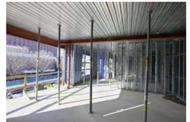
Metal wall framing has begun on the third floor.
