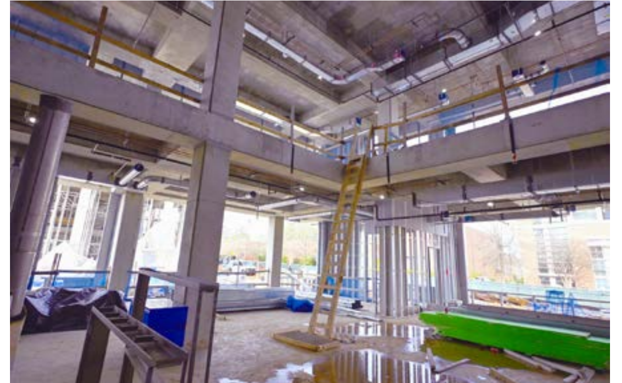
Mechanical, electrical and plumbing is being installed overhead in the entrance.
