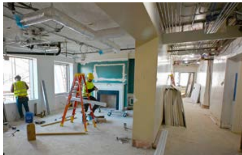
Drywall installation nears completion in Teague Hall.
