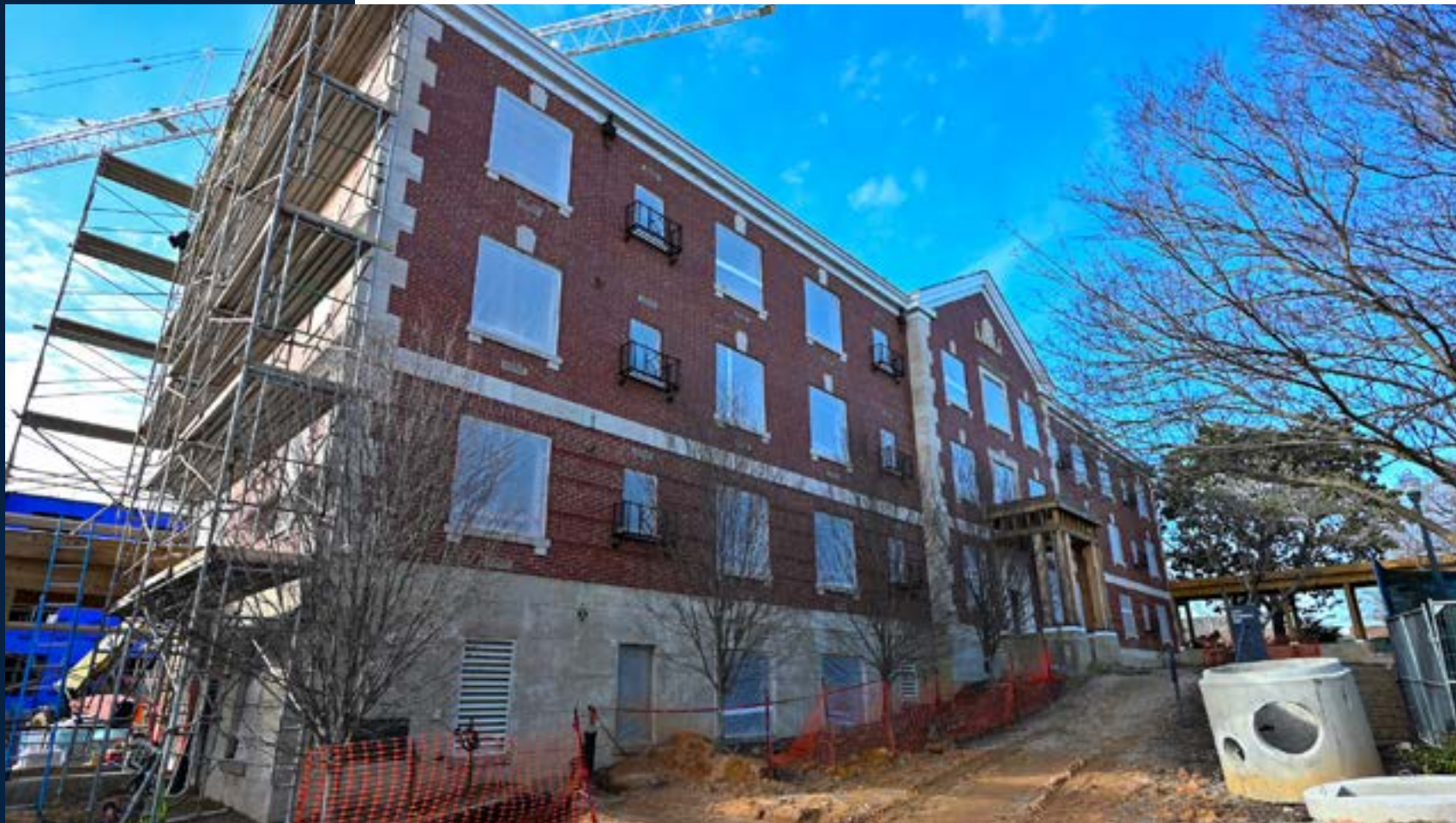
Brick repointing has begun on the south side of Little Hall.
