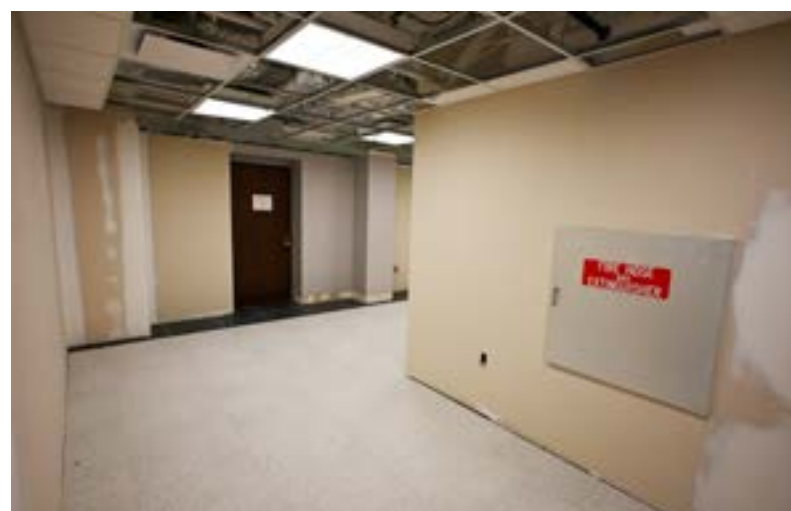
Installation of flooring tile was recently completed in this corridor.
