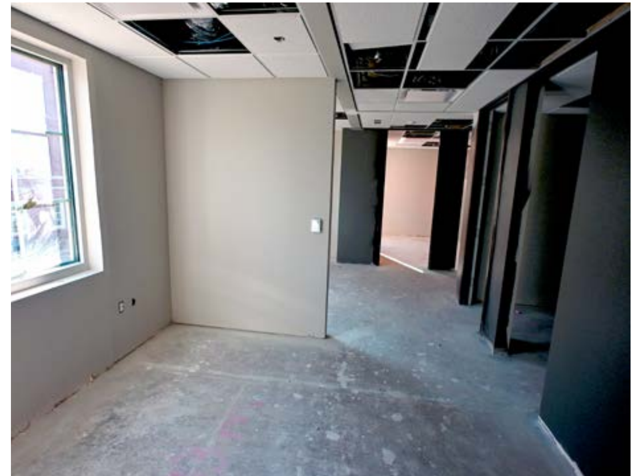
The main hallway has been painted and is awaiting ceiling inspection.
