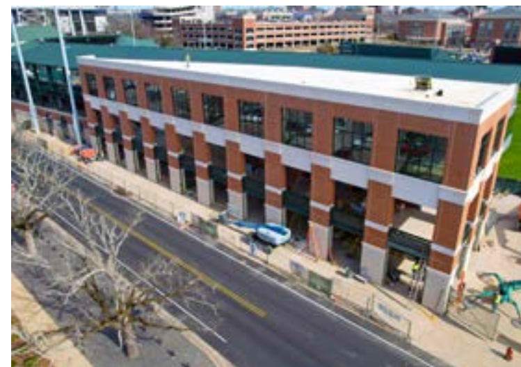
An aerial view of the three-story extension along South Donahue Drive.
