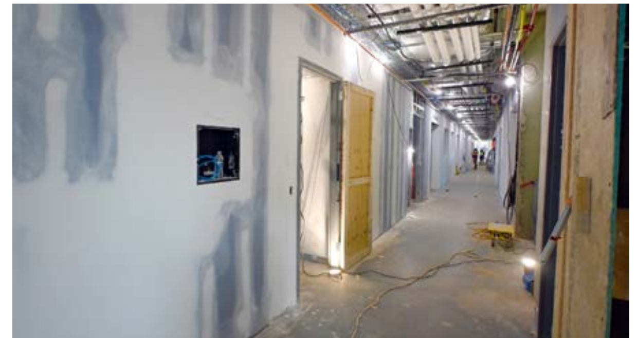
Walls are being readied for paint in this hallway.
